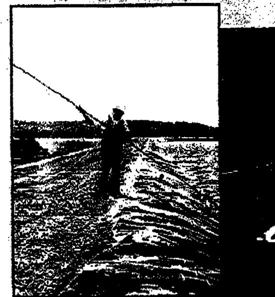
Surveys of side slopes are conducted using sensor probes with long handles.
