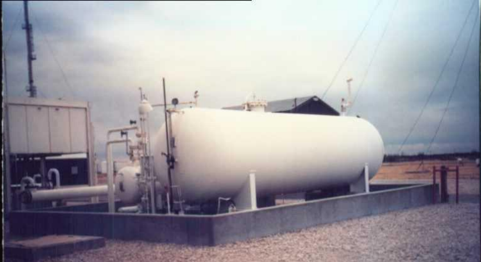
COOPER Engine oil STORAGE AREA #5
