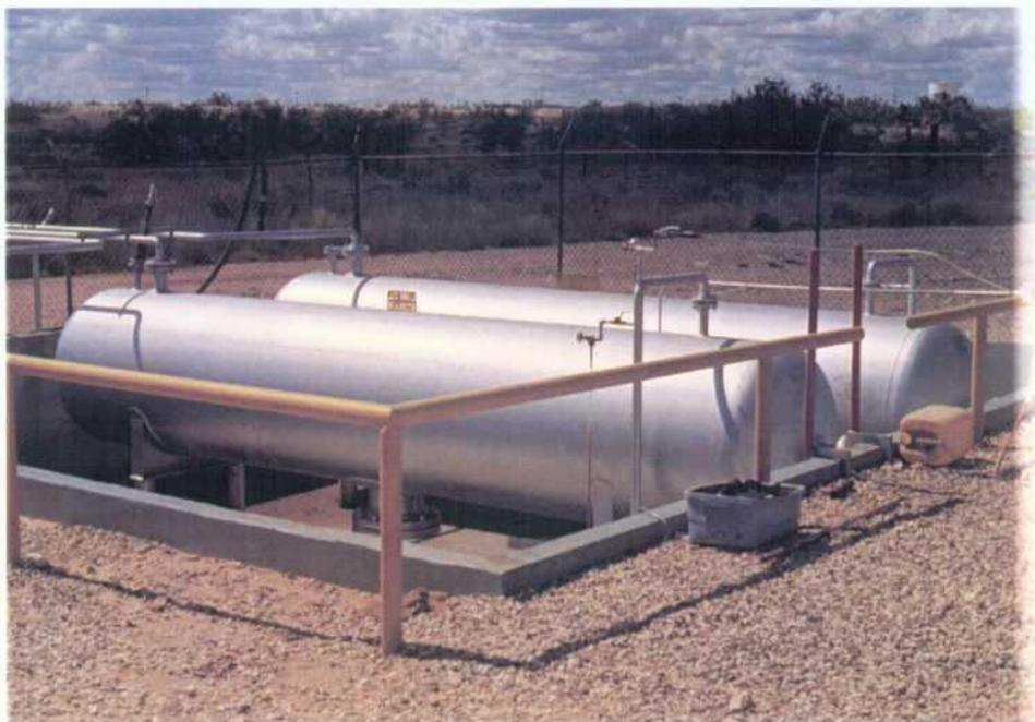
**Figure 2 –Lube Oil (left) and Antifreeze Tanks**
