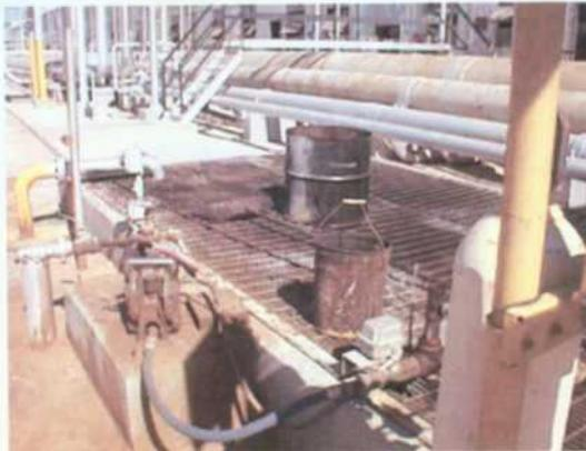
Pic#4 Main Compressor Sump located south of Compressor bldg. Has secondary containment.
