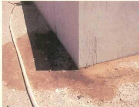
Pic#18 - West Side oil/water tanks - secondary containment leaking.
