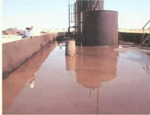
Pic#17 West Side oil/water tanks - recent tank overflow.
