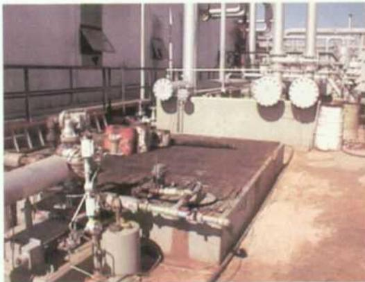
Pic#5 Main compressor Sump north side. Has secondary containment.
