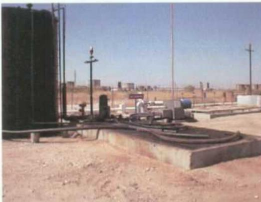
Pic#6 Main Plant oil water separator located on south side of plant area. System has secondary containment.
