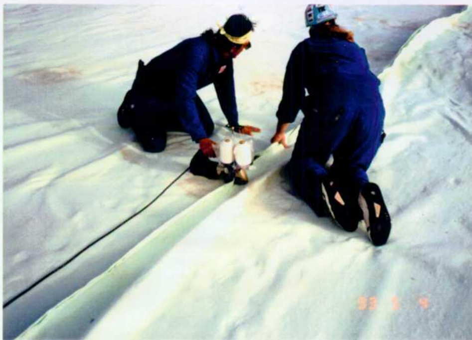
Plate 1 - Stitching Subgrade Geotextile
