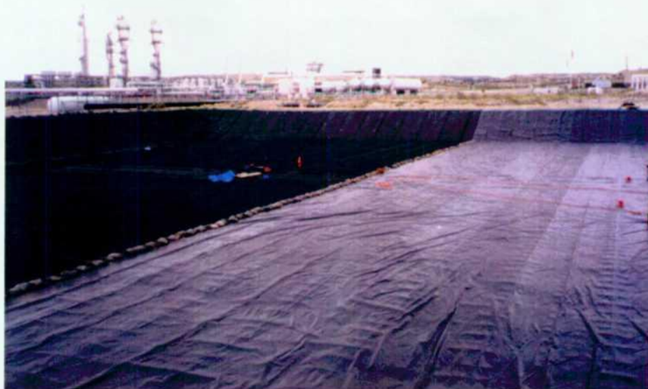
Plate 2 - Net Installation
