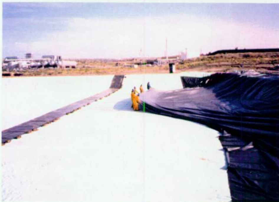
Plate 2 - Opening and Spreading Panel 2
