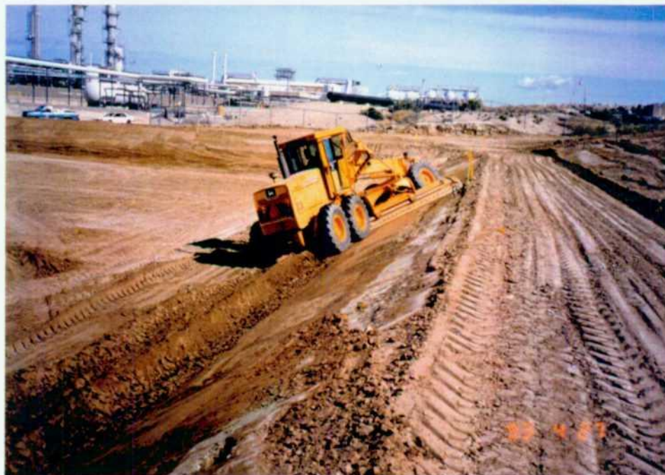
Plate 2 - Pond 1 Slope Grading
