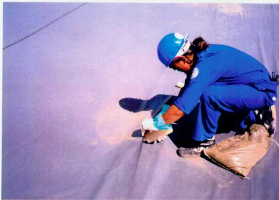
Plate 2 - Pond Liner Seaming
