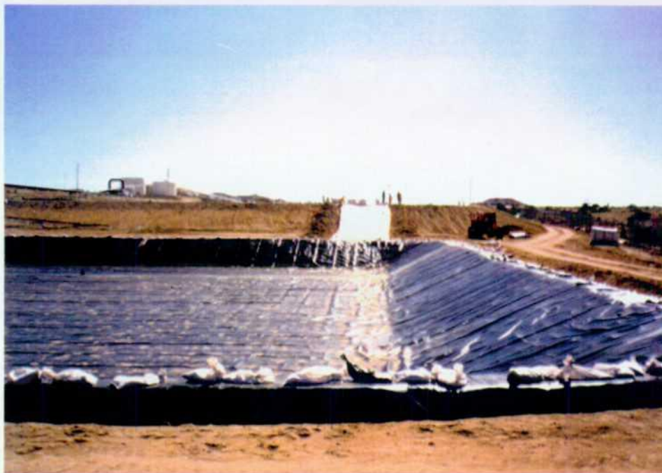
Plate 1 - Pond 1 (Secondary Lining of Overflow)
