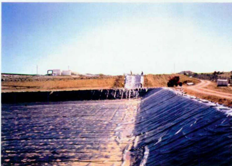
Plate 2 - Pond 1 (Primary Lining of Overflow)
