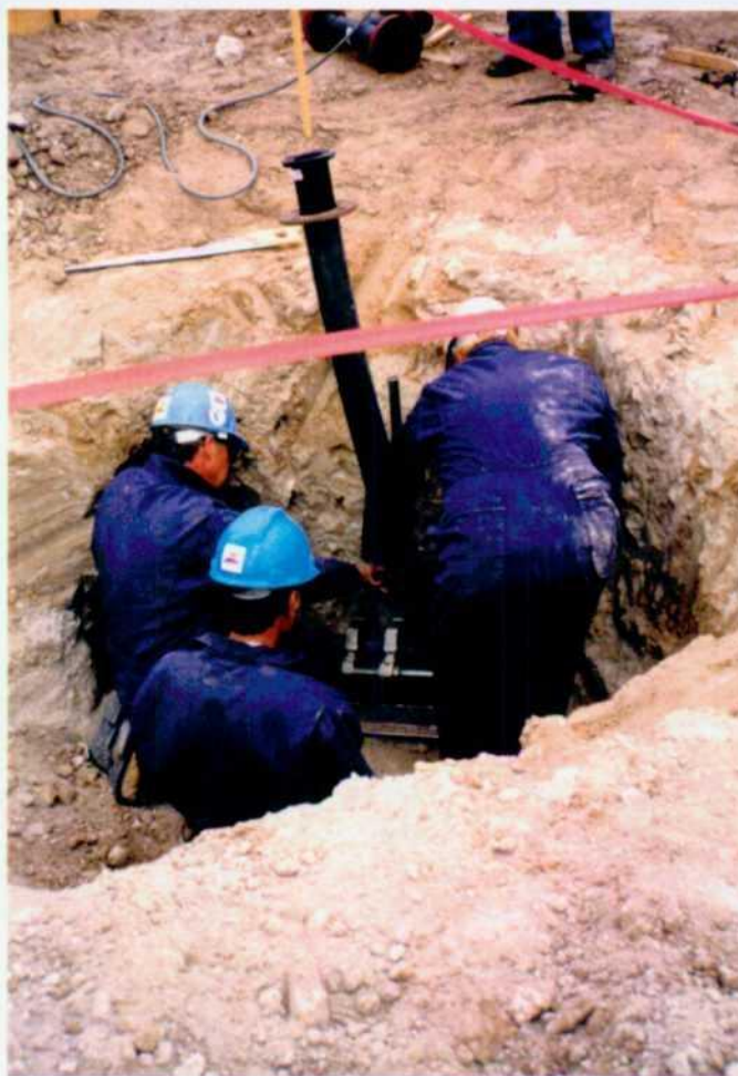
Plate 6 - Wastewater Stub End
