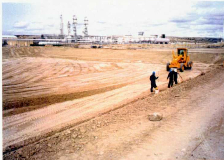
Plate 6 - Pond 2 Grading
