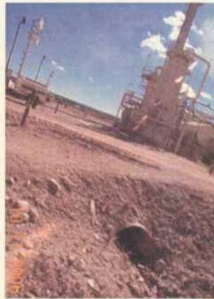
Looking south back toward SE area of process unit where overflow drained through storm water culvert to pond in berm area at NE region of process area.
