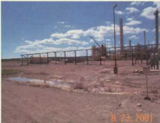
Pic #2- water discharge to ground. Area located NE of plant gas concentration unit. PH of water was measured at 7
