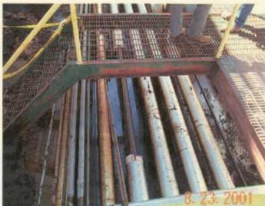
Pic #8- Pipe Rack between Tank # 703 & 706 area free oil on ground.
