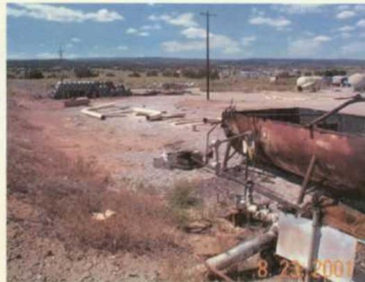
Pic #4- Below-Grade Tank (BGT) old fuel oil unloading catch tank with steam trap.
