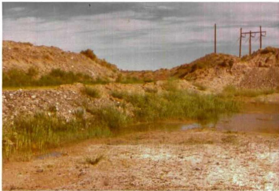
Figure 10. View to the west immediately north of solar evaporation pond #1 showing leakage from the Hammond ditch. The ditch runs from left to right through the photograph but is hidden by the spoil pile on its right bank. Note the cobble in the spoil pile.
