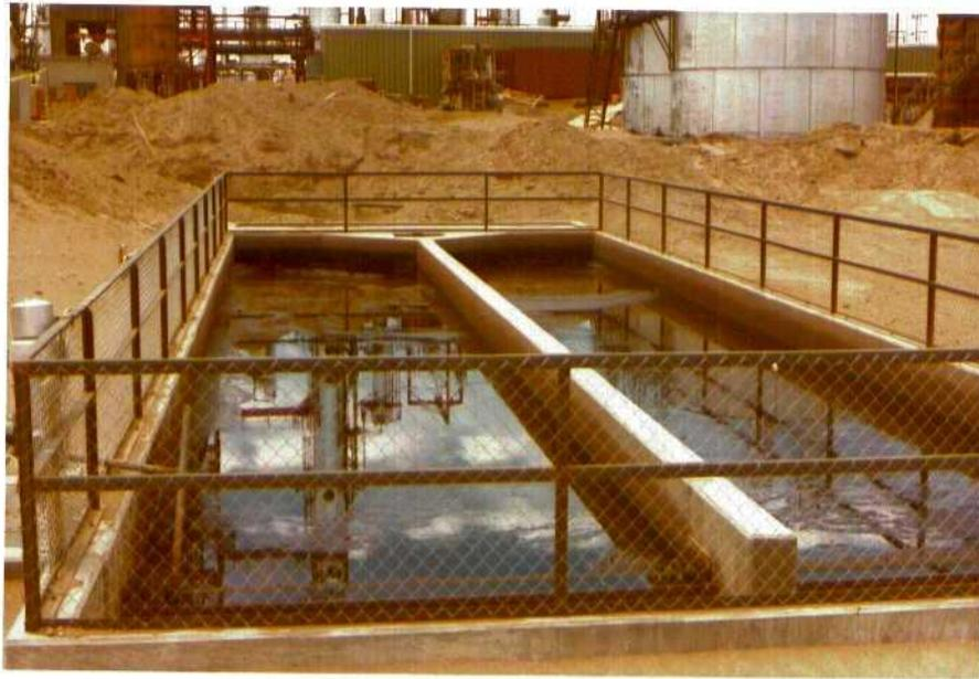
Figure 16. API separator at the Plateau refinery.
