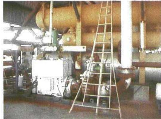
Rankine cycle pentane gas-liquid turbine and induction generator.
