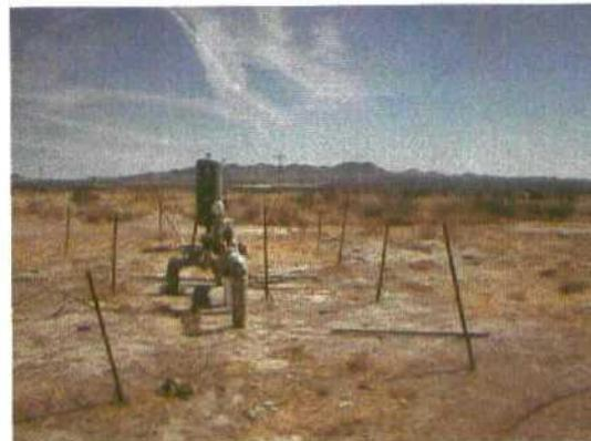
Burgett fresh water well located 10,000 feet west of facility. TDS 300 mg/l. depth of water is 60 feet BGS.
