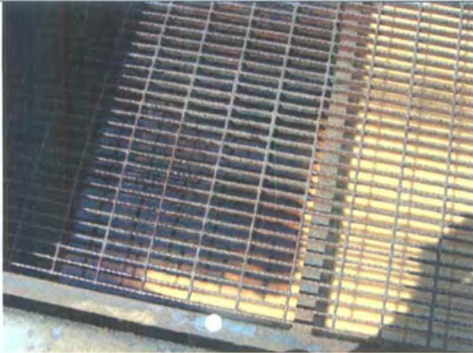
Photo 25: Filter drain area.
