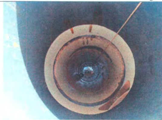
Photo 4: 2 produced water pond leak detection system with fluids.
