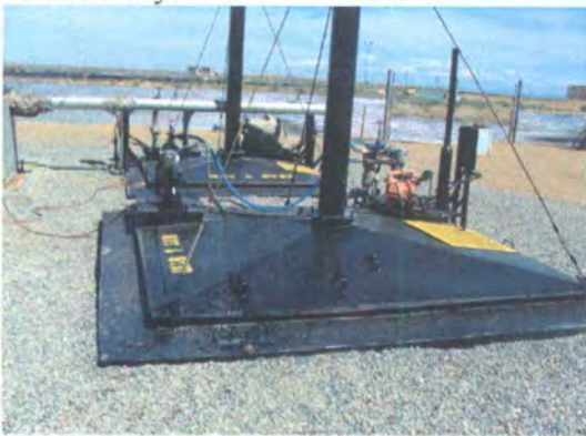
Photo 21: 2 of 3 BGT, leak detection verified dry.
