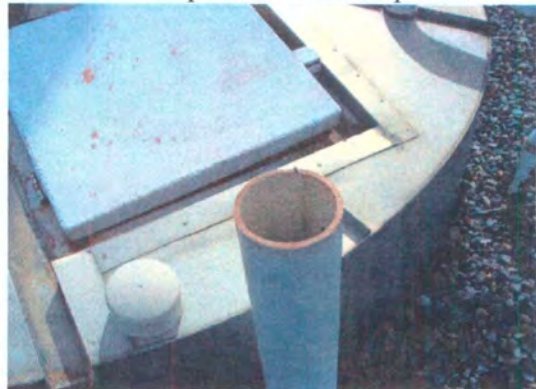
Photo 6: Leak detection of BGT, verified dry.
