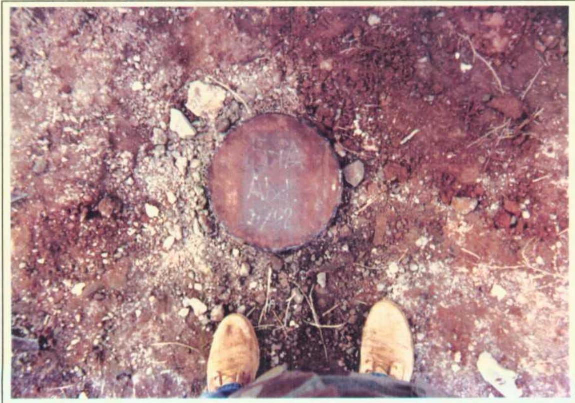
*Steel abandonment cap welded to surface casing*
