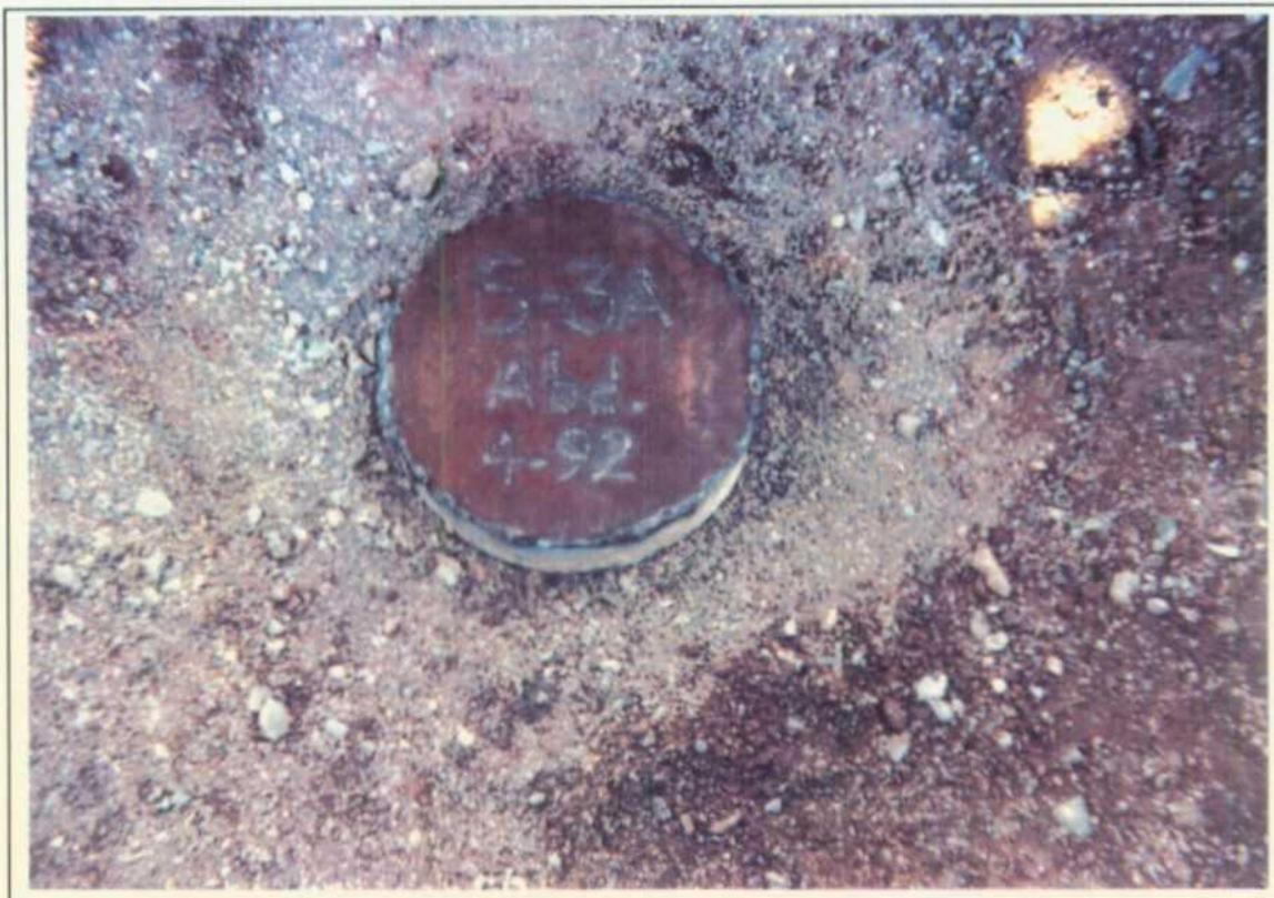
*Steel abandonment cap welded to surface casing*
