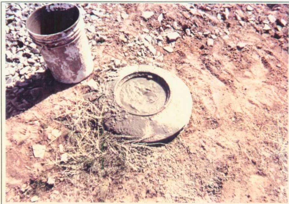
*Monitor well 5-27B cement grout level at surface, prior to welding steel abandonment cap*
