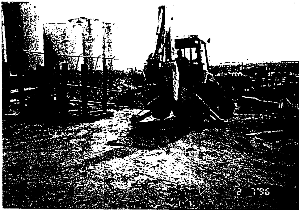
VIEW OF TEST PIT EXCAVATION ACTIVITIES LOOKING SOUTH
