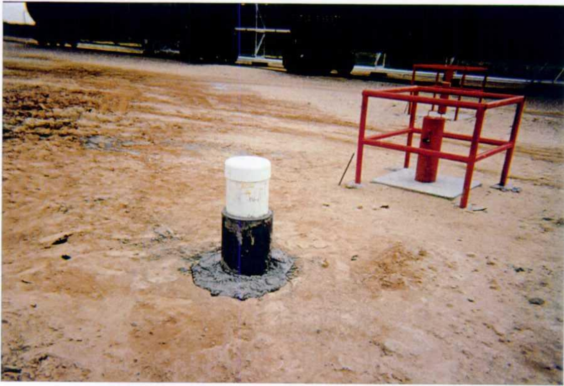
Recovery well RW-1 to be completed after installation of remediation system
