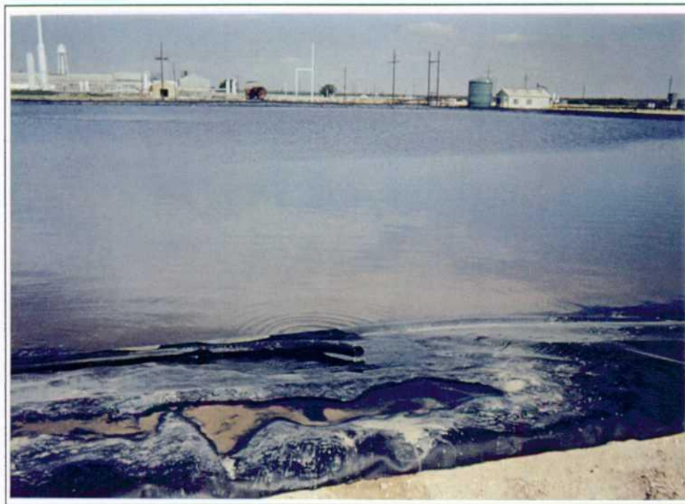
Development water from RW-1 pumped to southern brine pit
