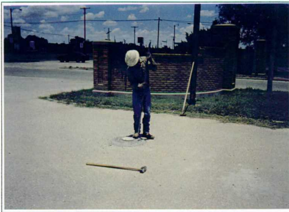
Removal of monitor well in parking lot of Sheriff's Department property
