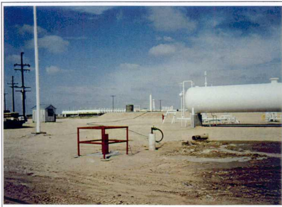
Development of RW-1 with Grundfos Pump
