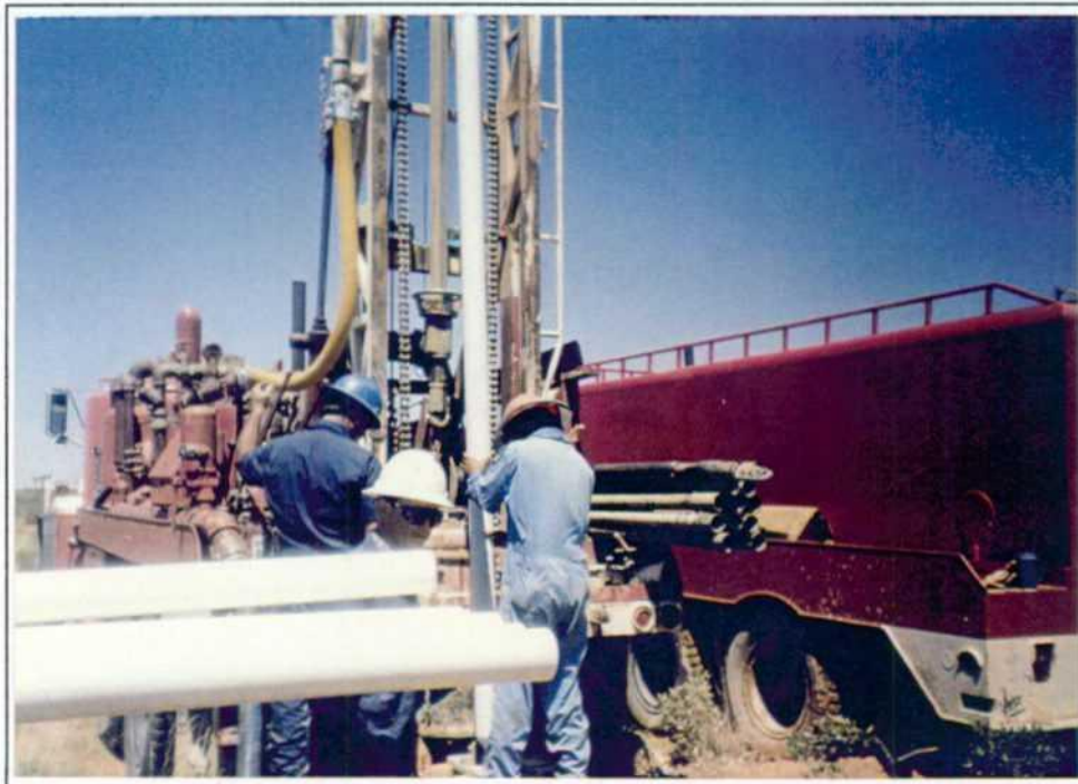
Installation of 4" piping in ACW-13
