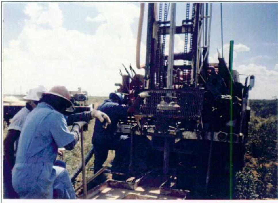
Installation of 4" piping in ACW-14
