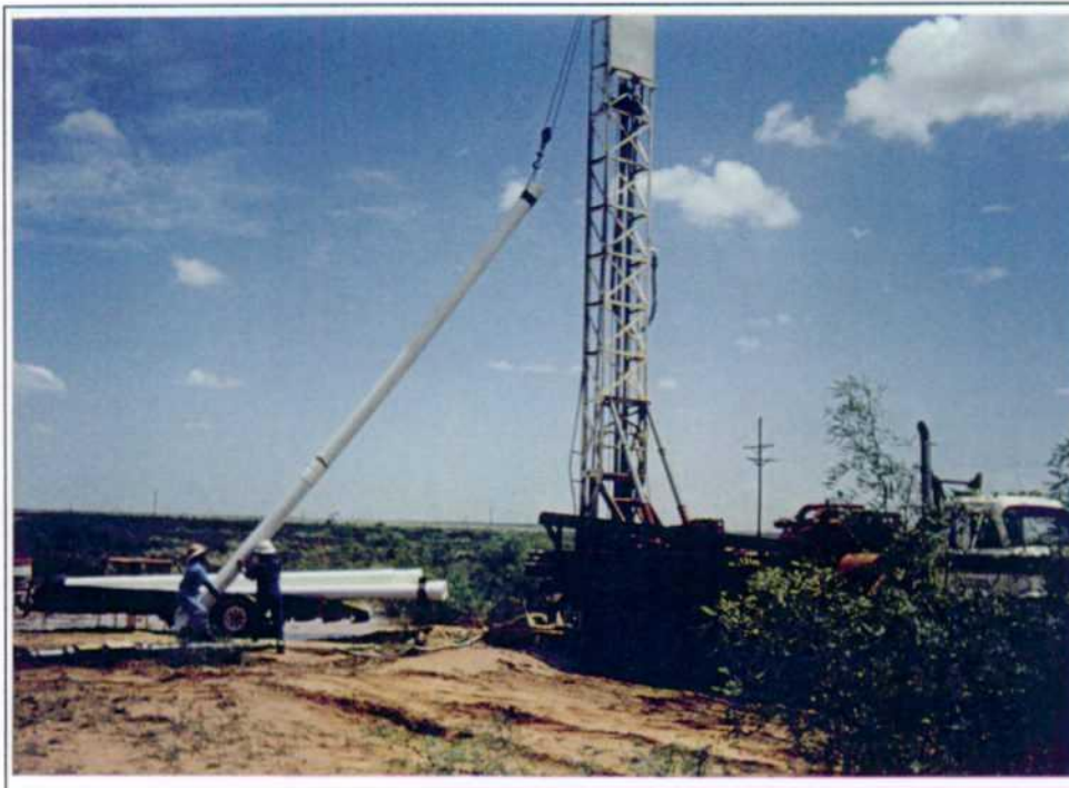
Installation of piping for RW-2
