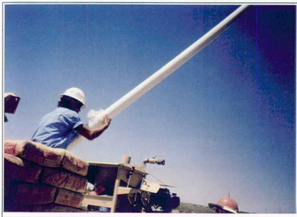
Installation of 4" piping in ACW-12
