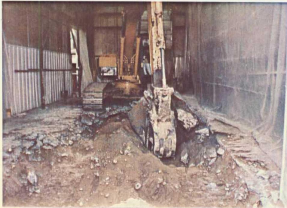
9. Removal of concrete and excavation of soils inside northern margin of HFTO building. Note plastic walls (at left and right) constructed to minimize migration of dust and odors into other portion of the building.
