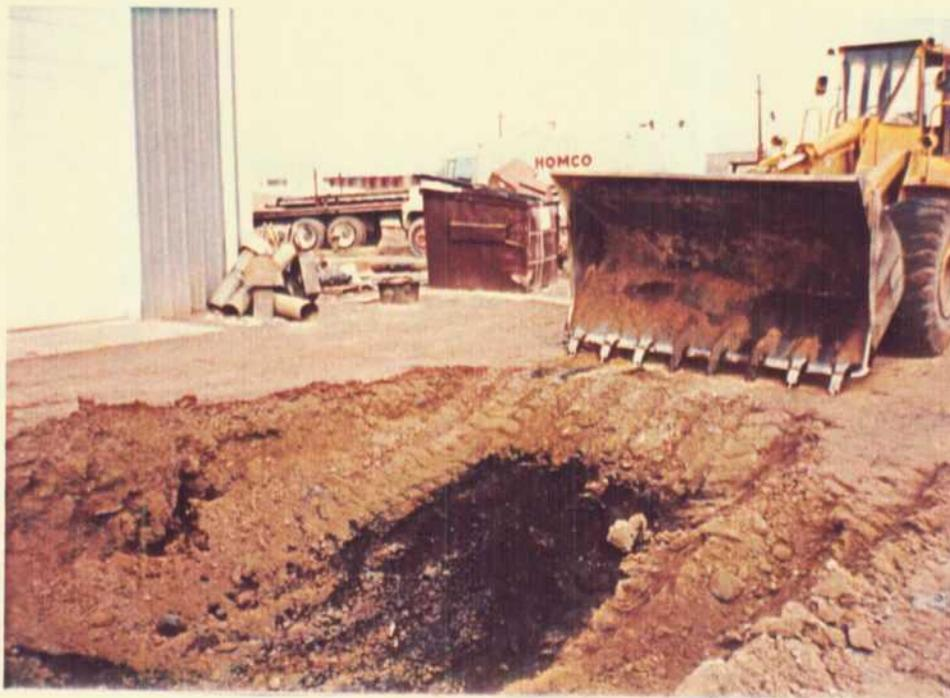
12. Excavation of leach field directly in front of HWS building. Leach field gravels and adjacent soils are saturated with petroleum hydrocarbons. This leach field is the source of contaminants for the bedrock plume.
