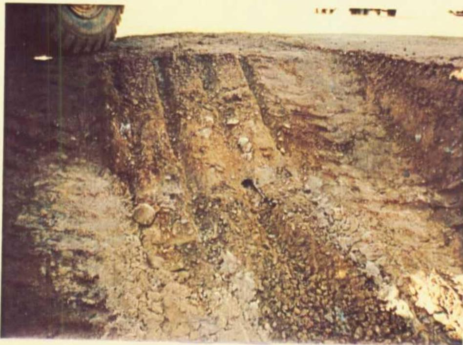
8. Excavation of drain line and leach field that extend to southwest from the HFTO building and past the facility fence. Leach field gravels visible in the foreground do not exhibit extensive hydrocarbon staining. Analytical results of sample collected from these materials exceeded NMOCD action levels; leach field was subsequently removed.
