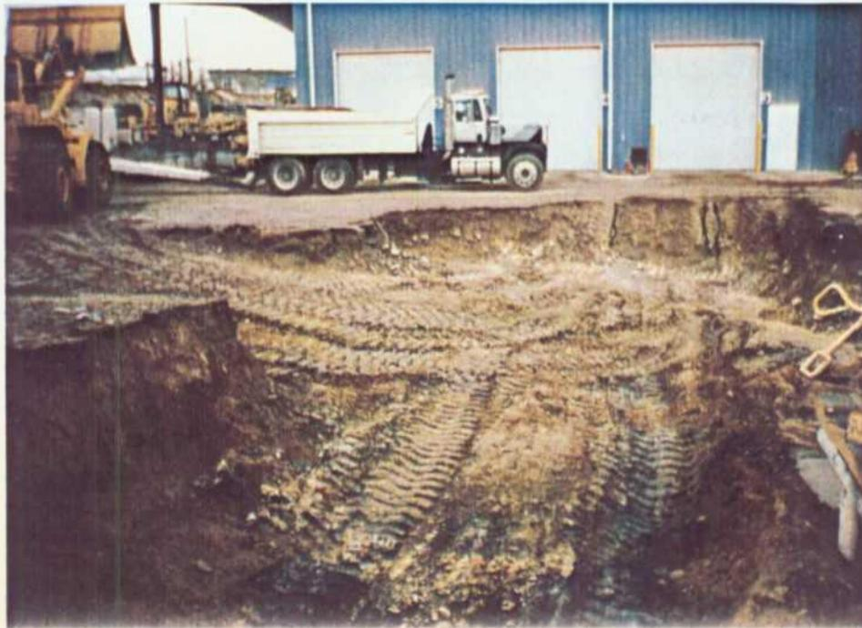
25. View of northeast margin of completed excavation for shallow drain lines and leach fields originating from HWS building.
