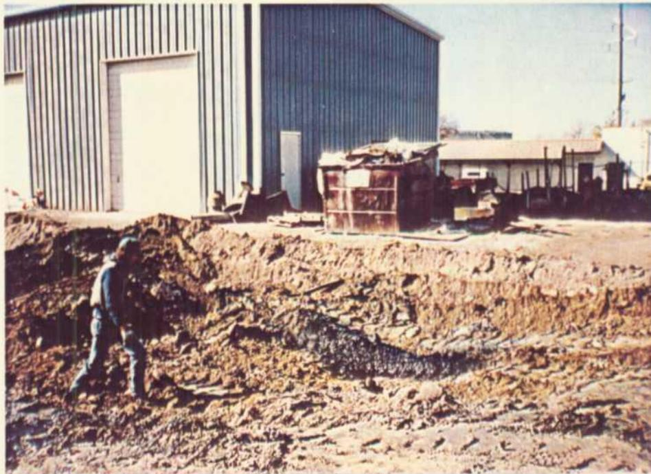
14. Excavation of leach field extending to the north from the front of the HWS building. Leach field gravels and adjacent soils are saturated with petroleum hydrocarbon contaminants.
