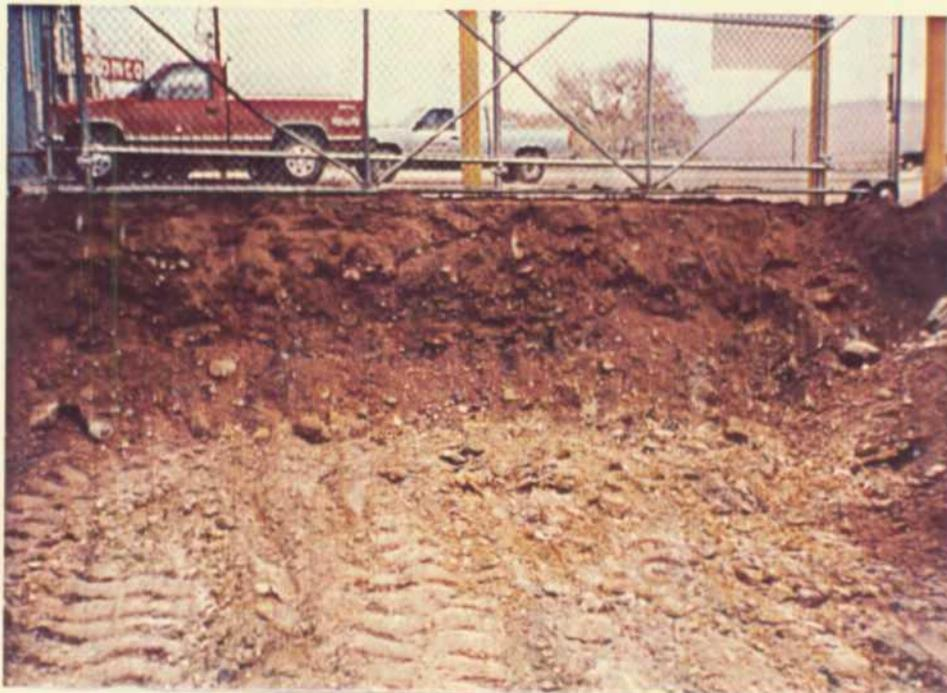
4. View of south wall of excavation adjacent to western margin of HFTO building. Hydrocarbon-stained materials are visible in this sidewall. Excavation was extended to south to remove these stained materials after the fence was dismantled.
