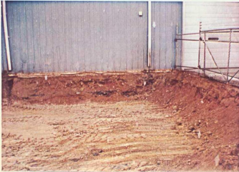
5. View of southeast corner of excavation adjacent to western margin of HFTO building. Petroleum hydrocarbon contaminants visible in the east wall occur in soils beneath the building foundation. These contaminants migrated from the indoor sump located on the other side of the wall. The east wall was not excavated any further to avoid damage to the building foundation.
