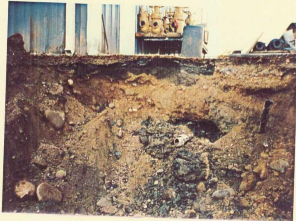
16. View of drain line and leach field that trend in east-west direction along northern margin of HWS building. Surficial soil is stained black from spillage of used oil.
