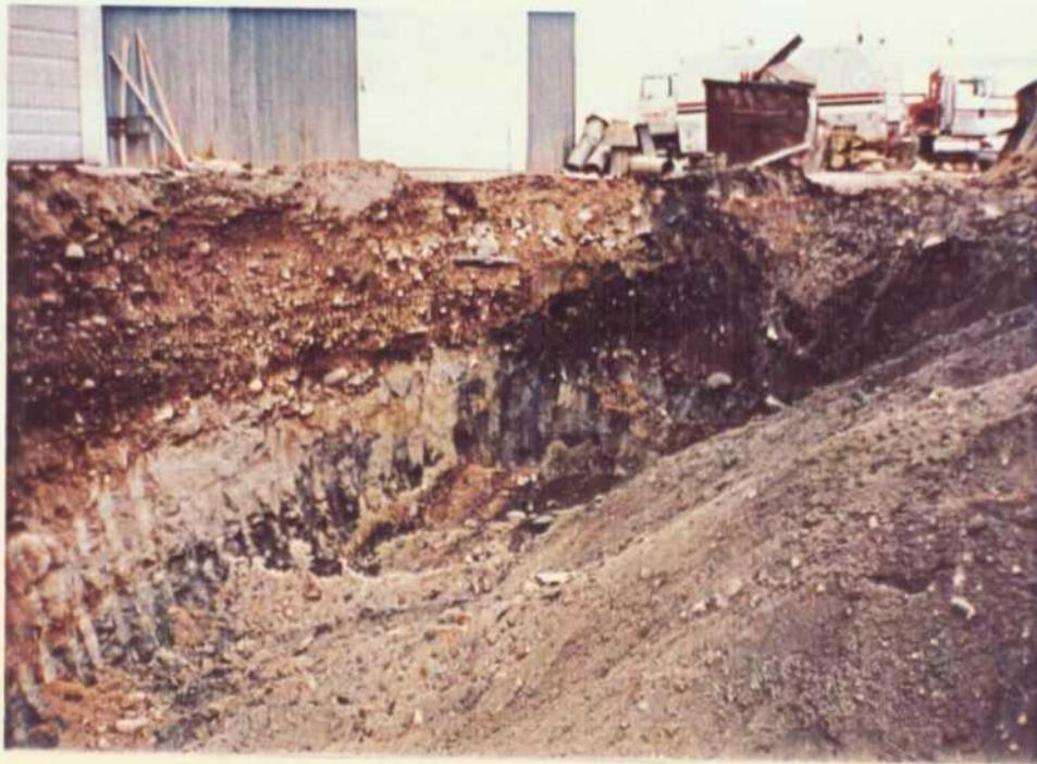
21. View to northwest of excavation for bedrock plume. Overlying leach field was source of petroleum hydrocarbon contaminants for this plume.
