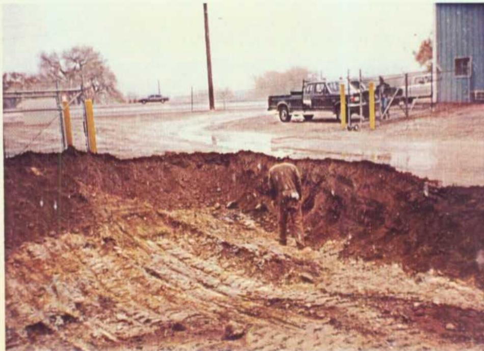
1. View of southwest corner of excavation adjacent to western margin of HFTO building. West wall and southwest corner of this excavation are the furthest extent of the excavation completed in these directions. The total depth of the excavation into the bedrock (light colored material at left in foreground) is also depicted.
