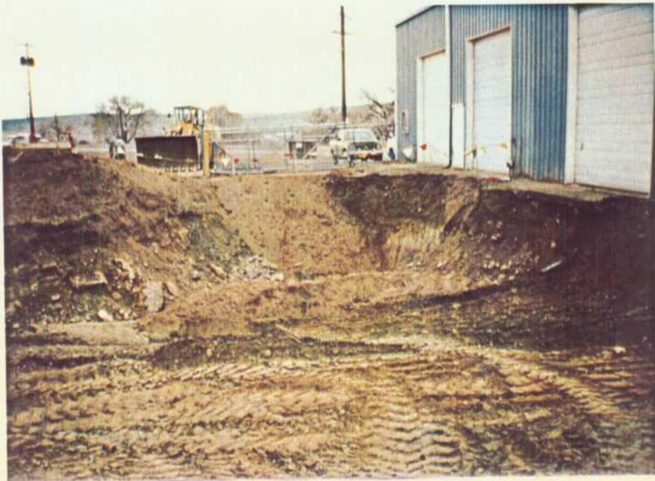
27. View to south of completed excavation for shallow drain lines and leach fields originating from HWS building.
