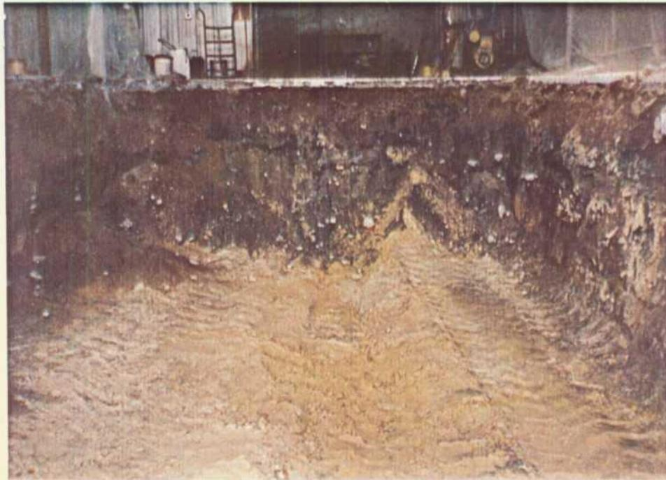
11. Close up view of completed excavation inside northern margin of HFTO building. Note the hydrocarbon stained soils present in the sidewalls, The excavation was not extended further to avoid damage to the building foundation.
