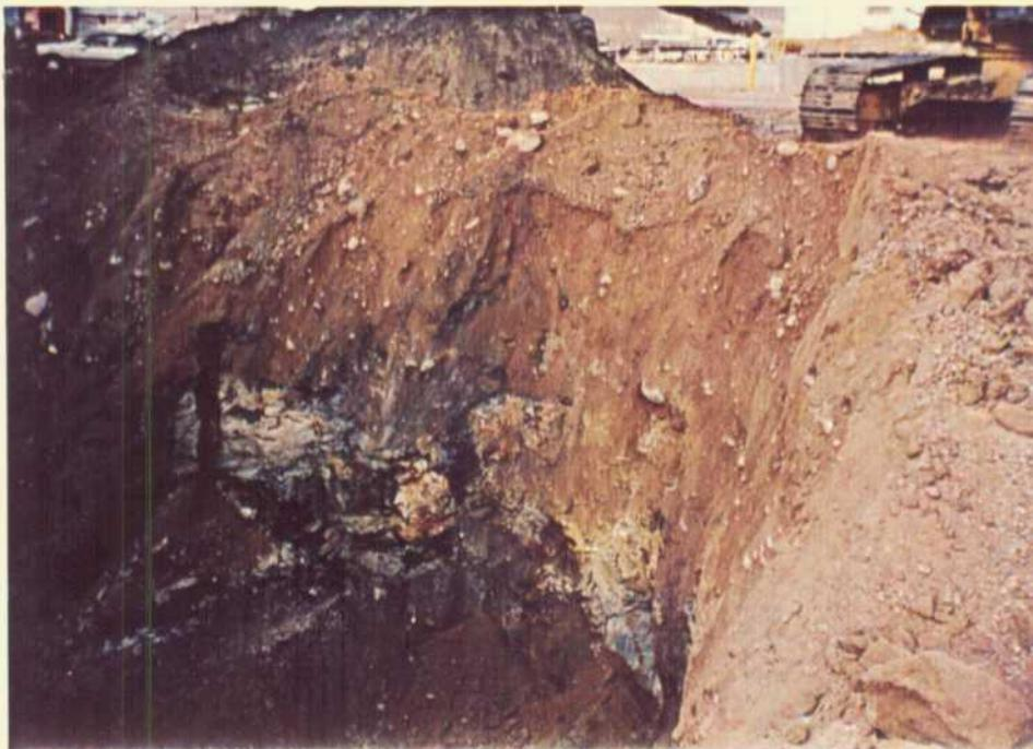
24. View of north wall of completed excavation for southern margin of bedrock plume. The petroleum hydrocarbon contaminants visible in the north wall were sampled for Sample #9111041200. These contaminants were left in place and capped with concrete.
