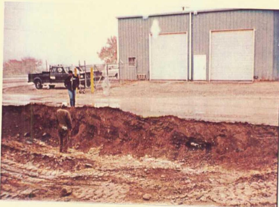
6. View of west wall of excavation adjacent to western margin of the HFTO building. The drain line and leach field that trend to the southwest from the HFTO building are visible in the west wall.
