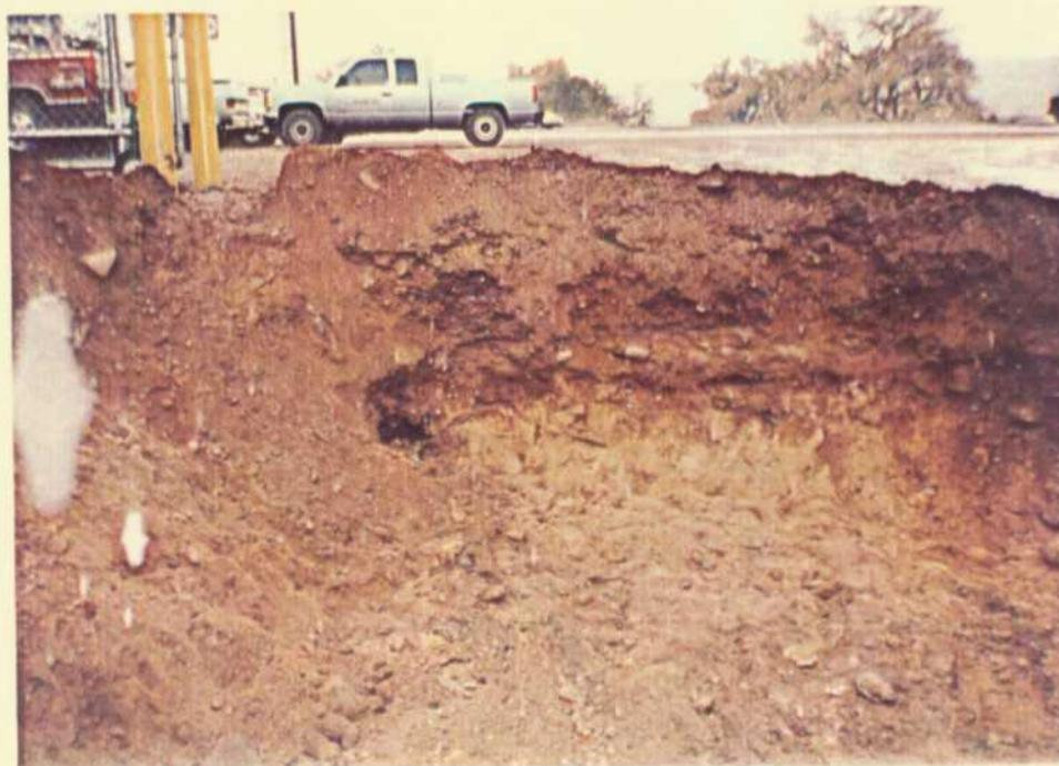
2. Closeup view of southwest corner of excavation adjacent to western margin of HFTO building. Hydrocarbon stain in south wall (left center) is from migration of contaminants from sump inside HFTO building. Hydrocarbon visible in the south wall were excavated and disposed after fence (top left) was dismantled. Unstained sidewall (to right of hydrocarbon stain) is furthest extent of excavation to southwest.
