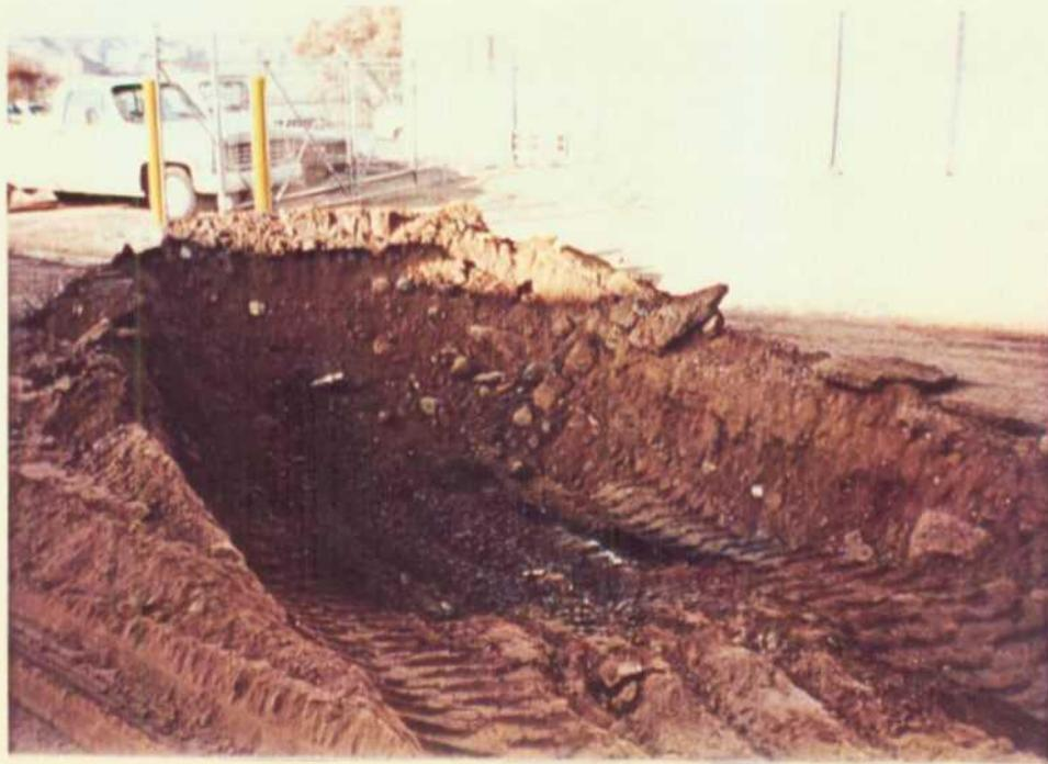
7. Excavation of drain line and leach field that extend to southwest from the HFTO building. Note black hydrocarbon stain in leach field gravels and adjacent soils.
