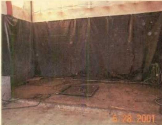
Pic #2 Tool wash bay area with single wall sump connected to water re-cycle system. Sump waste is disposed of by Safety Clean (Albq).
