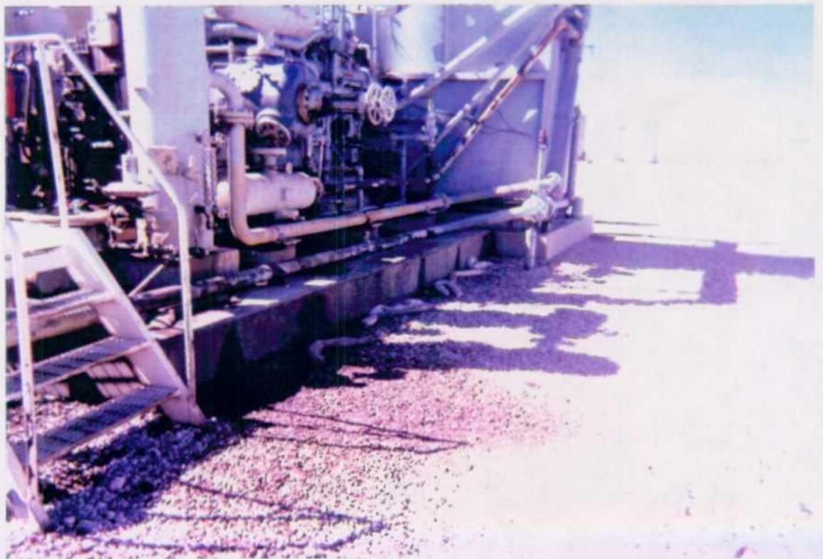
6. Compressor Units. Looking Southwest at Middle Unit near SB-10. Note Surface Contamination and Weep Holes.
