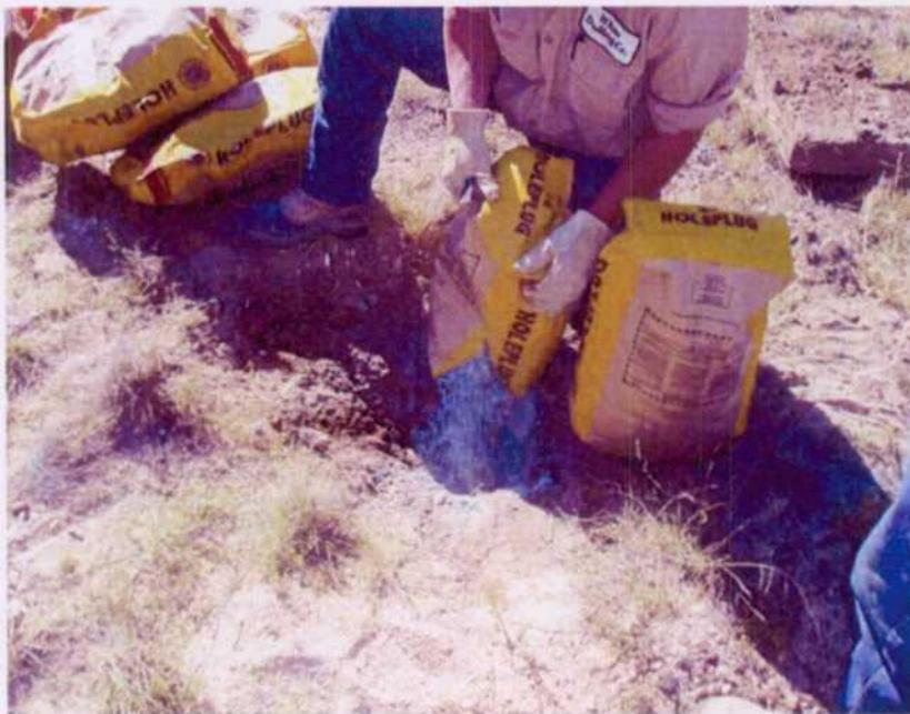
Bentonite chips being top loaded into a monitor well.
