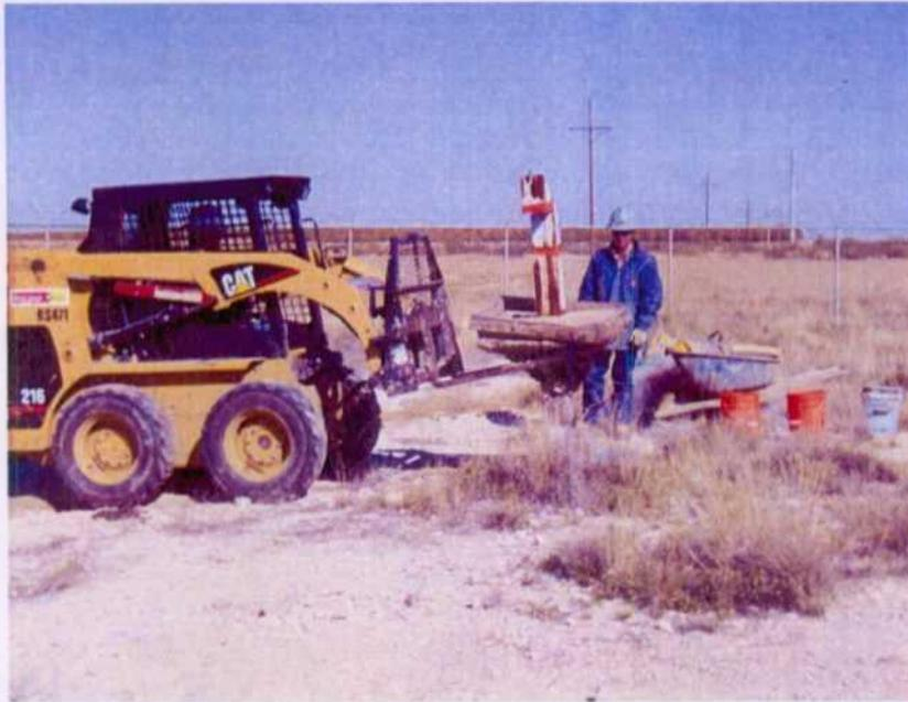
Monitor well surface completion being removed by White Drilling employees.
