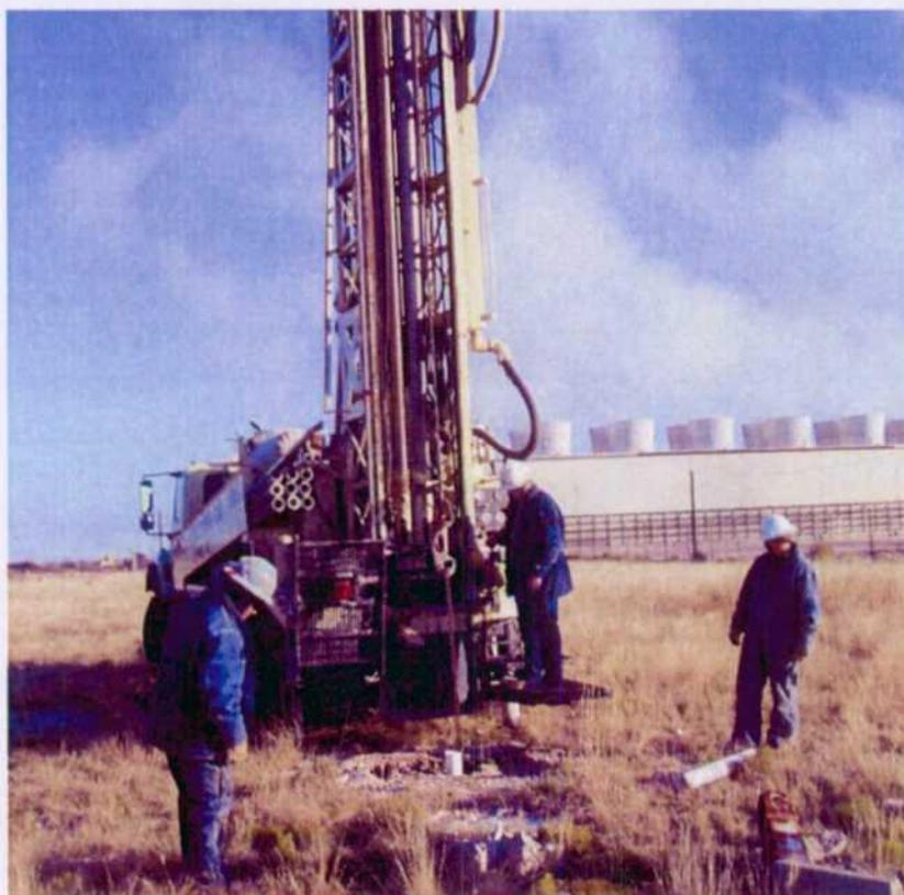
Unsuccessful attempt by White Drilling to remove monitor well casing from the ground.
