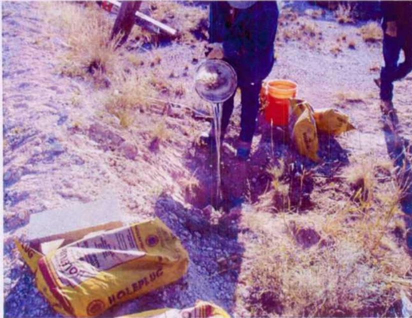
White Drilling employee hydrating bentonite chips at intervals in monitor well.
