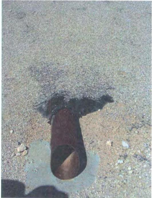
Photo 5: Drain line from berm AST area.
