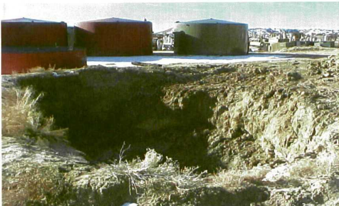
Photo 1: Photograph showing the excavation area as of January 8, 2002.
