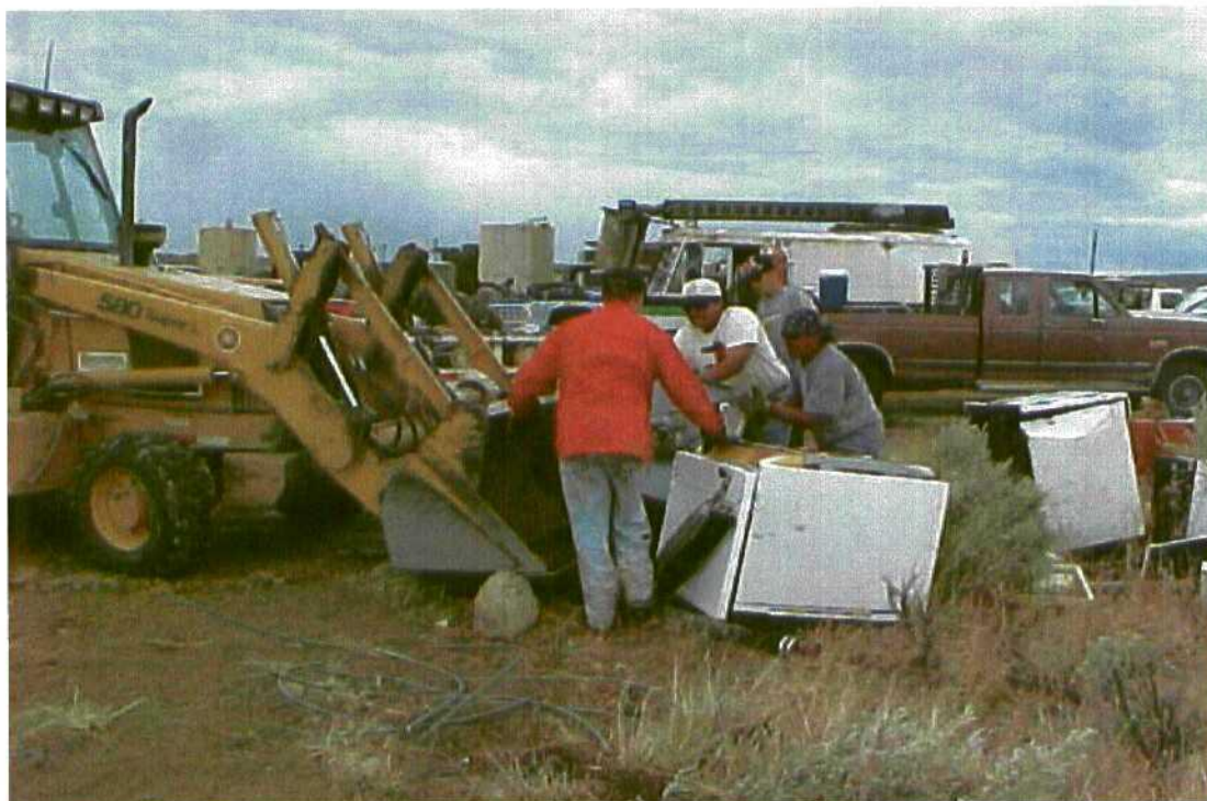
Photo 7: Photograph showing the loading of scrap metal in preparation for shipment to San Juan Recycling.
