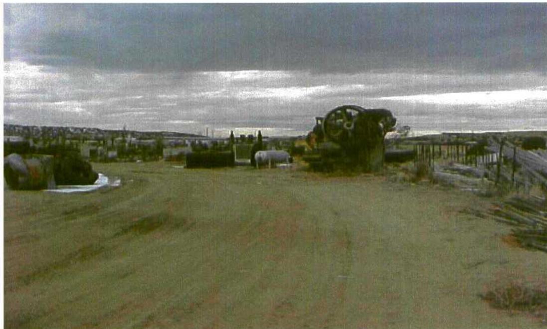
Photo 4: Photograph showing the northern boundary of the yard after the removal of over 300 containers of various sizes.
