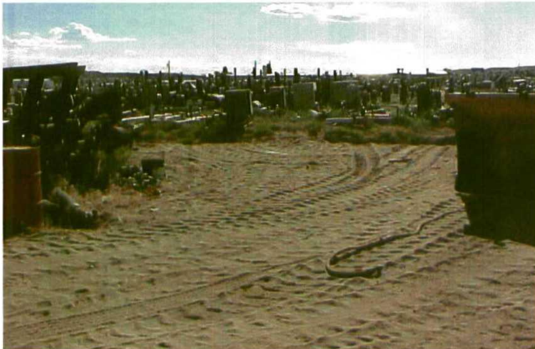
Photo 5: Photograph showing cells J-3 and K-3 after removal of debris.
