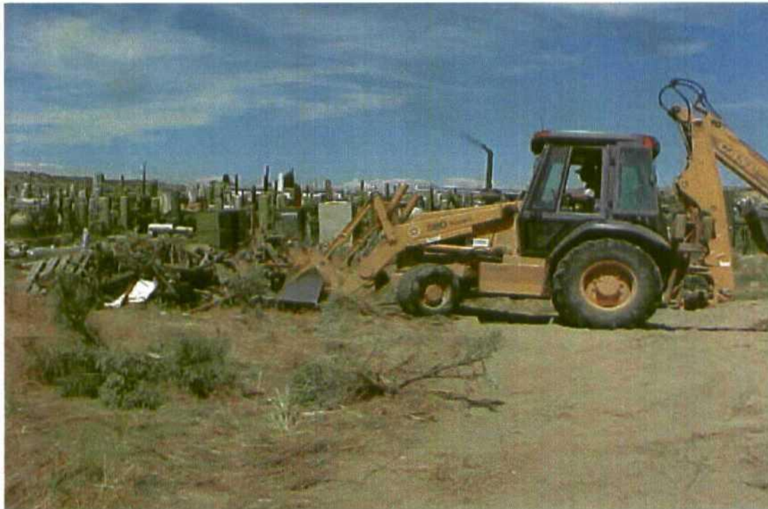
Photo 3: Photograph of the backhoe removing debris from the arroyo.
