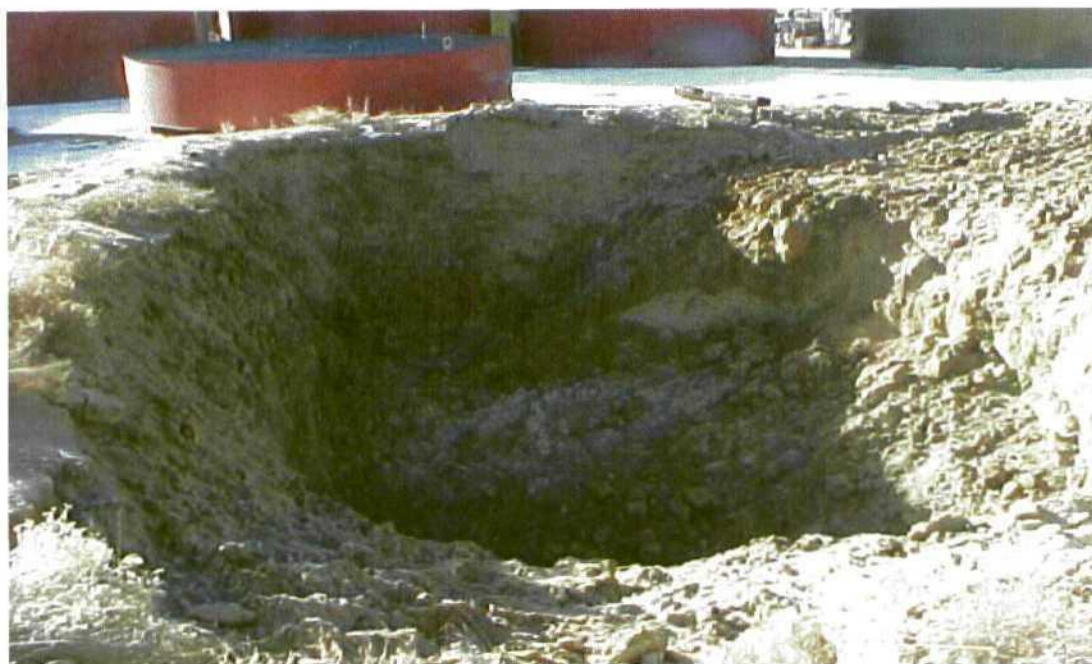
Photo 2: Photograph showing the excavation area as of January 8, 2002.
