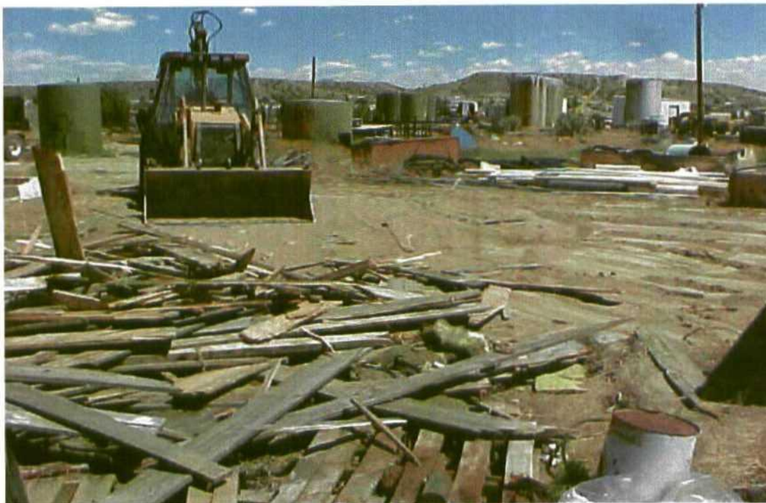
Photo 2: Photograph showing the backhoe removing debris from cell J-4.
