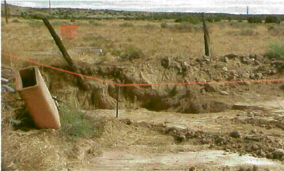
Photo 1: Photograph showing the excavation located along the northern boundary of the CIP yard.
