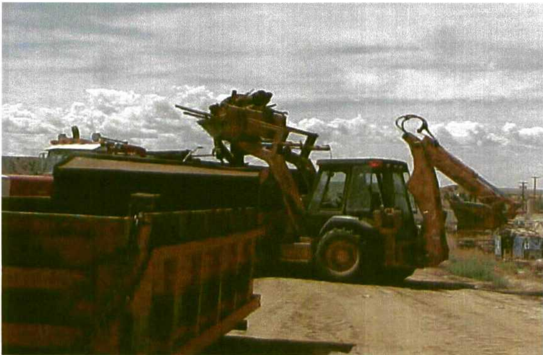
Photo 4: Photograph showing the backhoe loading various non-hazardous debris in preparation for transportation to the San Juan County Landfill.
