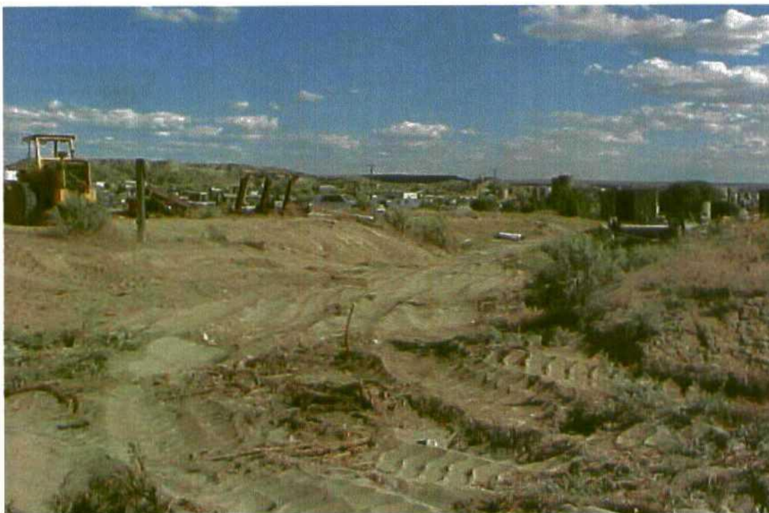
Photo 6: Photograph facing northwest showing the arroyo during the removal of debris.
