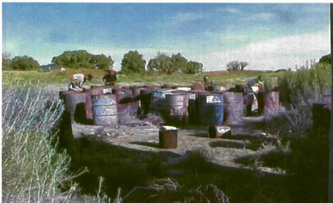
Photo 1: Photograph showing the de-heading process continuing into July 5, 2001.
