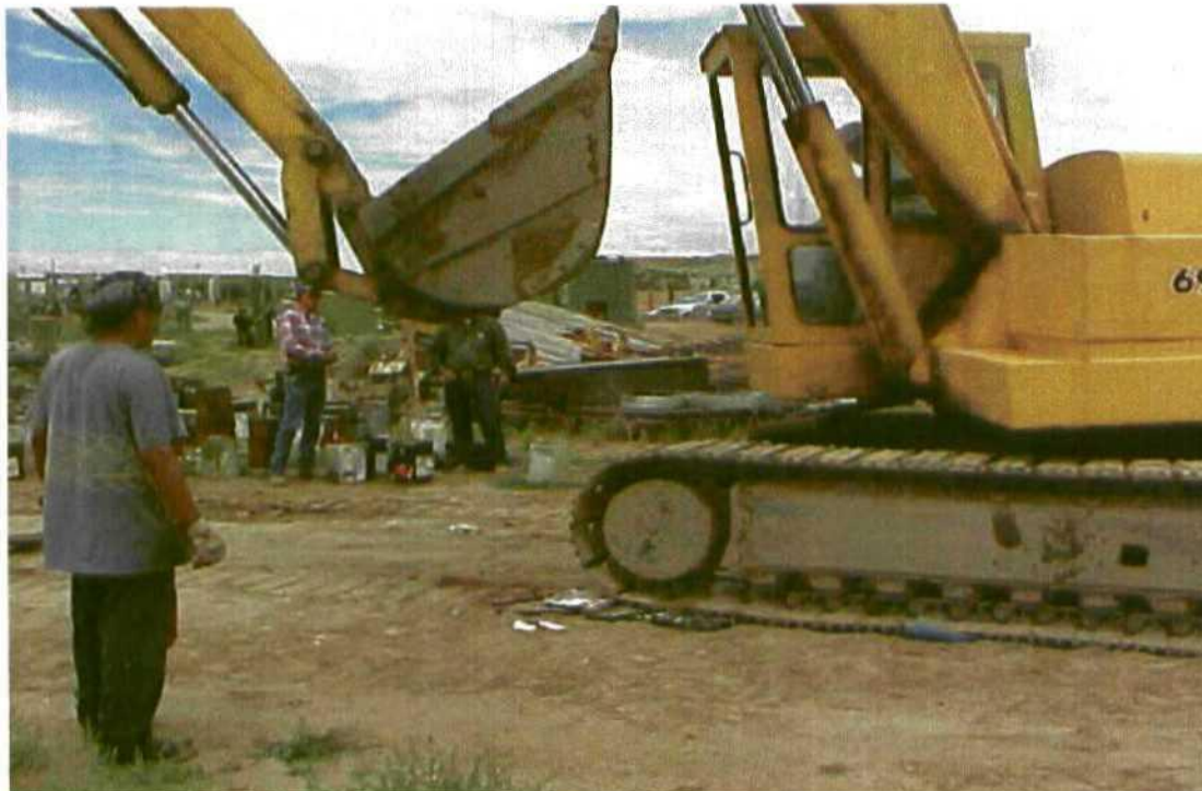
Photo 4: Photograph showing the track hoe crushing empty 5-gallon steel containers. This method was employed to conserve space when shipping scrap metal. (cells K-2 and L-2).
