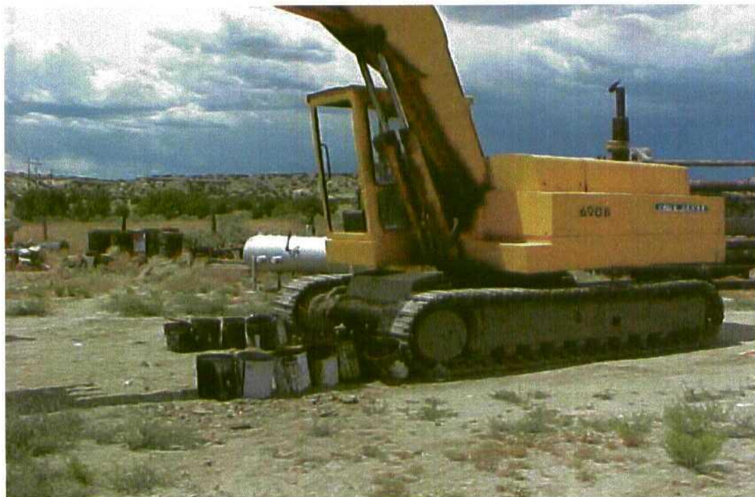
Photo 1: Photograph showing the track hoe crushing empty 5-gallon containers in preparation for transport to San Juan Recycling.
