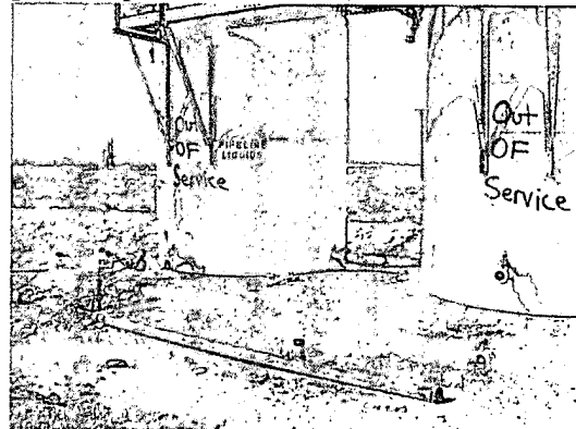
Photo 11: Old tank batteries not in service, in process of removing.
