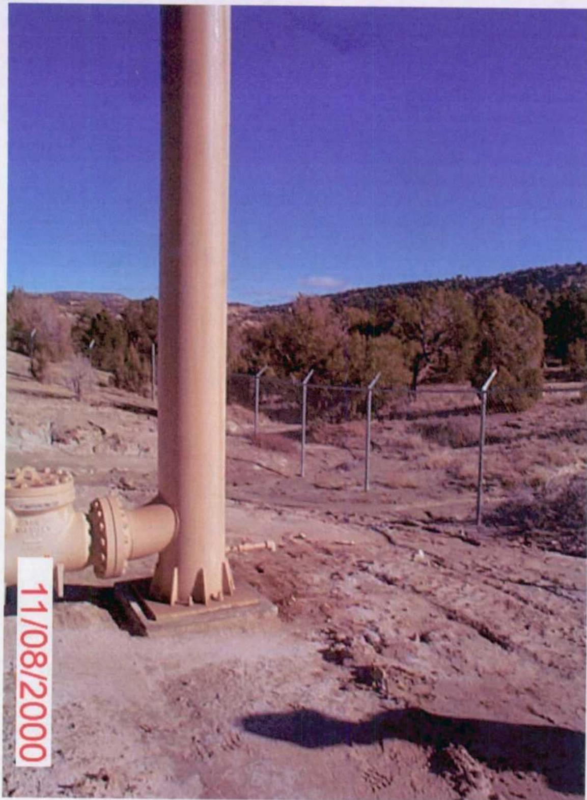
Picture #2- Plant ESD and normal vent stack located east of plant.
