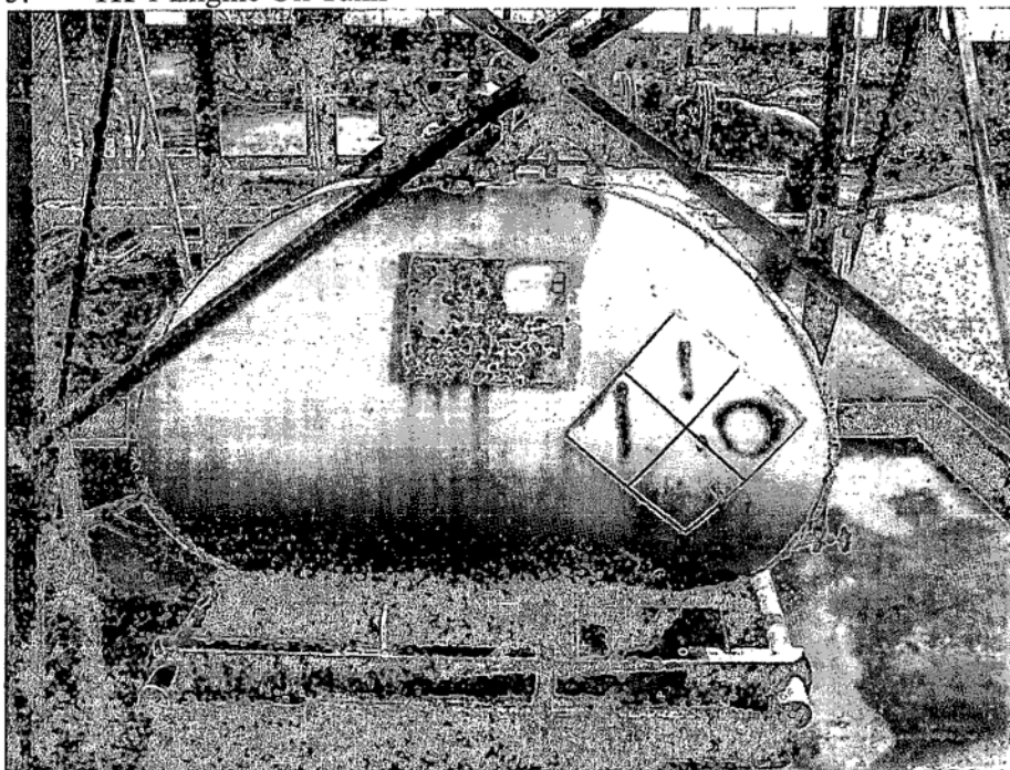
FIGURE 6: TK-2 Antifreeze Tank
