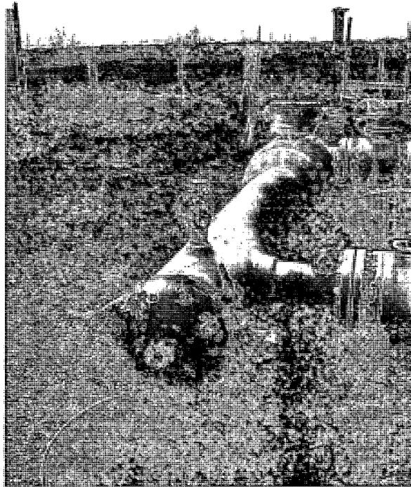
FIGURE 8: TK-5 Pig Receiver Drip Pan
