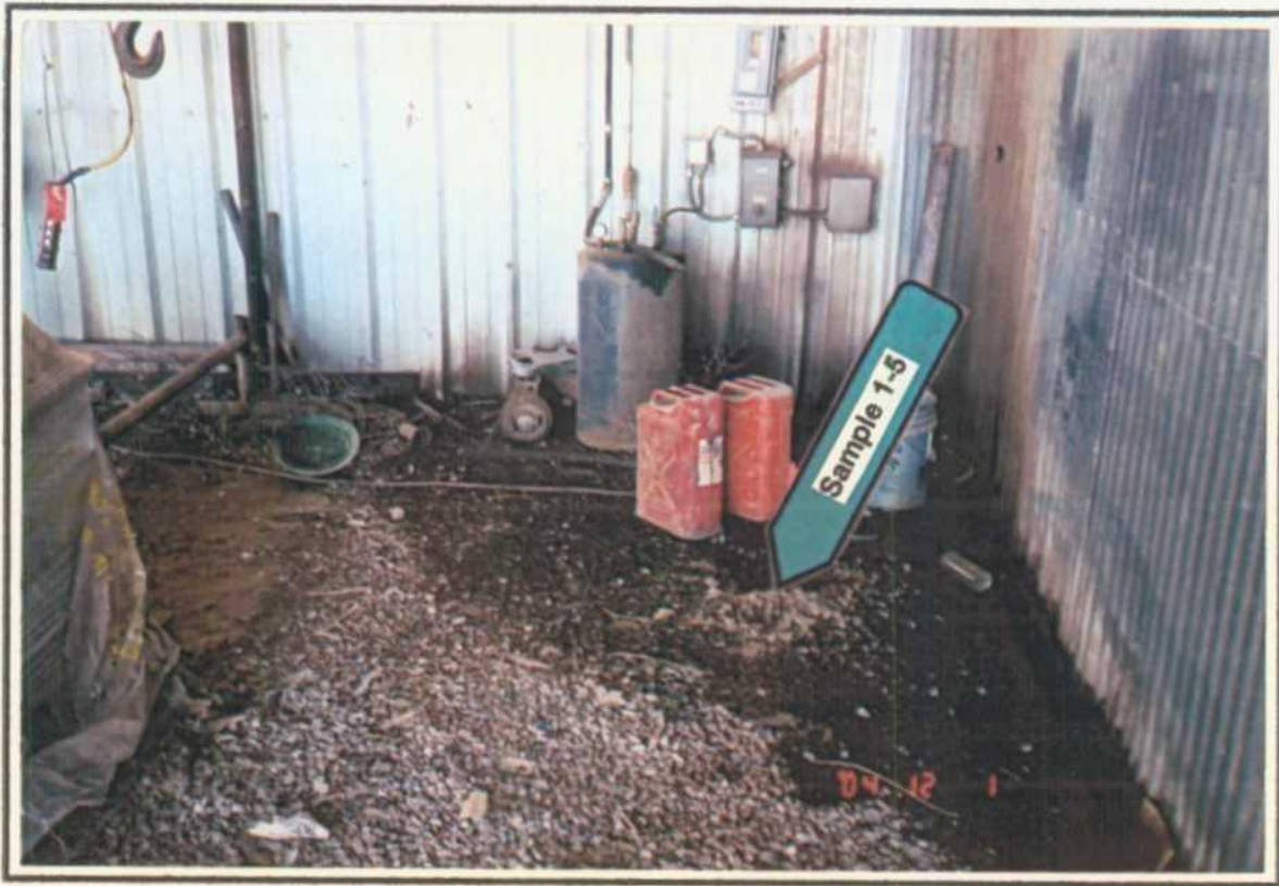
Photograph 3: Sample 1-5 was located in the southwest corner of the Covered Work Area.
