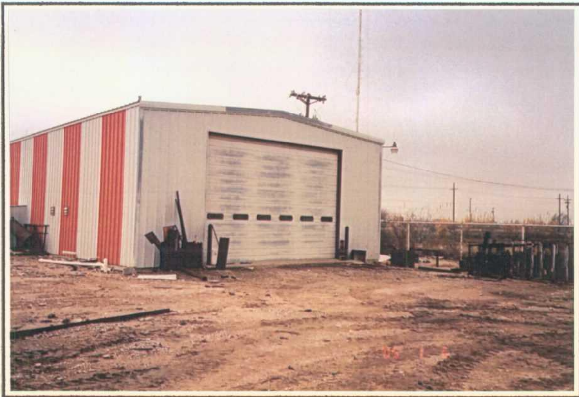
Photograph 13: The former Welding Shop was located near the west perimeter fence.
