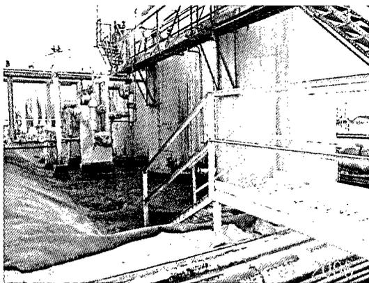
Oil Treater area housekeeping issue (oil, dirt, water observed inside of berm) and poses a possible fire hazard
