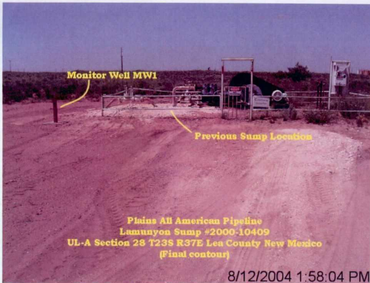
Photograph 7 – Looking northerly after sump removal.
