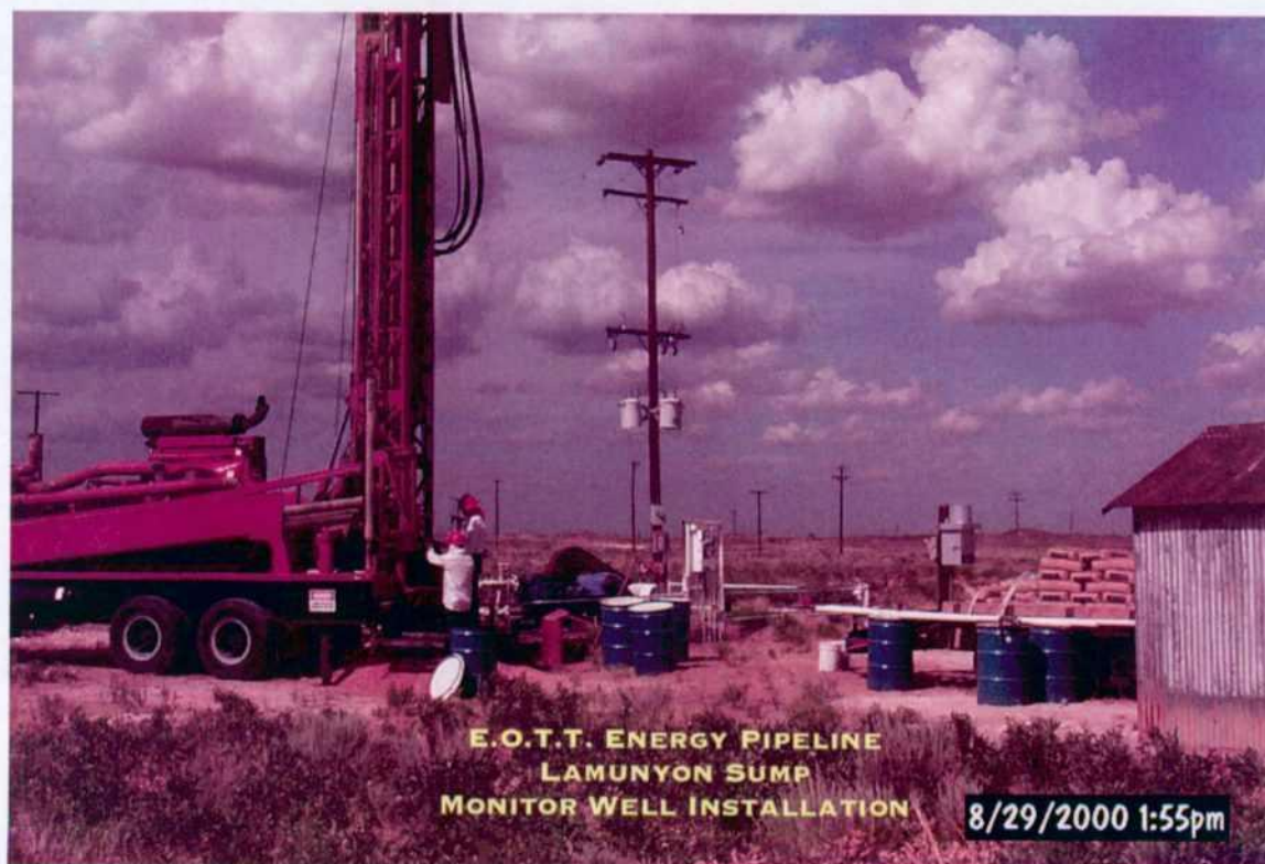
Photograph 4 – Monitor well installation.
