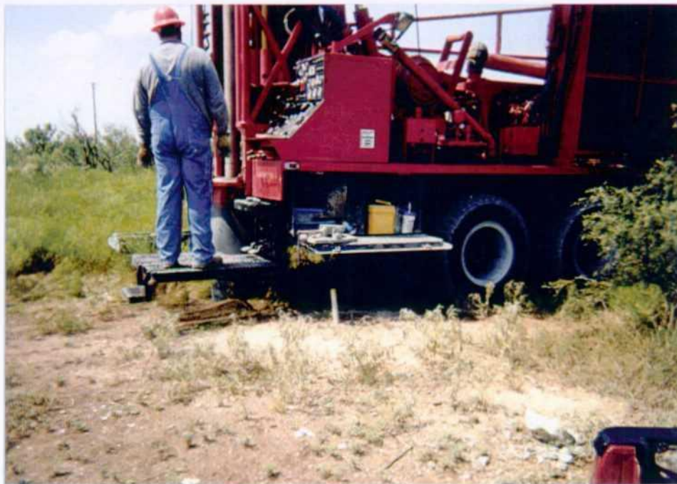
Photo 7: Drilling of monitor well MW-4.
