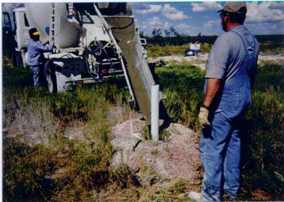
Photo 6: Installation of monitor well MW-3.
