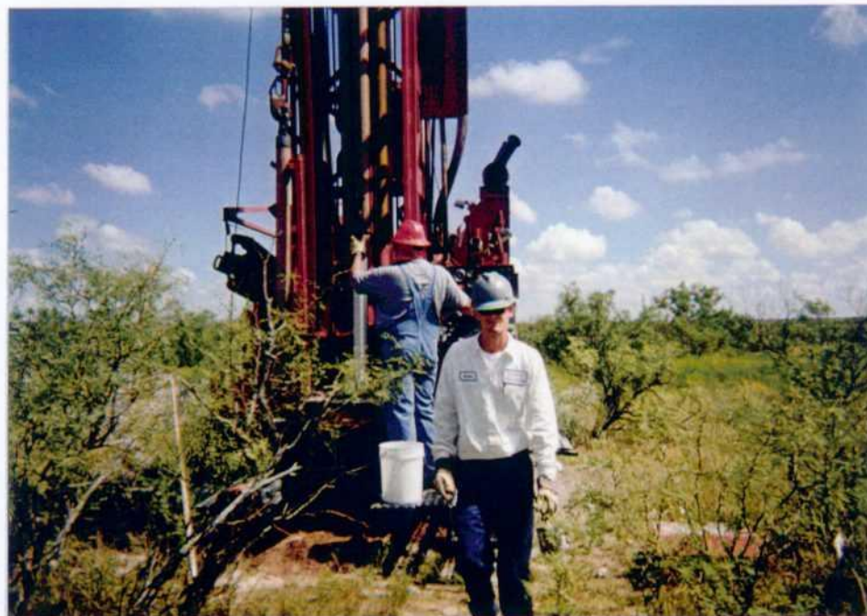
Photo 4: Installation of monitor well MW-2.
