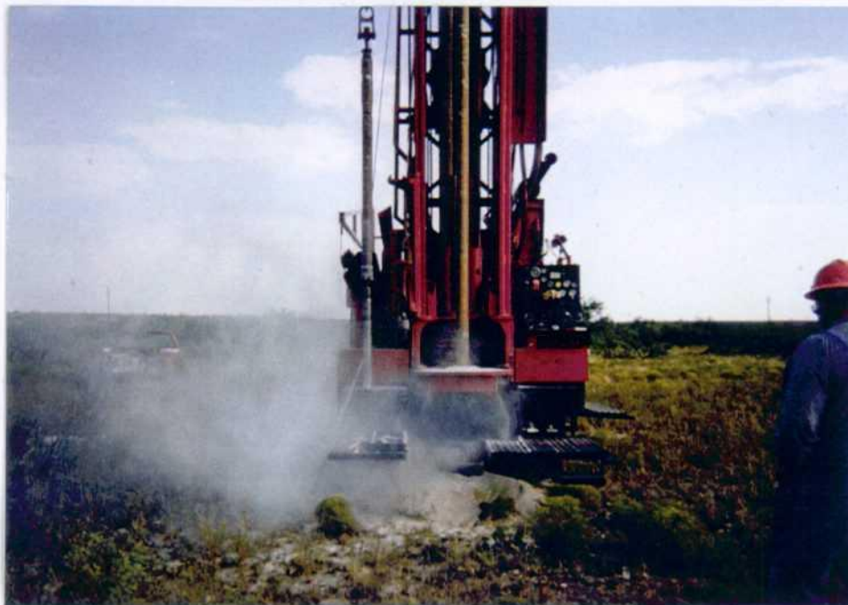
Photo 1: Drilling of monitor well MW-1.
