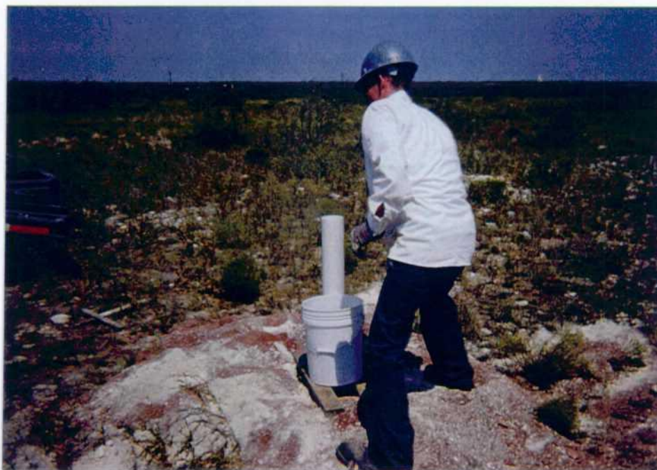
Photo 2 : Installation of monitor well MW-1.
