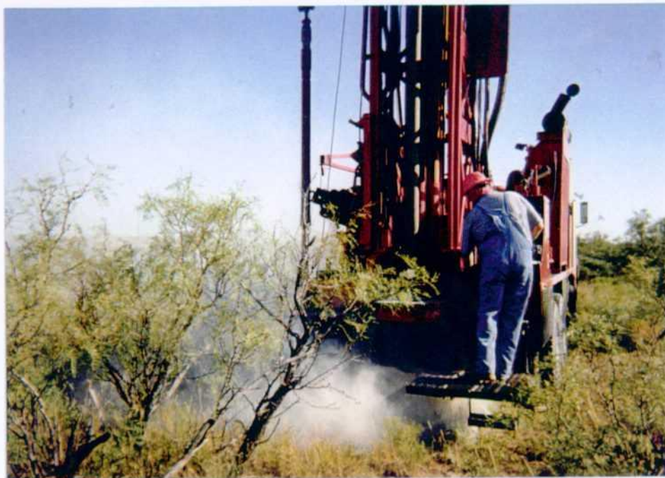
Photo 3: Drilling of monitor well MW-2.
