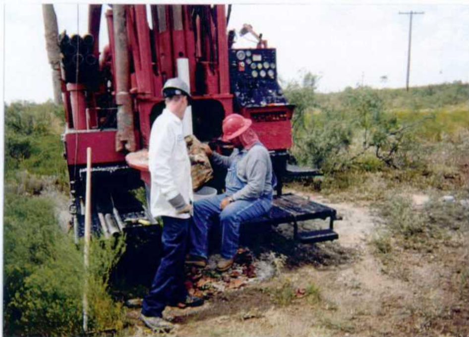
Photo 8: Installation of monitor well MW-4.
