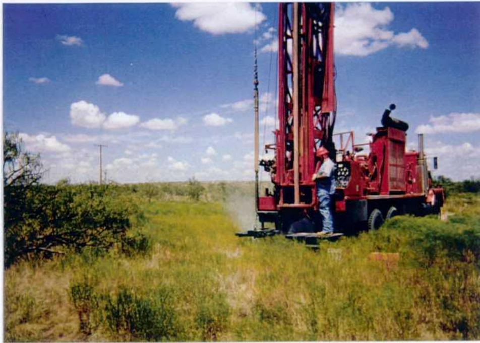
Photo 5: Drilling of monitor well MW-3.
