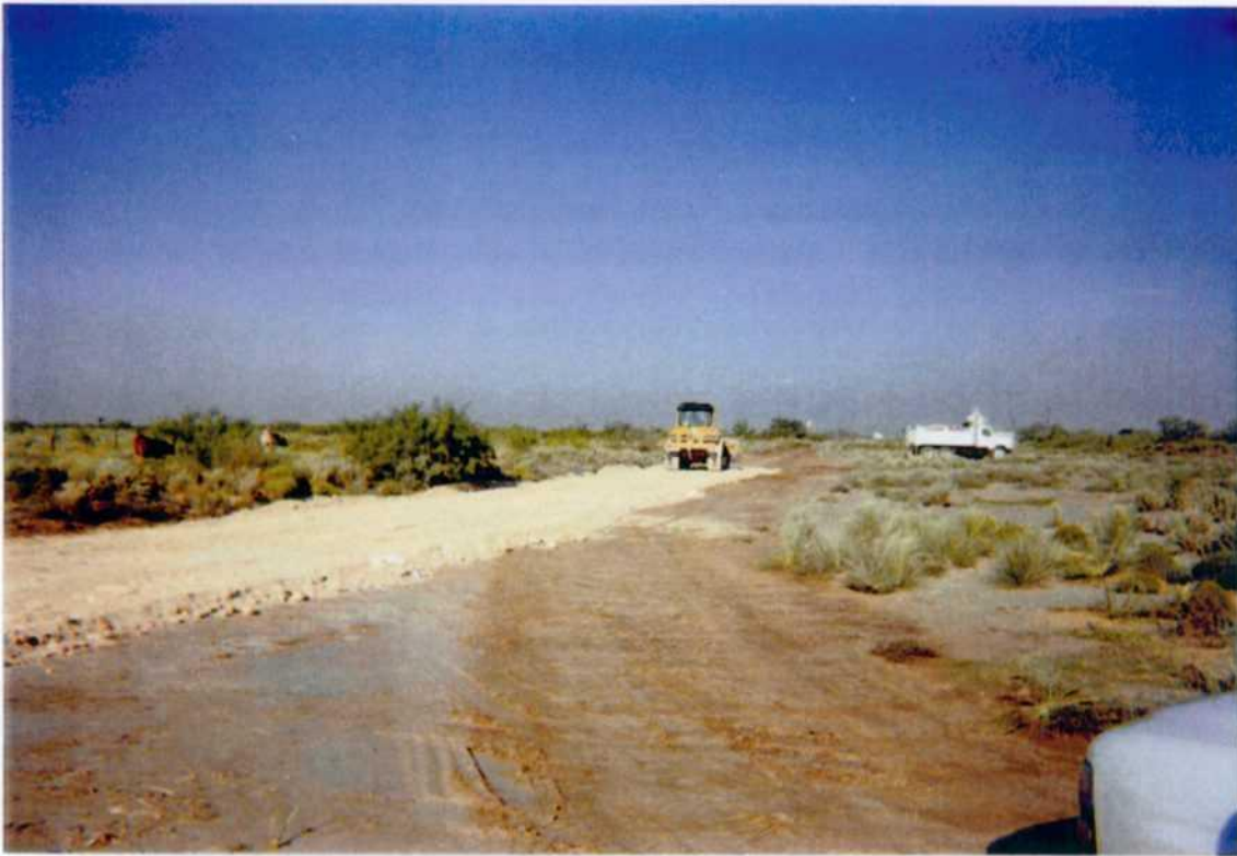
Photo 23: Repairs to dirt road.
