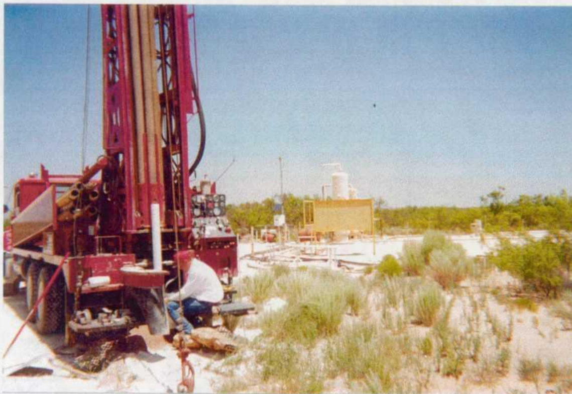
Photo 2: 6/25/01. Looking northeast. Setting monitor well MW-1. Well set at 42 feet below ground surface.
