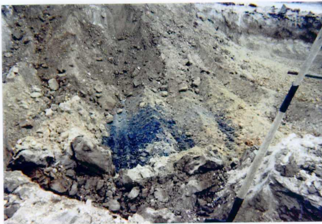
Photo 2: Excavation of Site 1.
