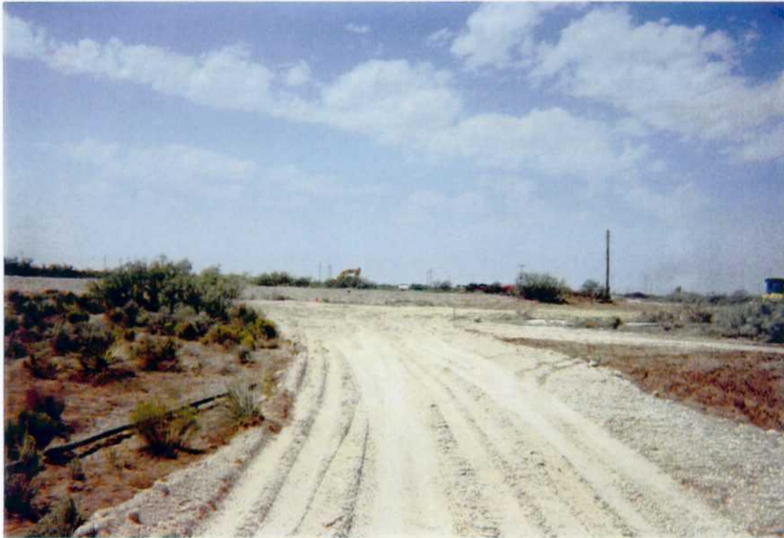
Photo 24: Repairs to dirt road.
