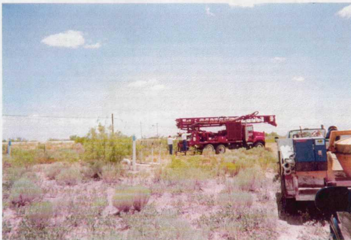
Photo 10: 6/25/01. Looking south. Setting up to drill soil boring SB-1. Note pipeline markers in foreground and Highway 8 at left (east).
