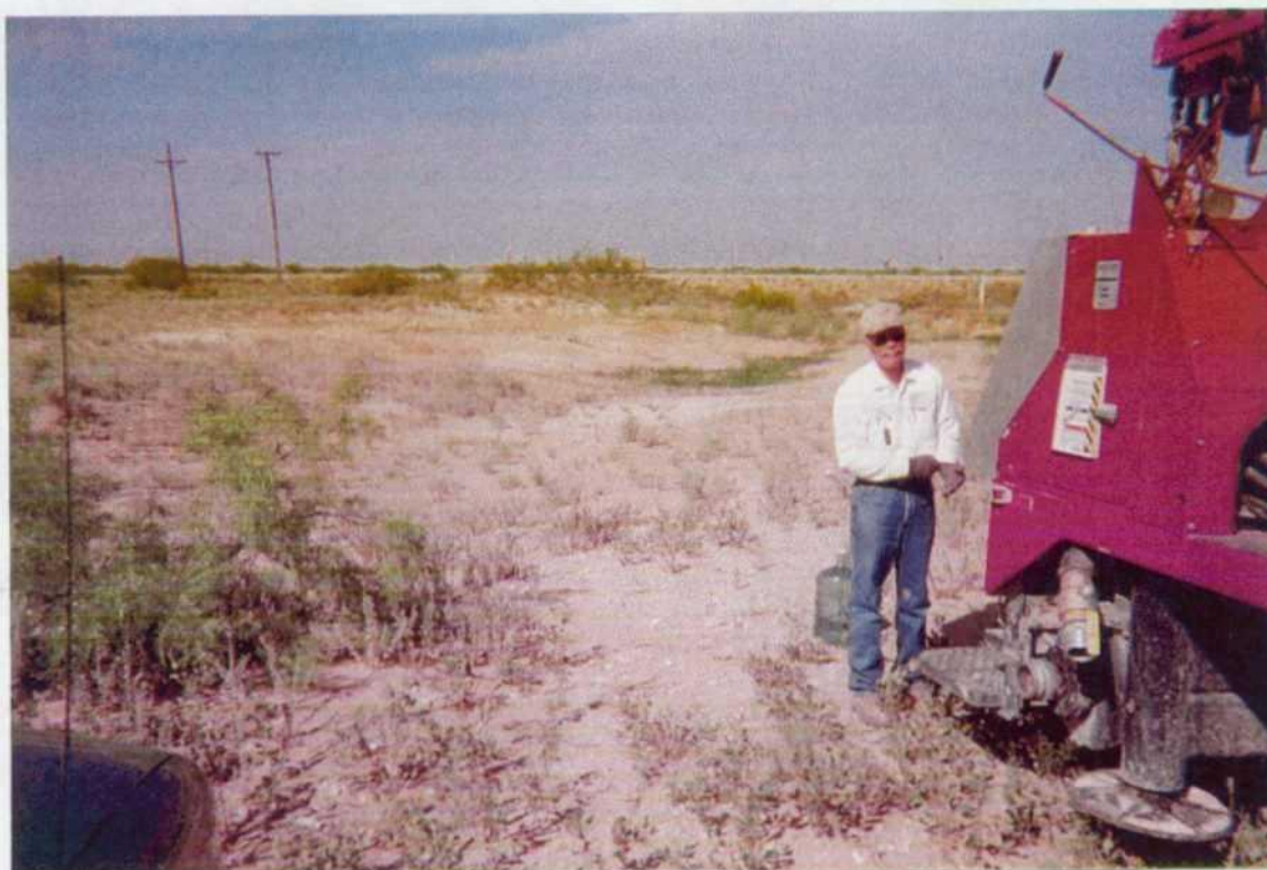
Photo 6: 6/26/01. Looking southwest. Drill rig set up at monitoring well MW-3. Note drainage area in background and pipeline marker at right.
