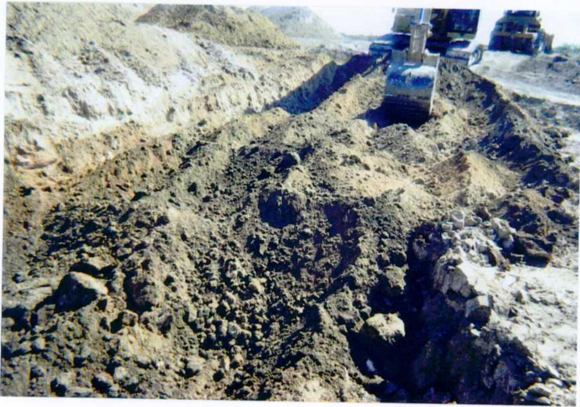
Photo 20: Excavation of Site3.
