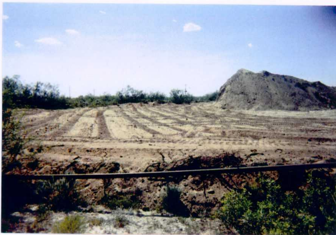
Photo 9: Completed backfilling of Site 2 (westpit).
