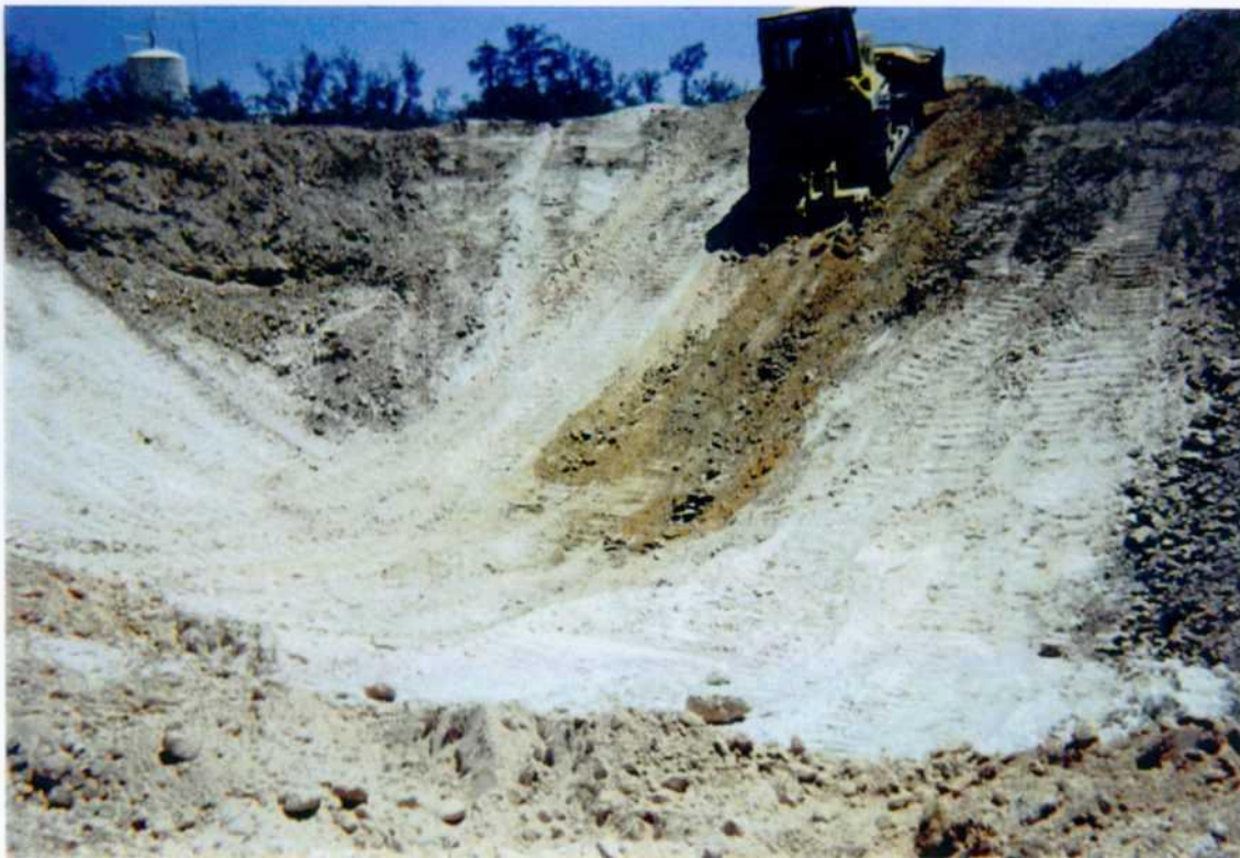
Photo 11: Excavation of Site 2 (eastpit).
