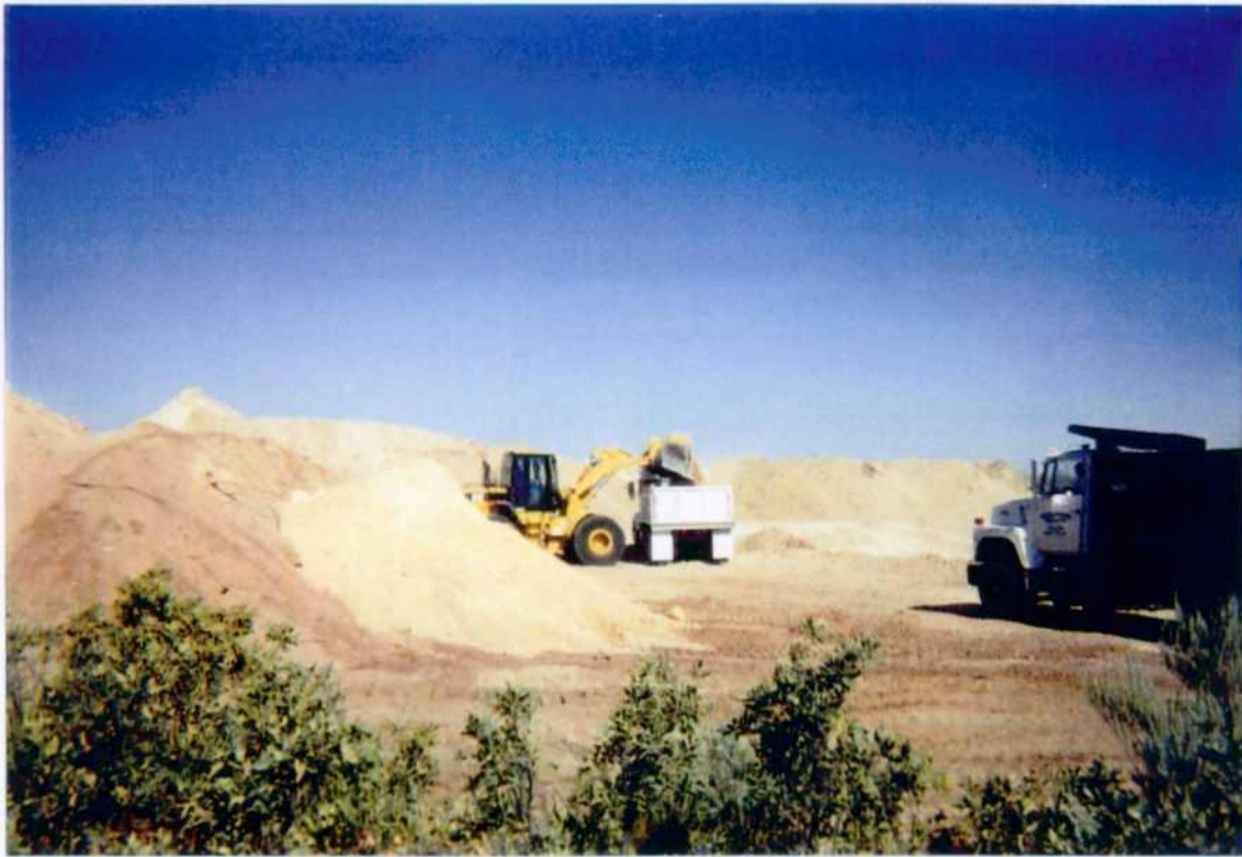
Photo 17: Backfilling of Site 2 (eastpit).
