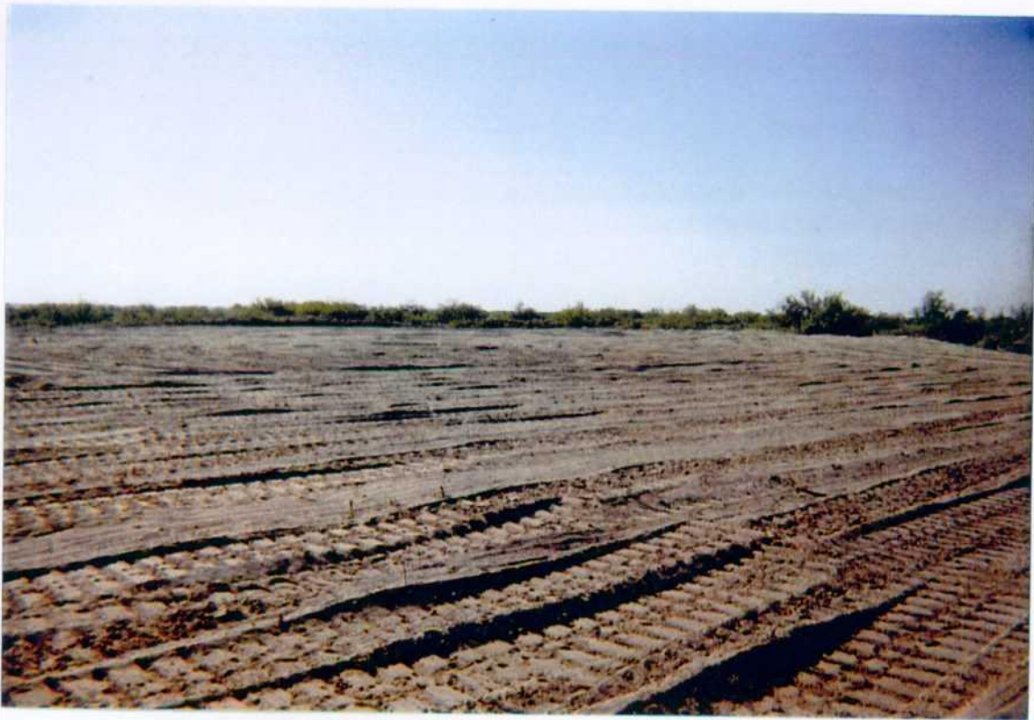
Photo 19: Completed backfilling of Site 2 (eastpit).
