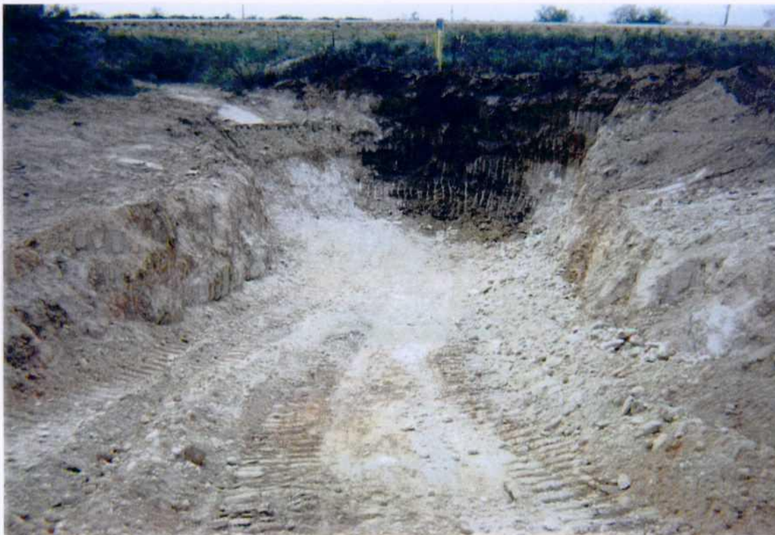
Photo 21: Excavation of Site 3.
