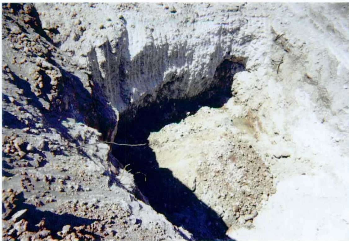
Photo 16: Excavation of northside of Site 2 (eastpit).
