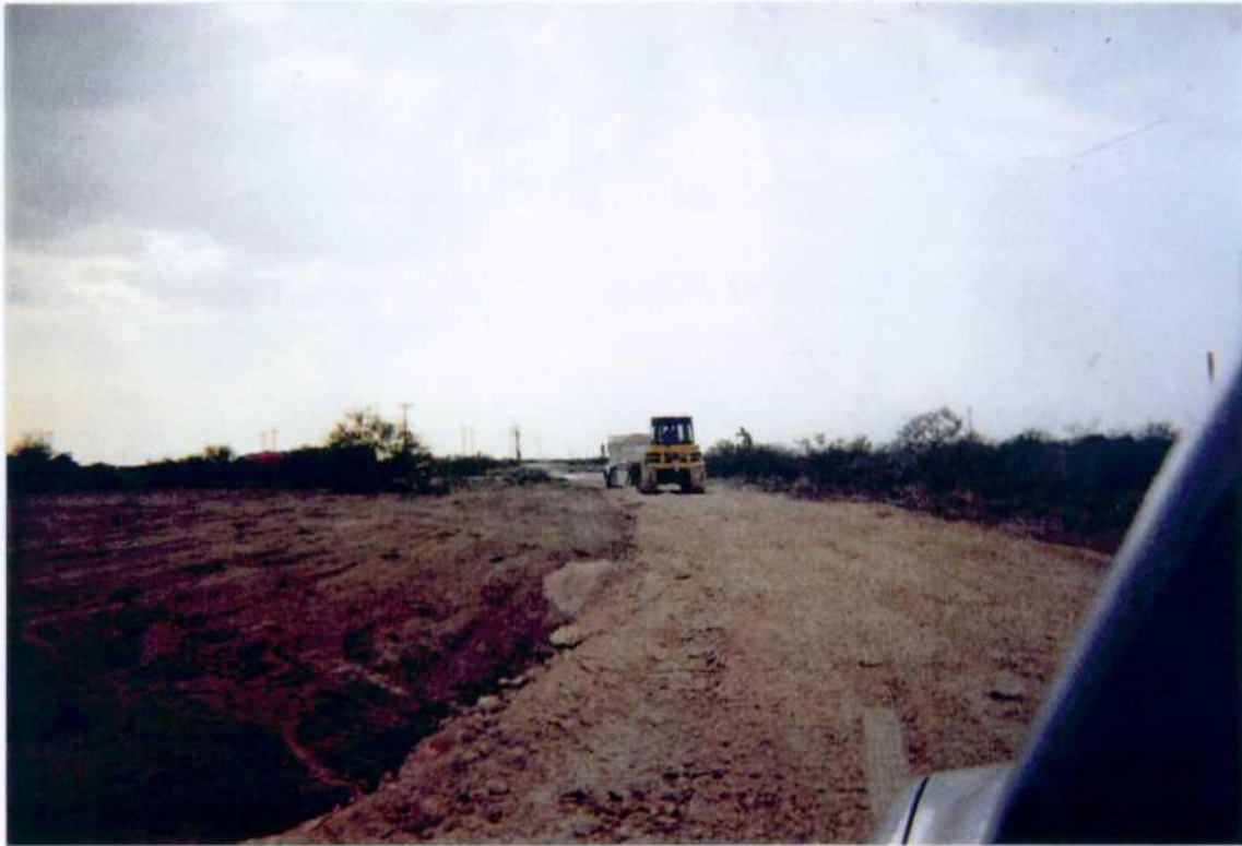
Photo 6: Completed backfilling of Site 1.
