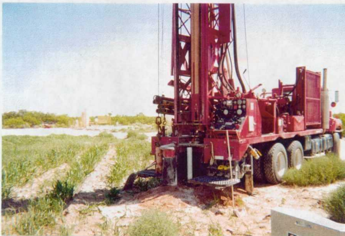
Photo 4: 6/25/01. Looking north-northeast. Setting monitor well MW-2.
