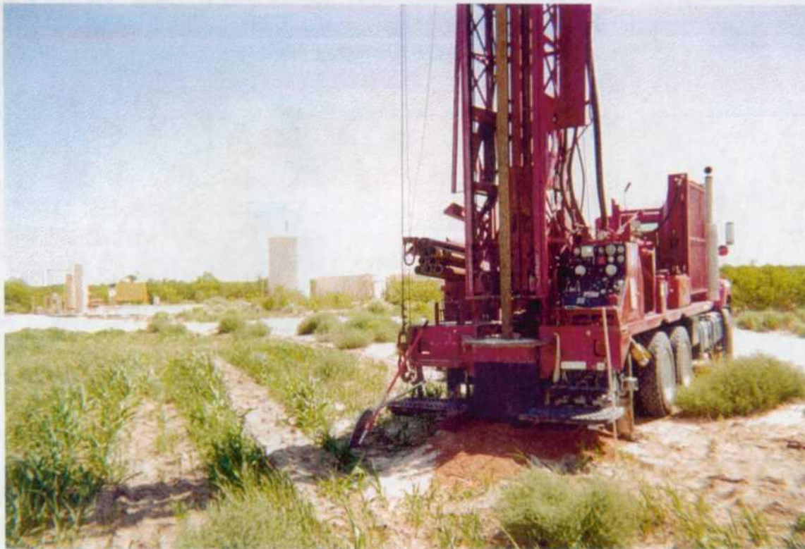
Photo 3: 6/25/01. Looking north-northeast. Drilling monitor well MW-2 at southeast edge of "Site 2" excavation. Note former excavation has been re-planted.
