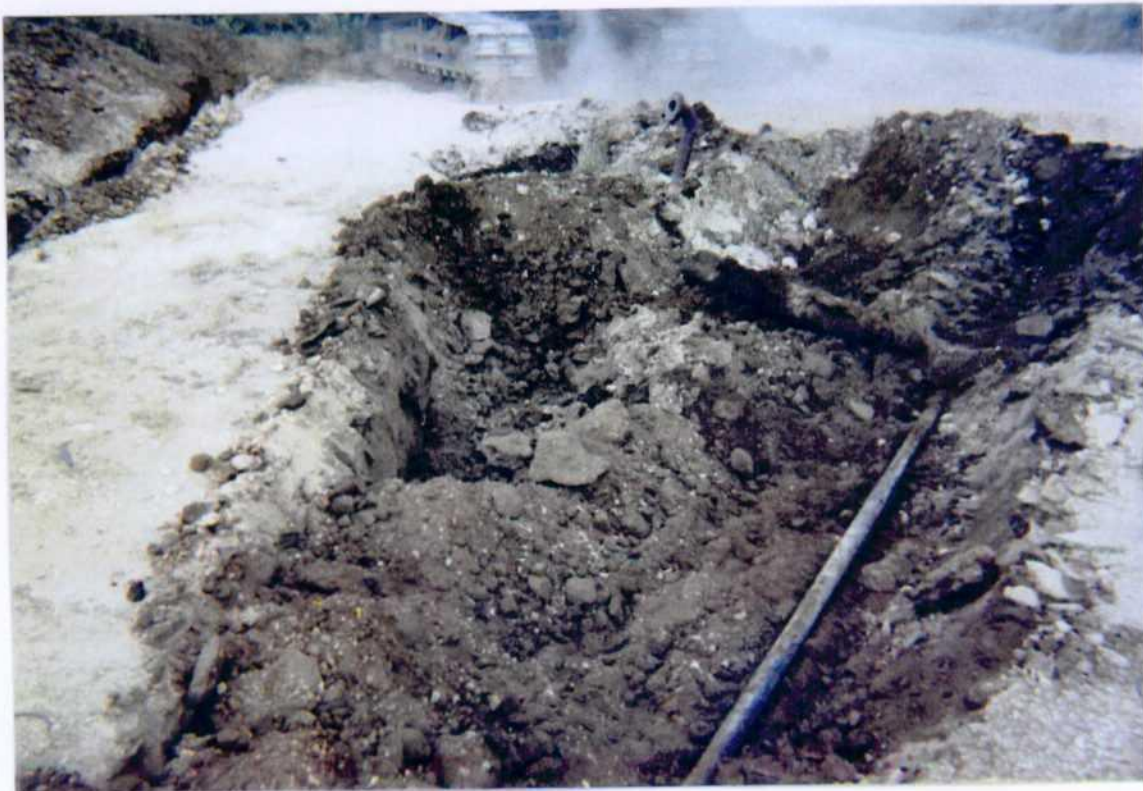
Photo 1: Excavation of Site 1.
