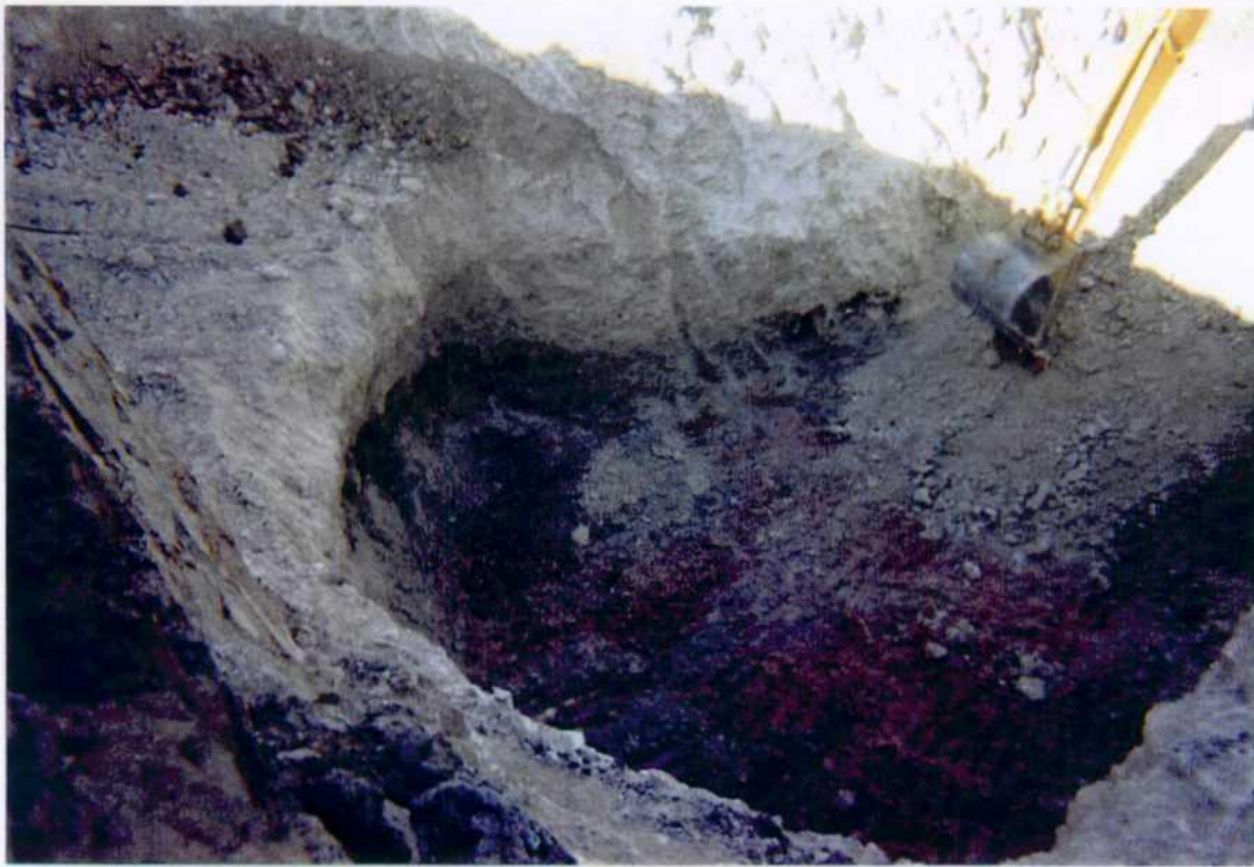
Photo 5: Excavation of Site 1.
