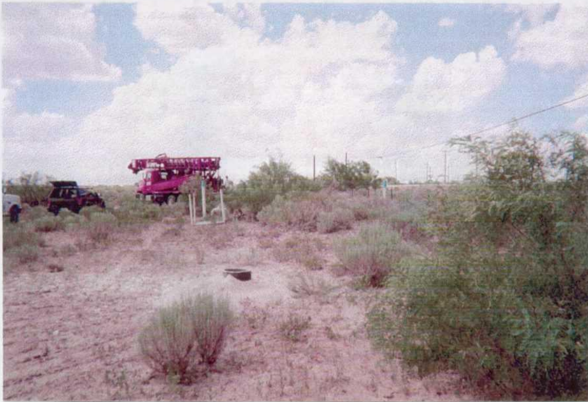
Photo 11: 6/25/01. Looking north. Setting up to drill soil boring SB-2. Note SB-1 in foreground. Pipeline markers and Highway 8 at right (east).
