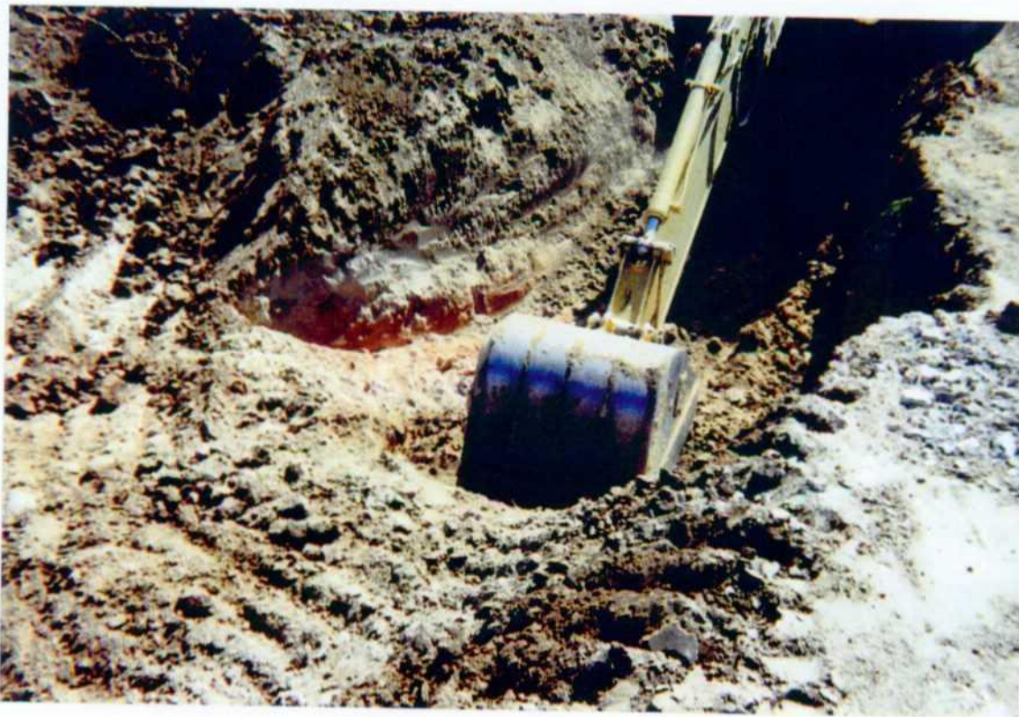
Photo 8: Excavation of Site 2 (westpit).
