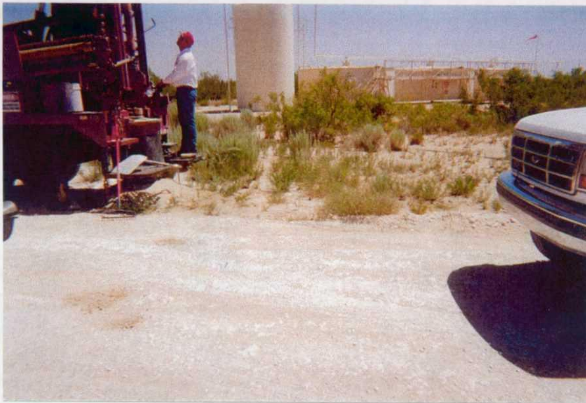
Photo 1: 6/25/01. Looking northeast. Set up to drill monitor well MW-1 located adjacent to southeast side of former "Site 1". Excavation completed August 18, 2000.
