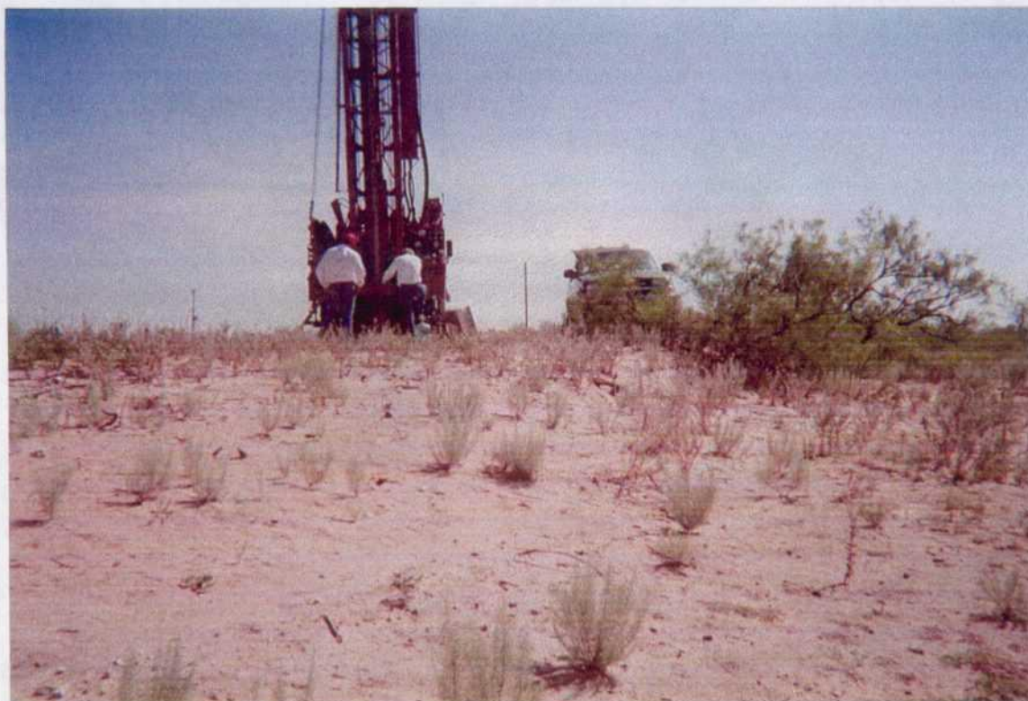
Photo 7: 6/26/01. Looking northeast. Setting up to drill monitor well MW-3. Note slope of drainage area. MW-3 was completed on southeast edge of former excavation "Site 3".
