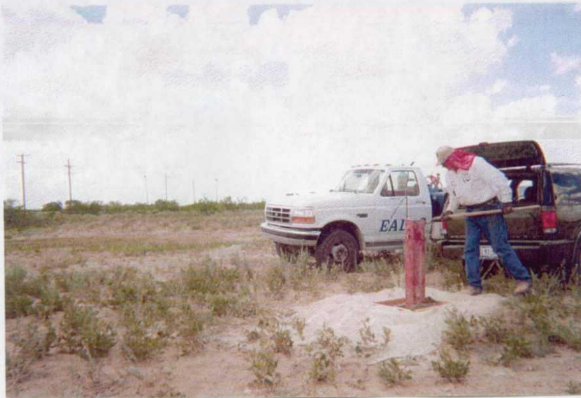
Photo 9: 6/26/01. Looking north. Completing monitor well MW-3.
