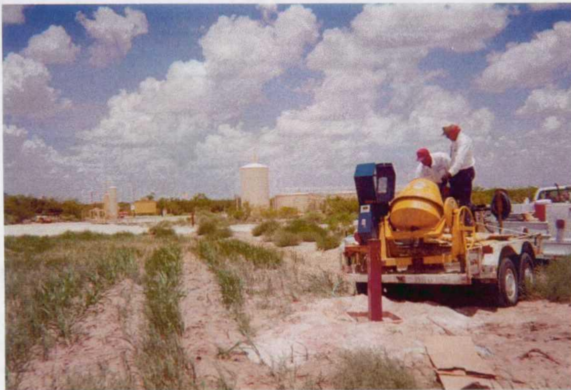
Photo 5: 6/26/01. Looking northeast. Completing monitor well MW-2. Note completed monitor well MW-1 in background.
