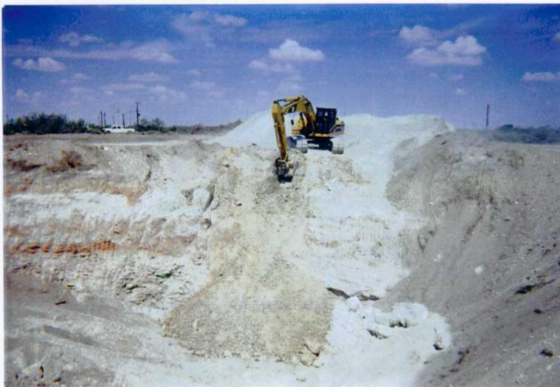
Photo 15: Extension of ramp to north for Site 2 (eastpit).
