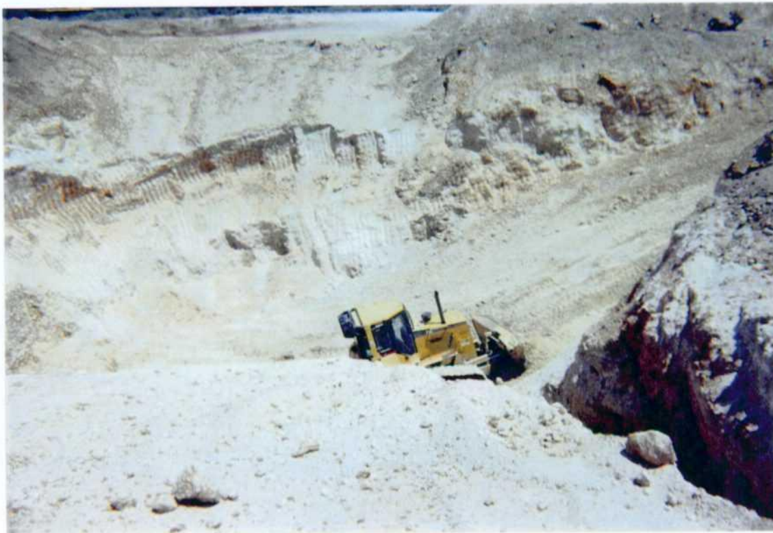
Photo 12: Excavation of Site 2 (eastpit).
