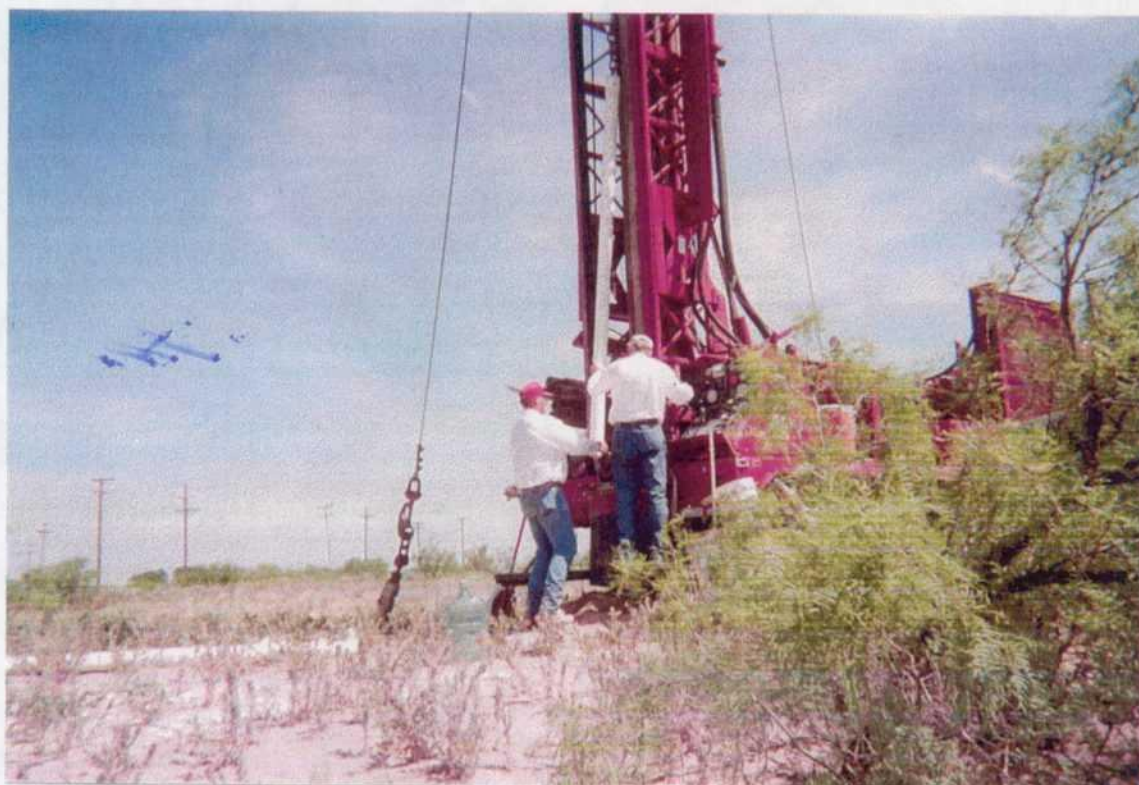
Photo 8: 6/26/01. Looking north. Setting monitor well MW-3.
