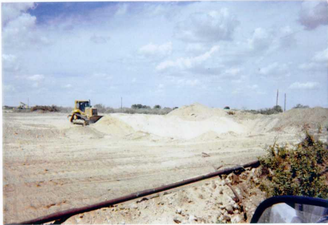
Photo 18: Backfilling of Site 2 (eastpit).
