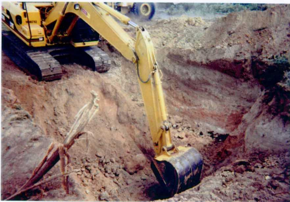
Photo 7: Excavation of Site 2 (westpit).
