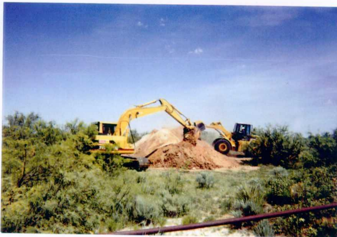
Photo 10: Stockpiling of overburden soil from Site 2 (eastpit).
