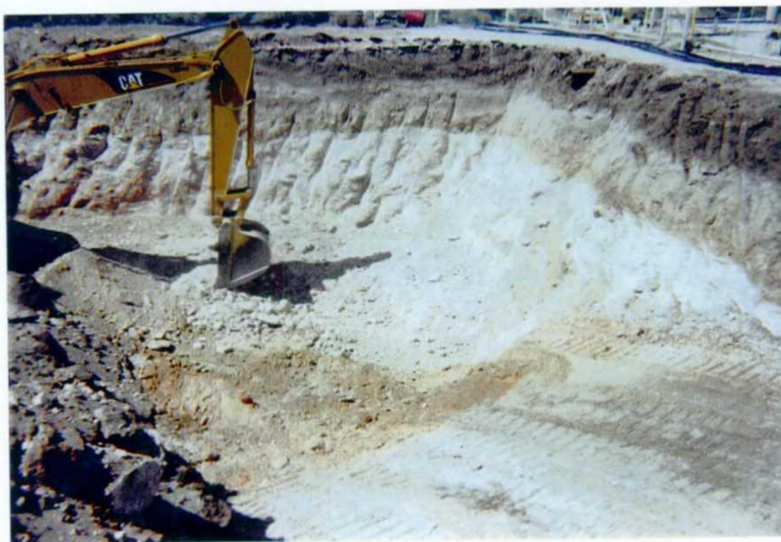
Photo 4: Excavation of Site 1.
