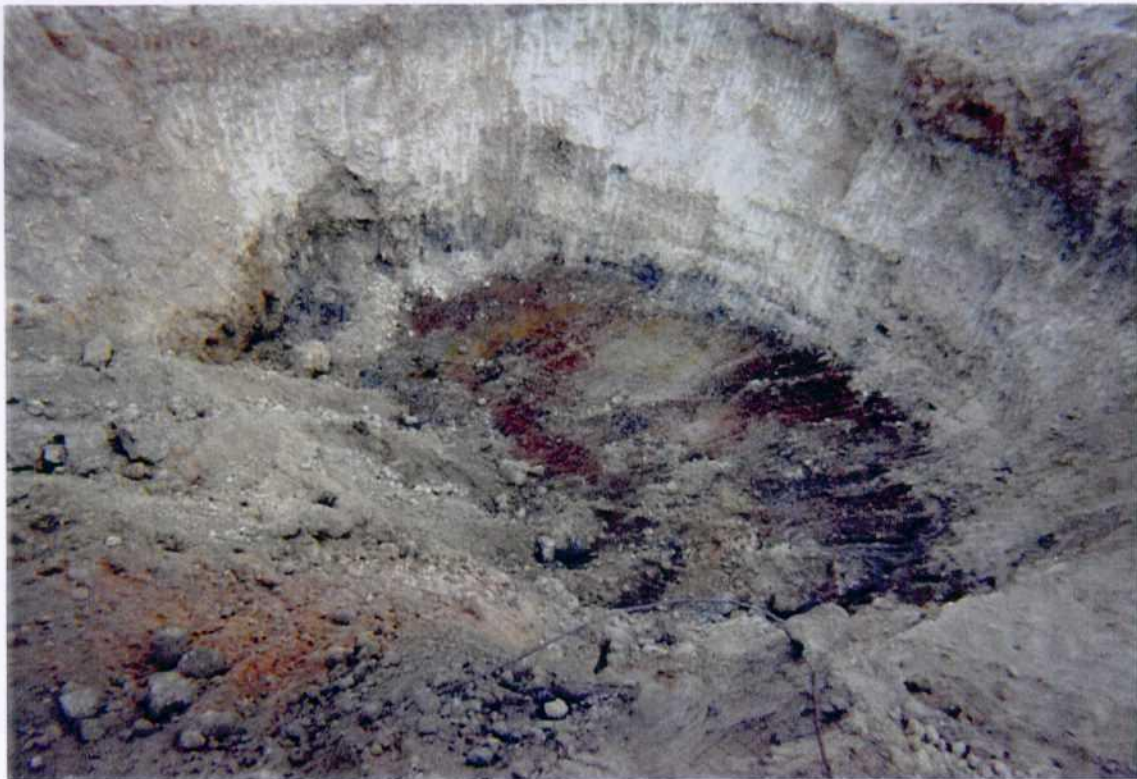
Photo 13: Excavation of Site 2 (eastpit) 35 feet depth in redbed.
