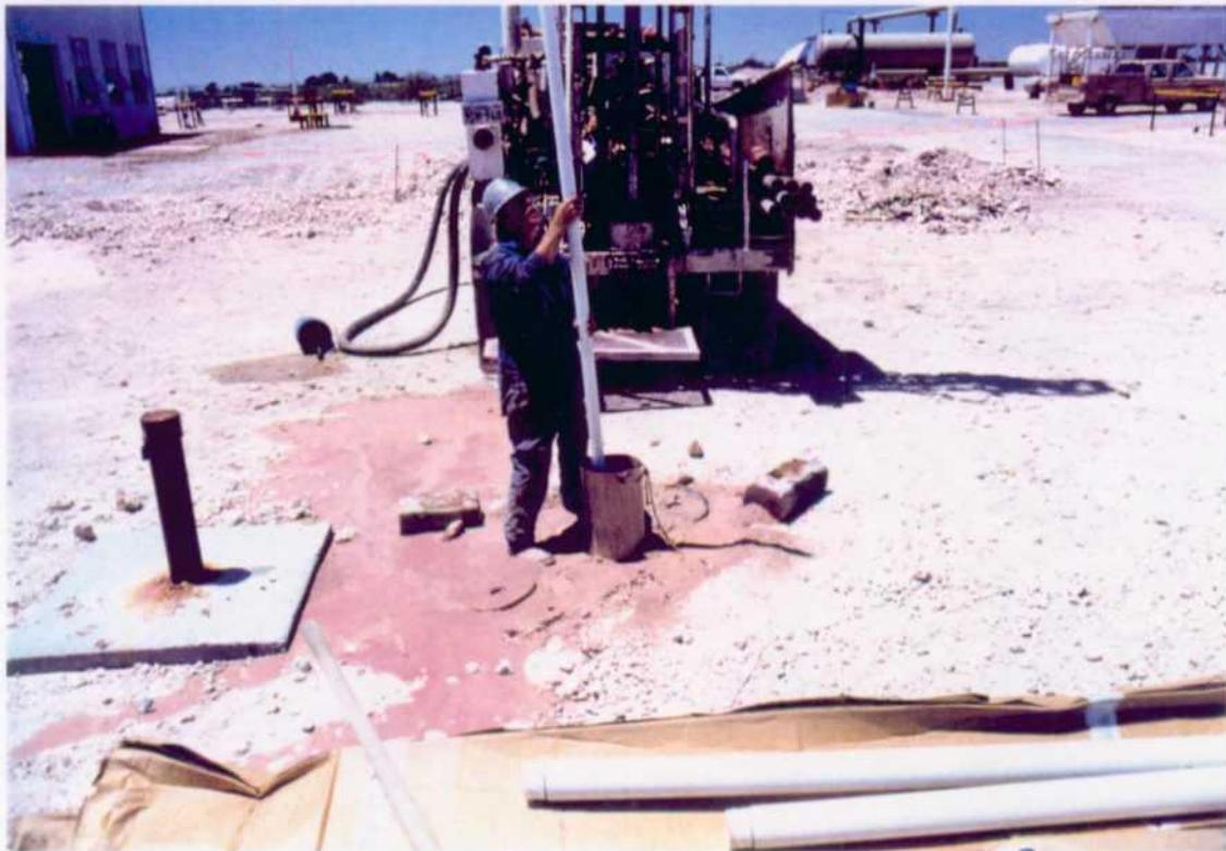
View facing west showing well completion operations for monitoring well MW-1D located adjacent (6 feet north) to monitoring well MW-1.
