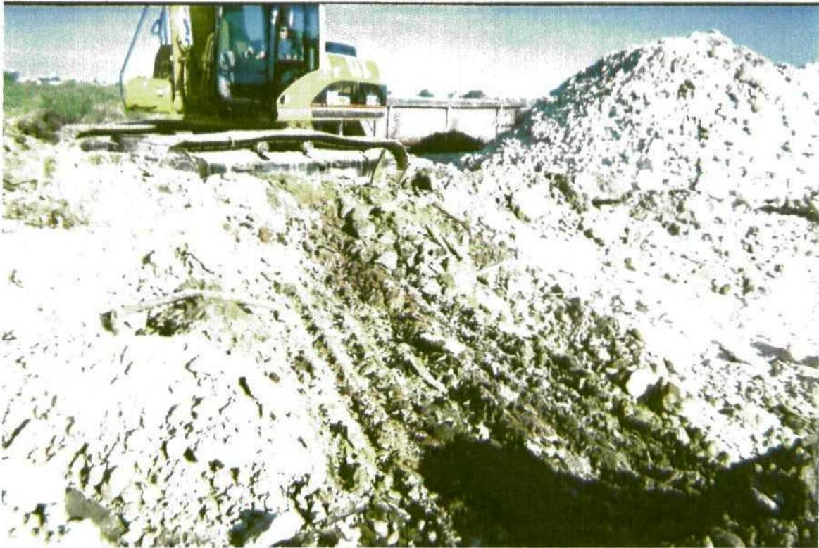
Impacted Area 1 Facing West-Southwest – Impacted soil and old flow line removal
