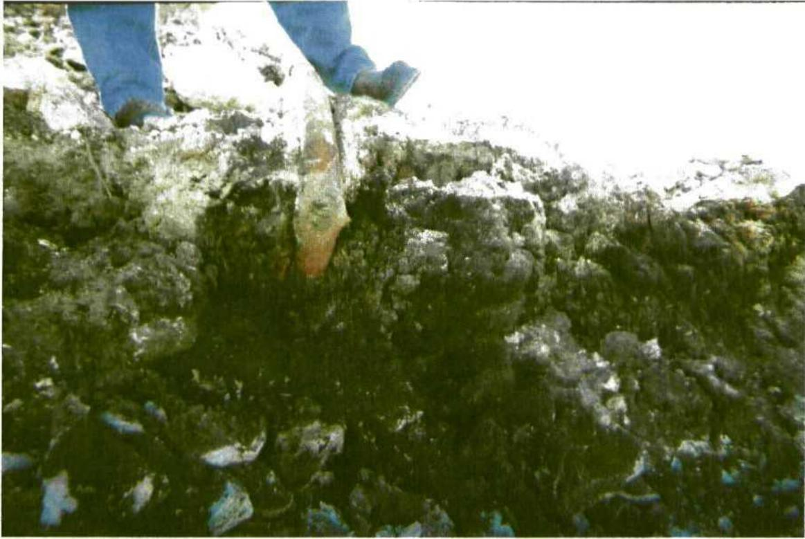
Impact Area 1 – Impacted soil around 2" flow line to be removed
