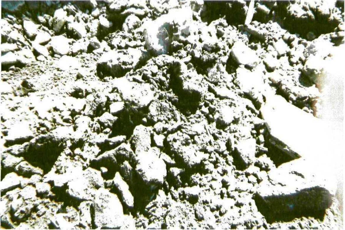
Impact Area 4 – Hydrocarbon contaminated soil excavated from 19 feet below land surface
