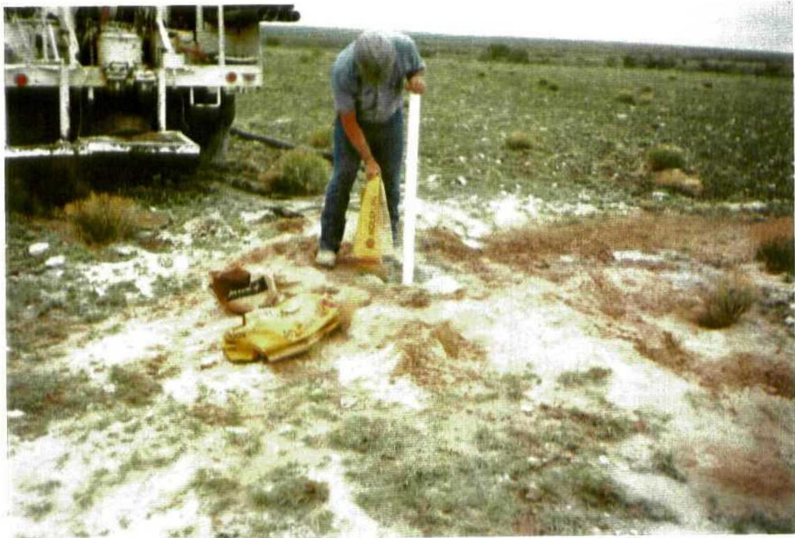
View facing southwest showing placement of bentonite well seal in monitoring well MW-5.
