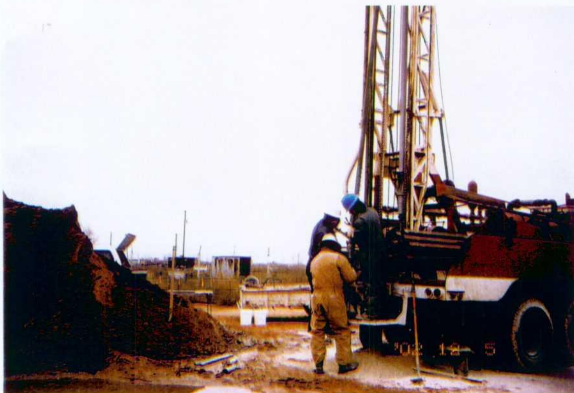
2. View to south. Installation of soil boring BH-13. Stockpiled soil to left in photo.
