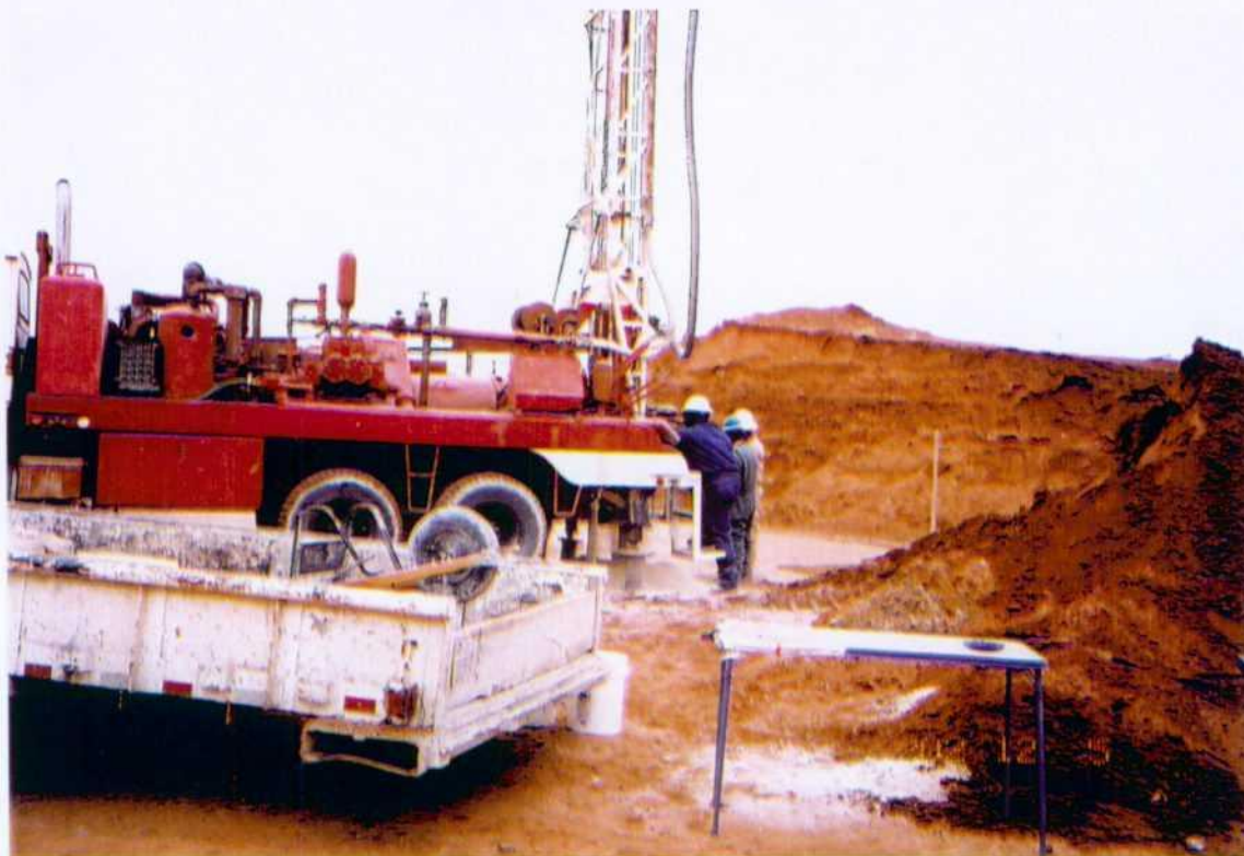
1. View to north. Installation of soil boring BH-13. Stockpiled soil to right in photo.
