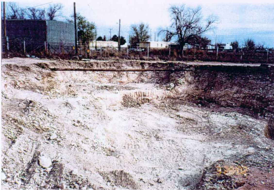
15. Hole #1 and Hole #2 (Looking Southeast)
