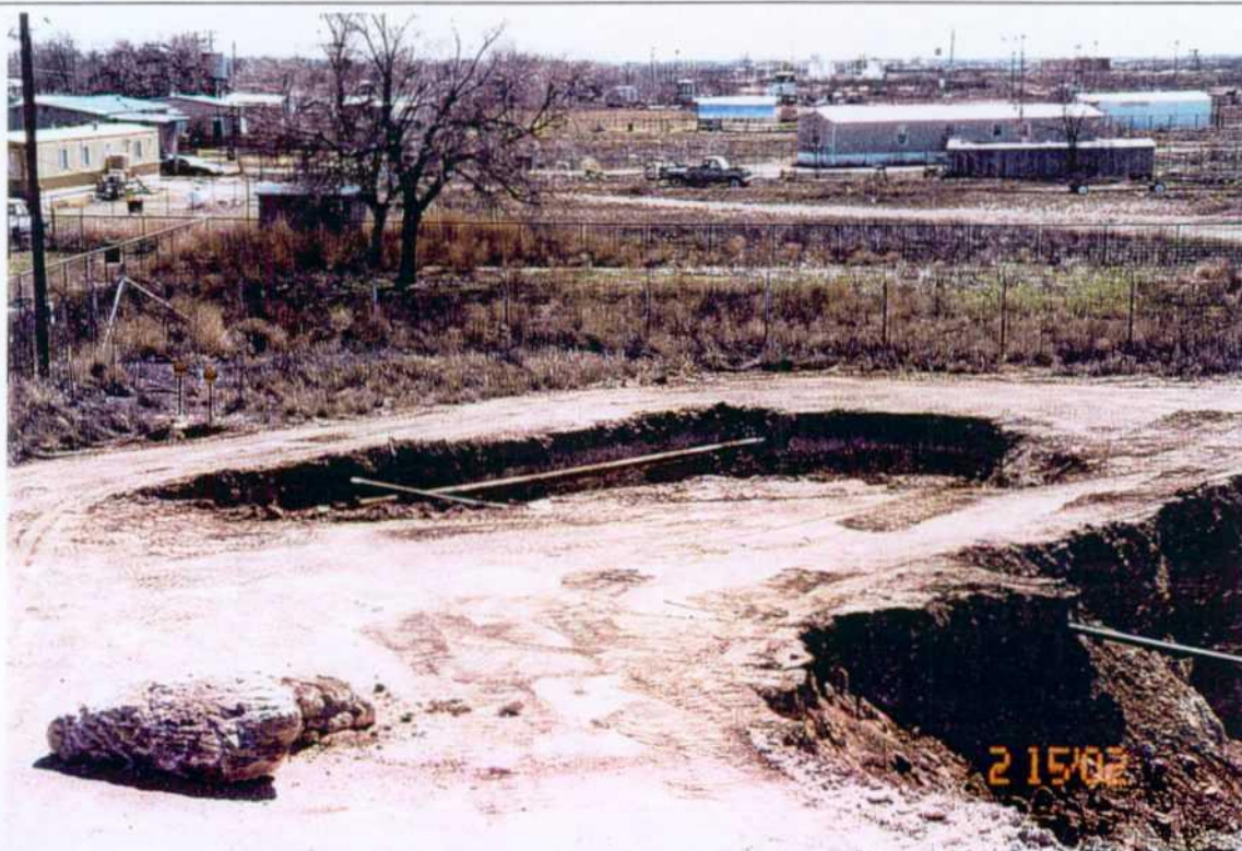
2. Hole #1 (Left) and Hole #2 (Right)
