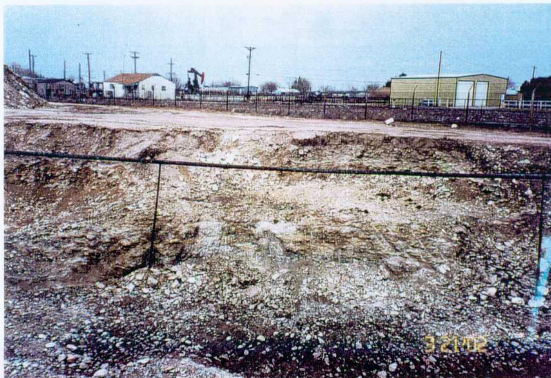
14. Hole #1 and Hole #2 (Looking East)
