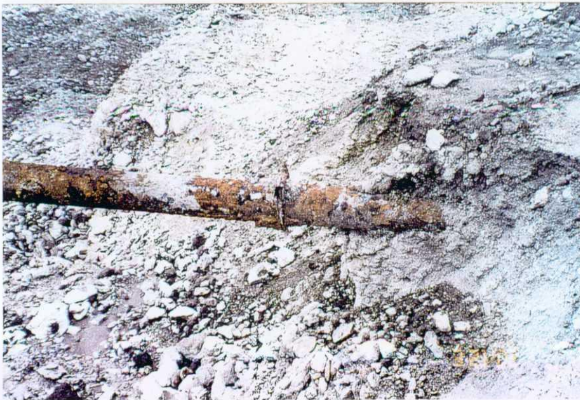
10. Hole #1 (Pipeline Clamp)
