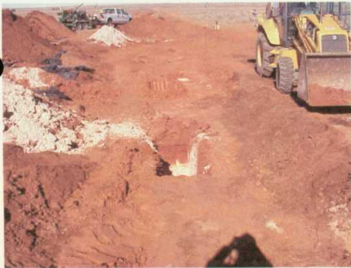
3-7 BH-3 Foreground BH-4 Background
