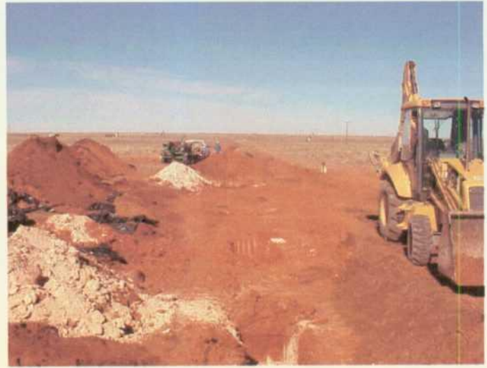
3-8 BH-3 Foreground BH-4 Background
