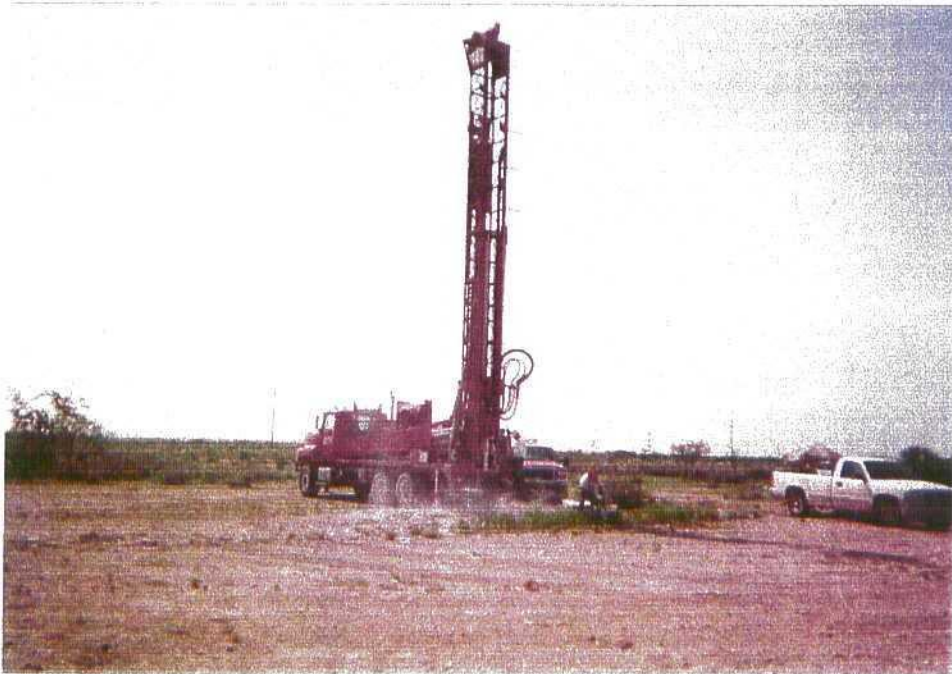
Photo 5: Drilling of soil boring S-6.
