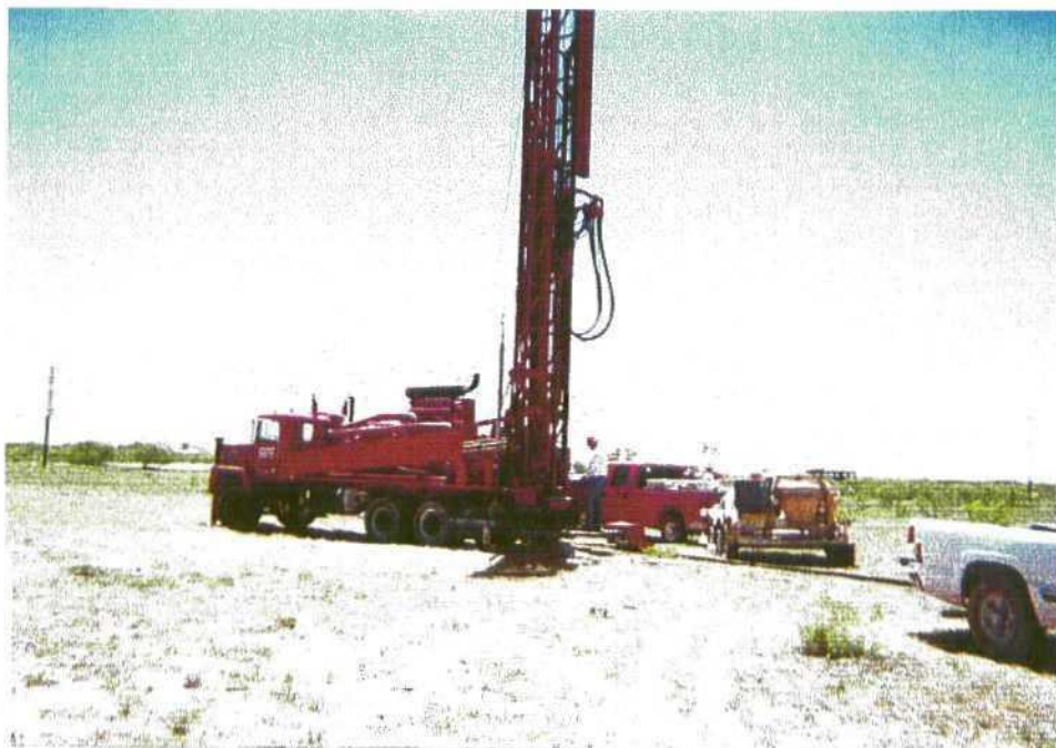
Photo 44: Drilling of monitor well MW-13.
