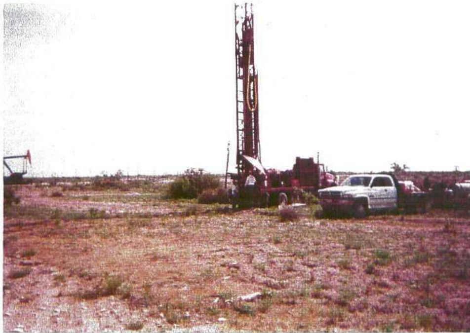
Photo 8: Drilling of soil boring S-9.
