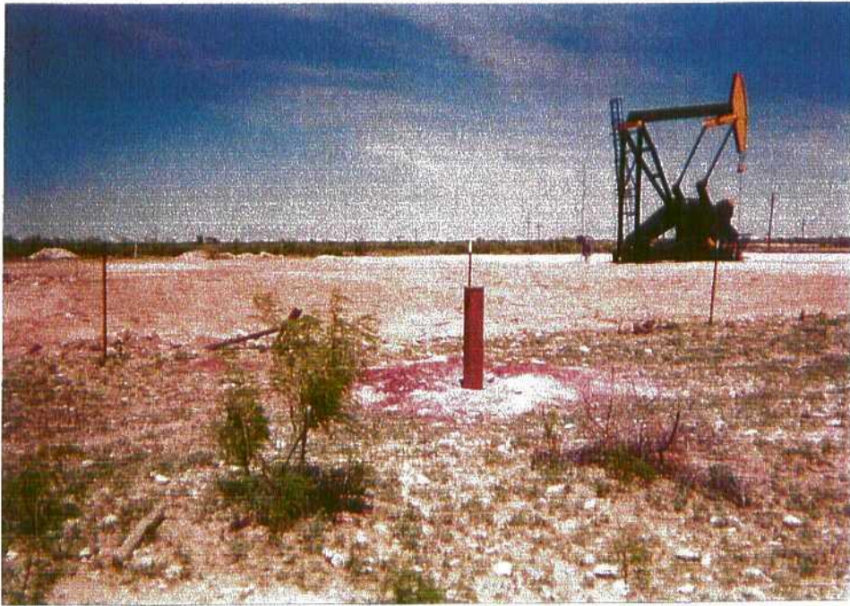
Photo 33: Completed monitor well MW-8.
