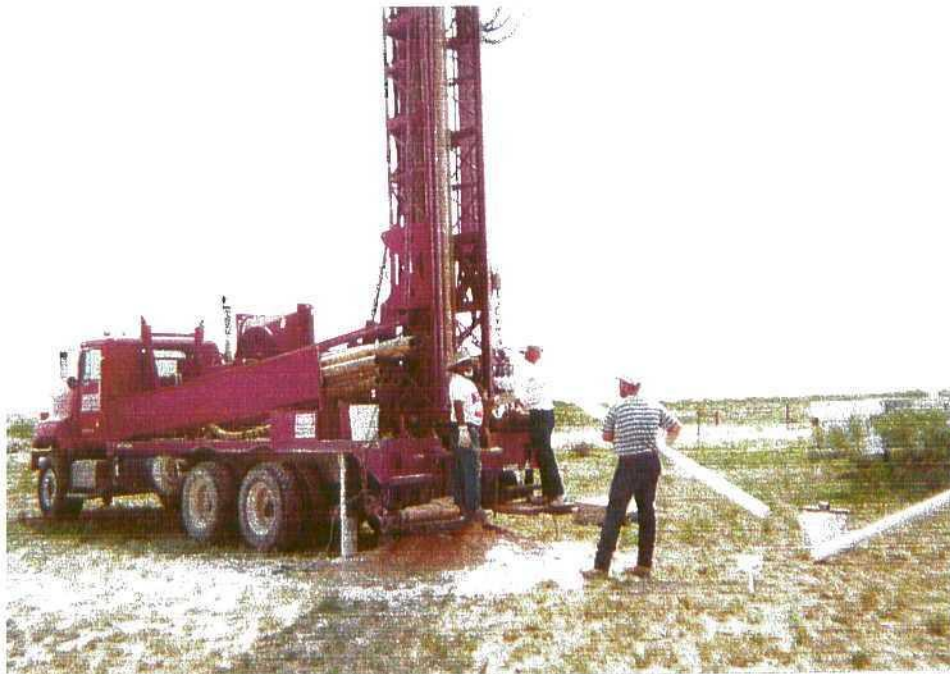
Photo 58: Installation of piping for monitor well MW-17.
