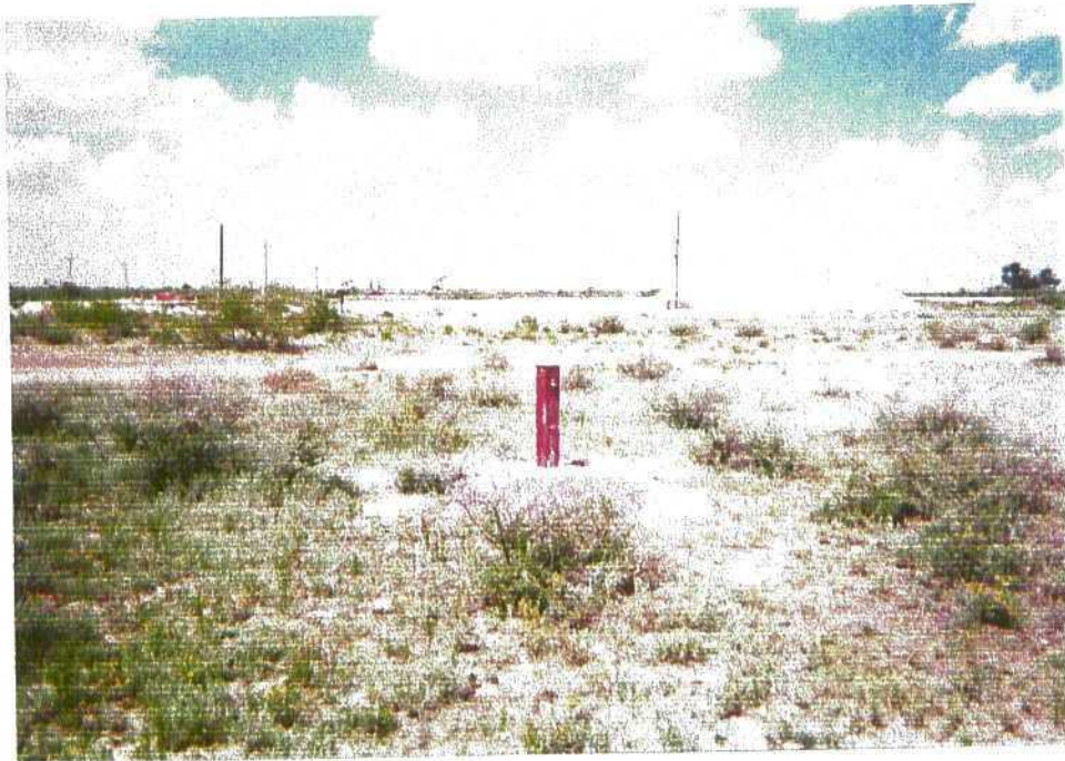
Photo 56: Completed monitor well MW-16.
