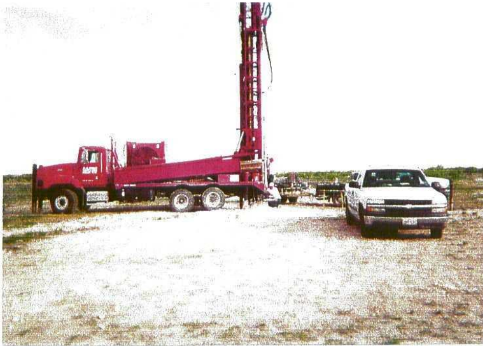
Photo 29: Drilling of monitor well MW-7.
