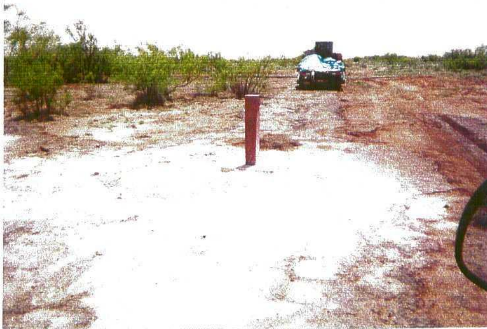
Photo 26: Completed monitor well MW-5.
