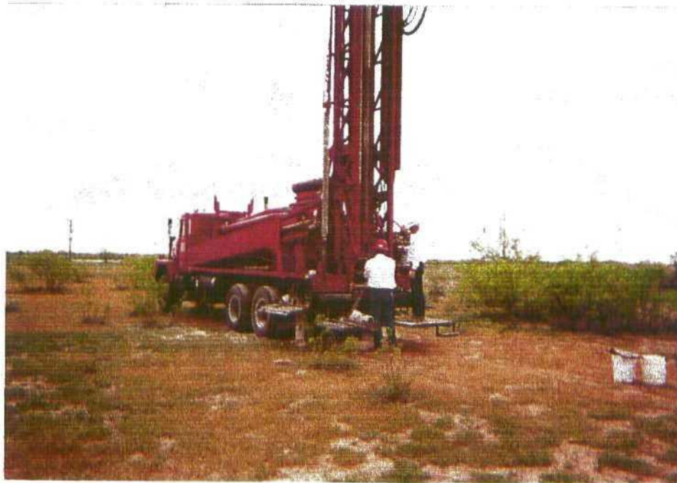
Photo 20: Drilling of monitor well MW-3.
