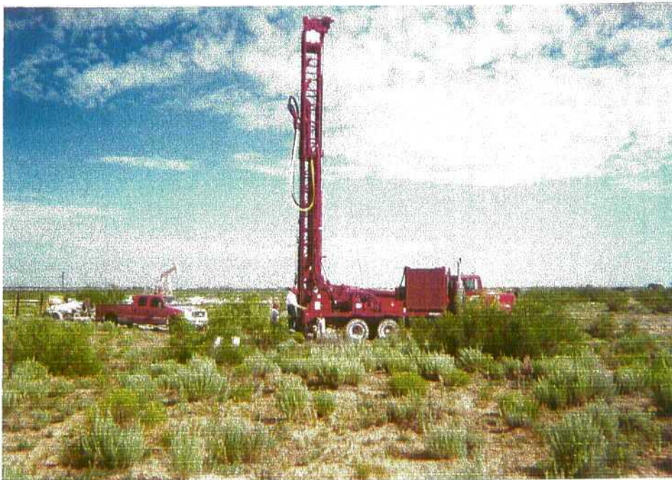
Photo 50: Drilling of monitor well MW-15.
