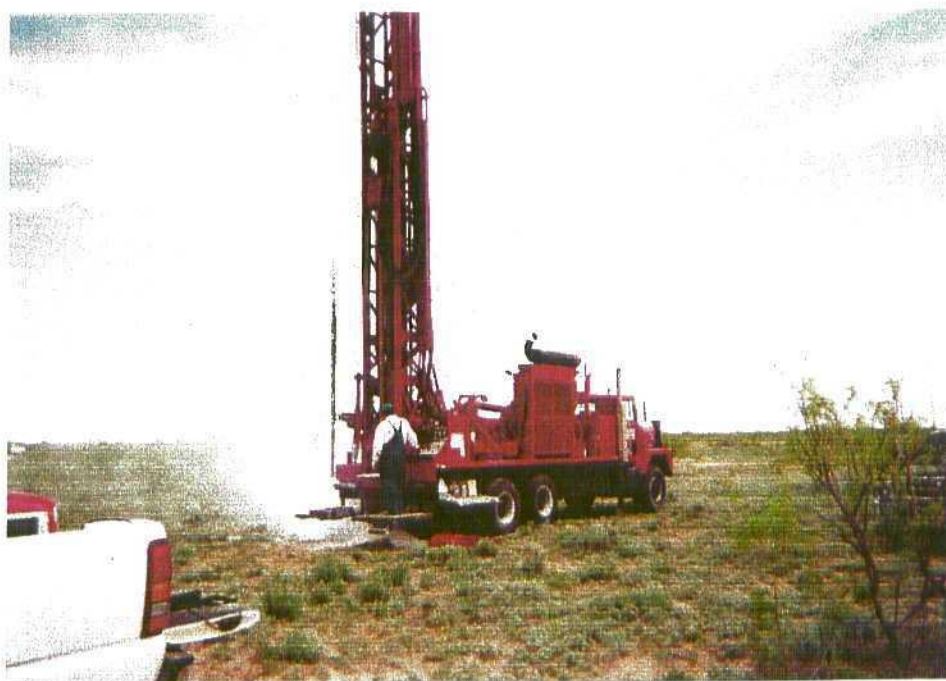
Photo 14: Drilling of monitor well MW-1.
