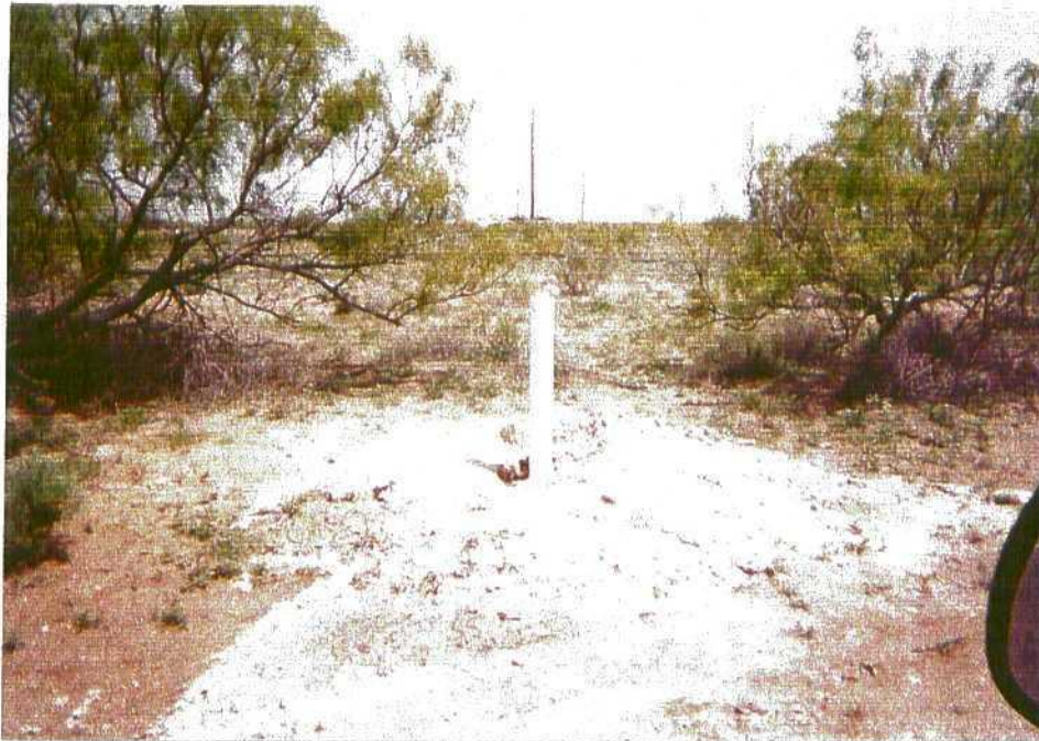
Photo 18: Completed installation of piping in monitor well MW-2.
