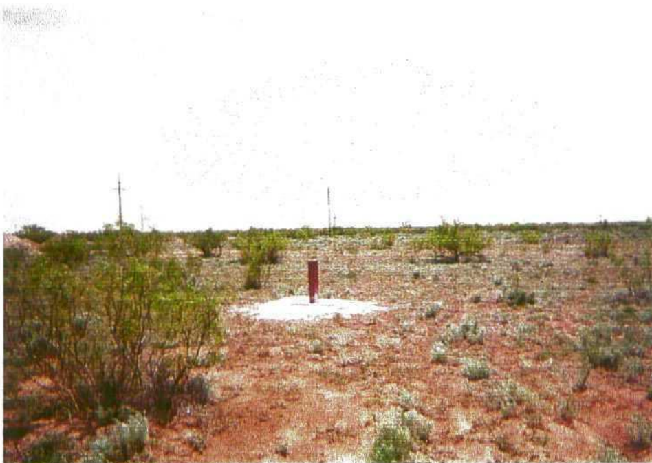
Photo 16: Completed monitor well MW-1.
