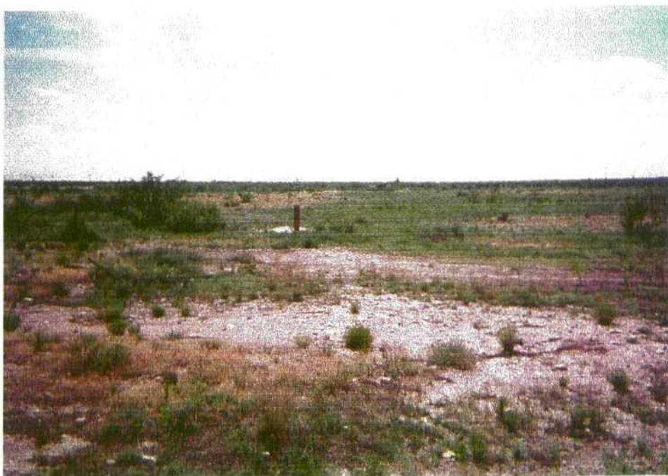
Photo 62: Completed monitor well MW-18.
