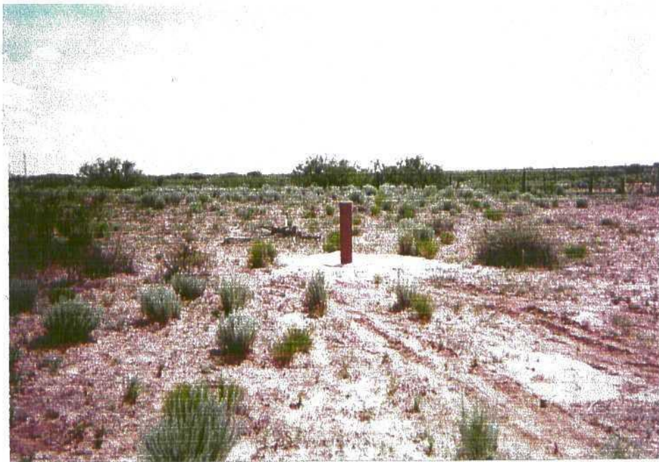
Photo 52: Completed monitor well MW-15.
