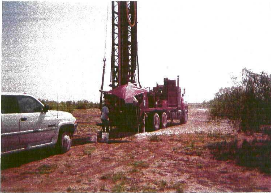
Photo 10: Drilling of soil boring S-11.
