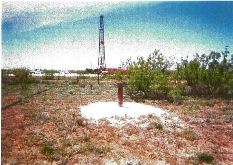
Photo 24: Completed monitor well MW-4.
