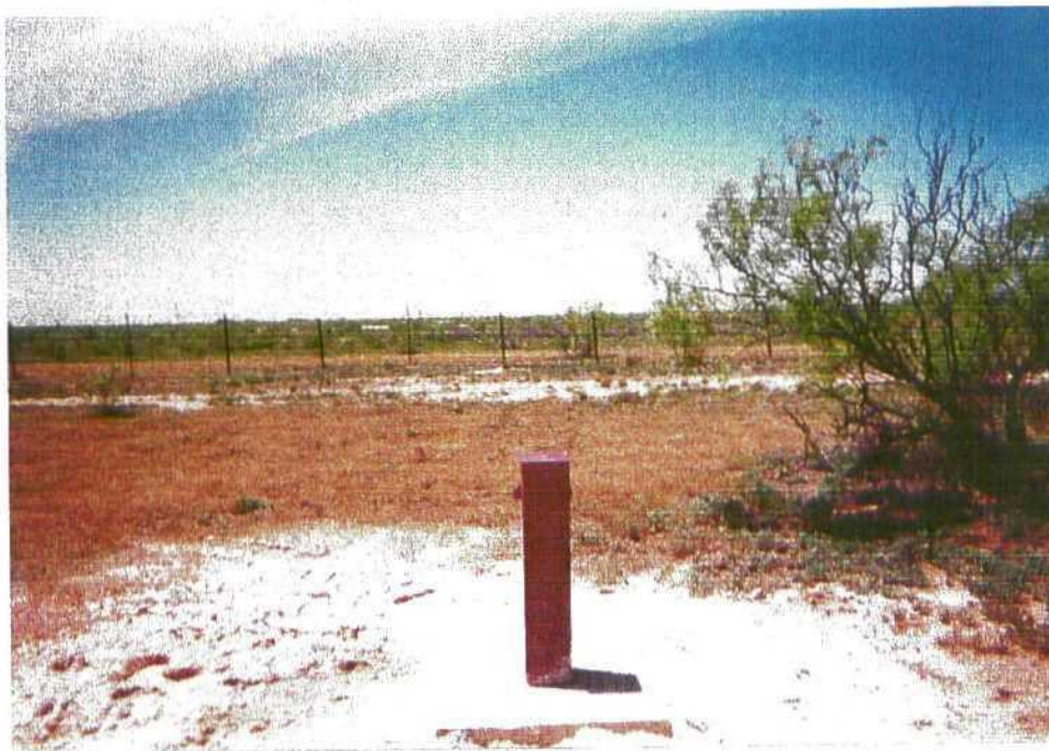
Photo 27: Drilling of monitor well MW-6.
