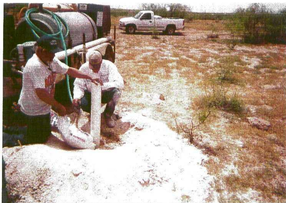
Photo 37: Drilling of monitor well MW-10.
