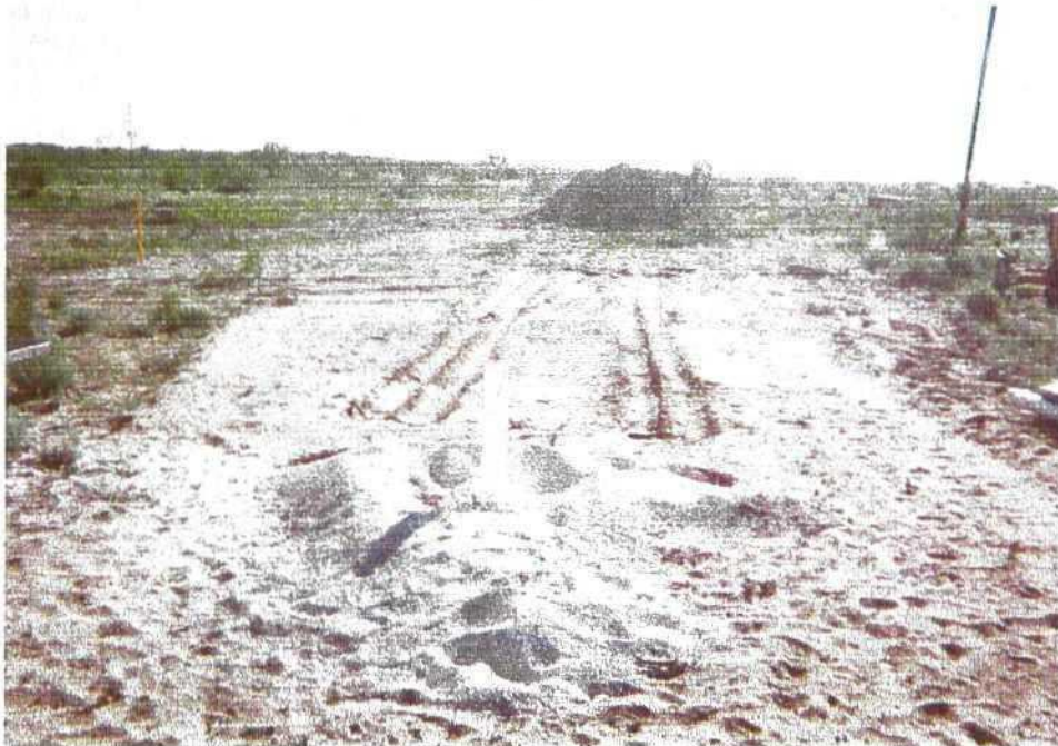
Photo 48: Installed piping for monitor well MW-14.
