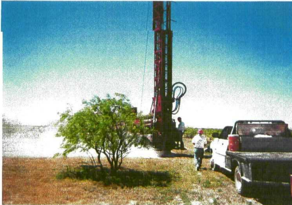
Photo 39: Completed monitor well MW-10.
