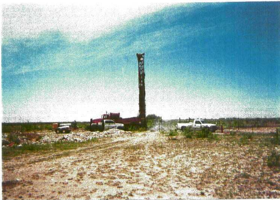
Photo 2: Drilling of soil boring S-4.
