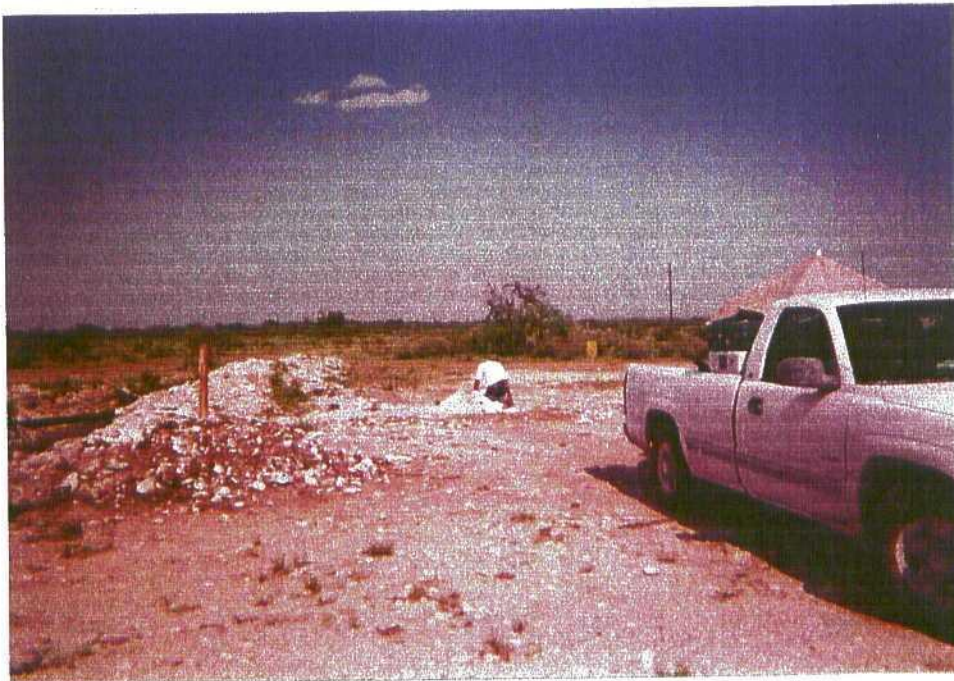
Photo 4: Grouting of soil boring S-5.
