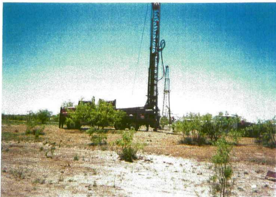
Photo 42: Drilling of monitor well MW-12.
