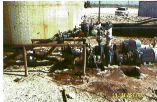
Picture # 1435- Saga SWD tanks and centrifugal pumps inside of berm. Picture taken from west side looking SE. At time of site visit these pumps were leaking water onto the ground surface.
