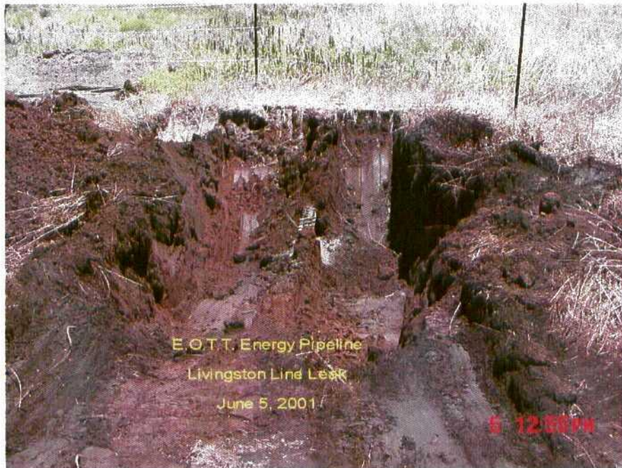
Photograph #3 – Looking westerly at initial excavation.
