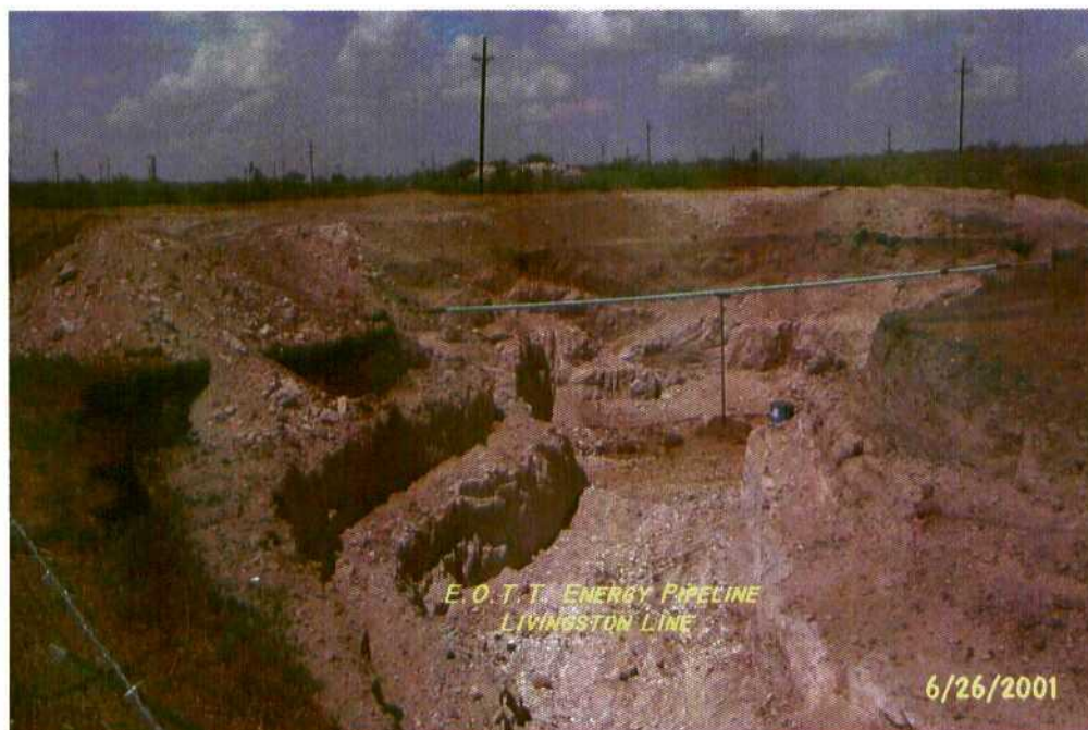
Photograph #3 – Looking northerly at excavation.
