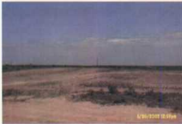
Site contoured and completed.
