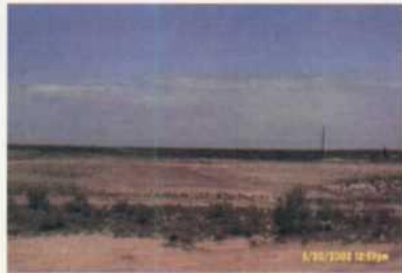
Site contoured and completed.
