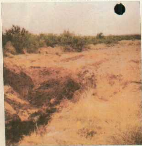
#2 Leak TNM P/L 10-3-96
