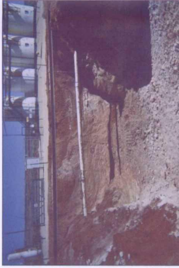
Looking North: Final Excavation 30 x 18 x 12 ft deep
