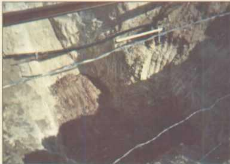
Clay Barrier @ 16' bgs
