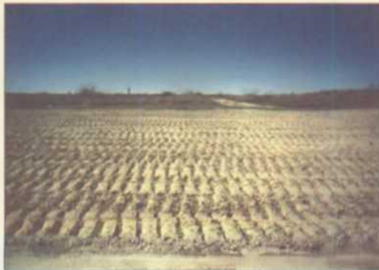
Remediated & Backfilled (looking west)
