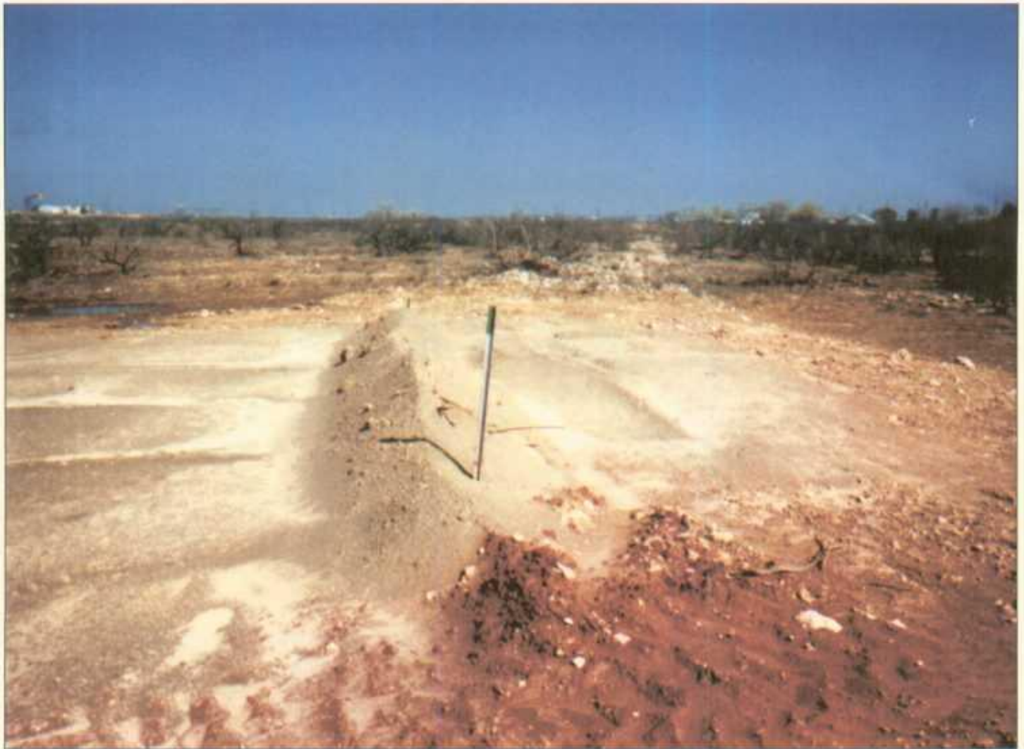
After Remediation (No Junction Box)
