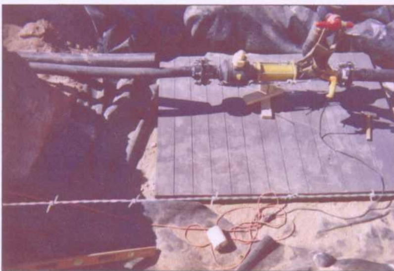
Floor Construction of New Plastic Box with Poly Liner (130 ft East)
