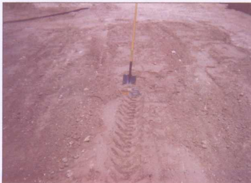
Old Jct. Site: Backfilled with ID Plate
