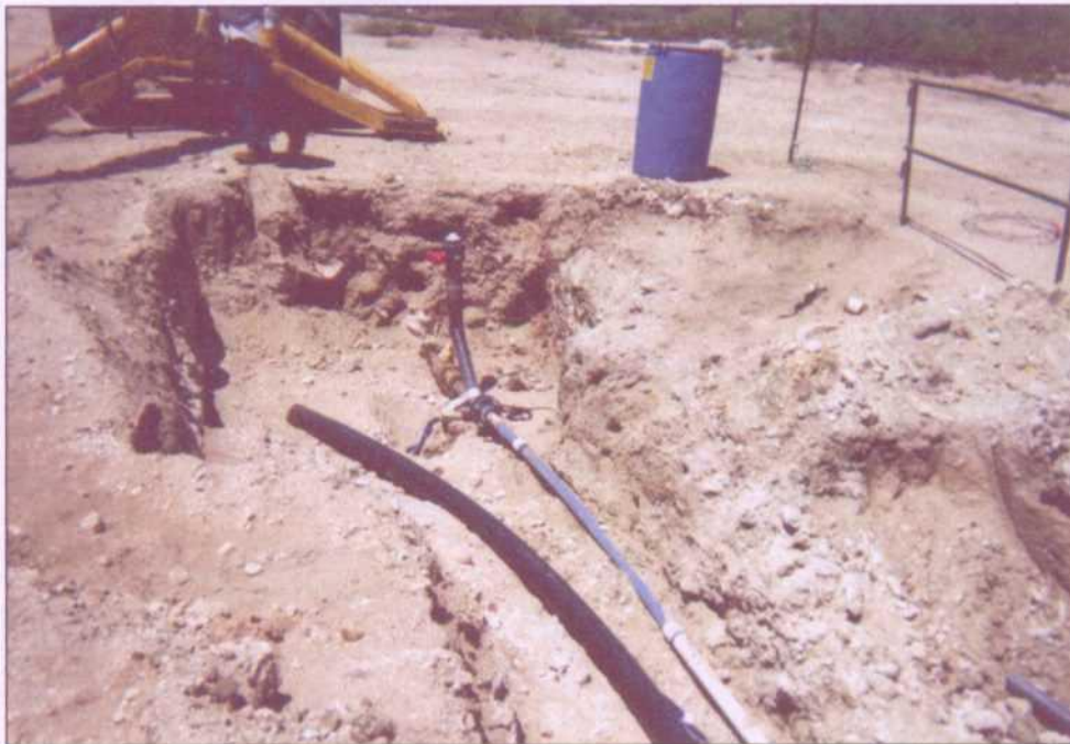
After NORM Removal; Before Impact Delineation & Excavation
