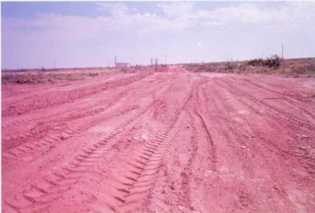
Complete & Backfilled (no junction box required)
