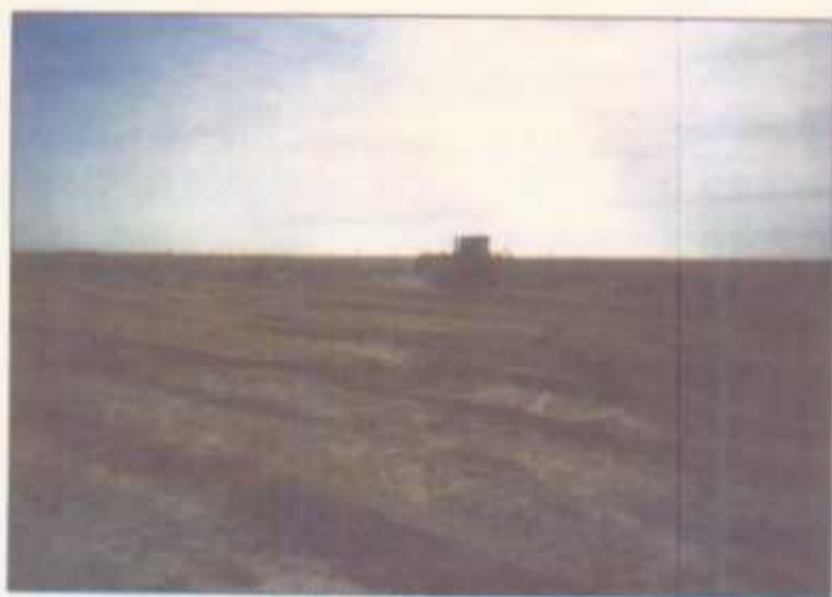
Backfilled (looking south)
