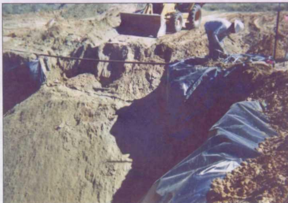
Backfilling Into Liner
