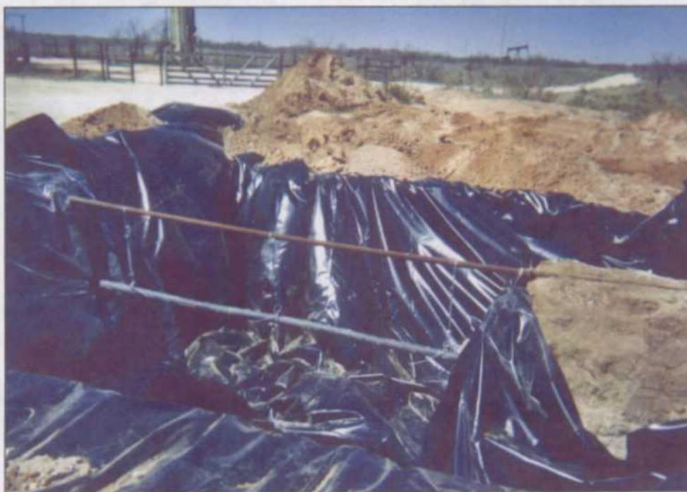
Poly Liner Installed
