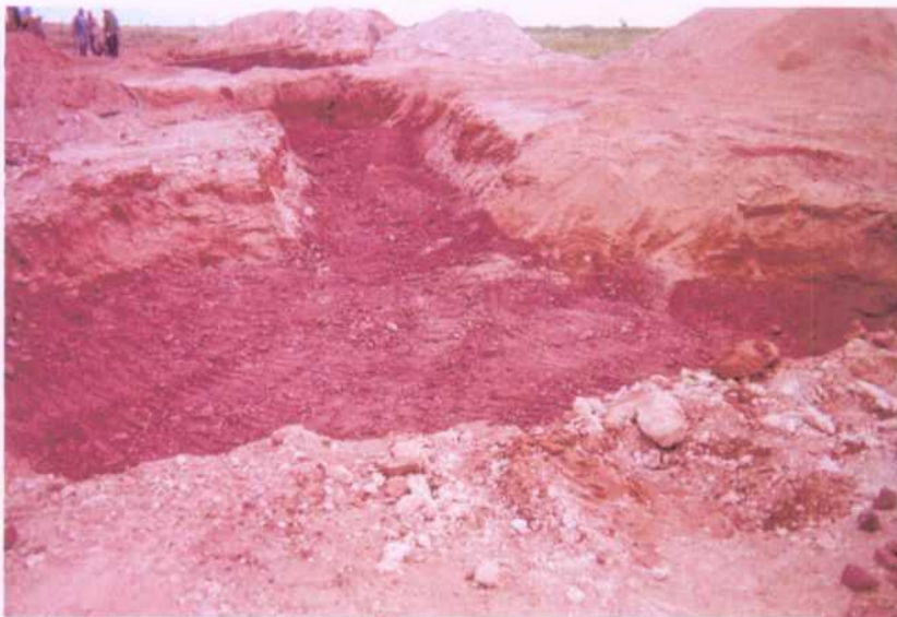
Clay liner connected to O-17
