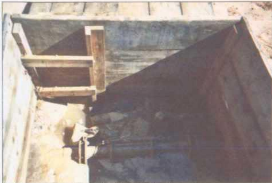
Old Junction Box Before Excavation
