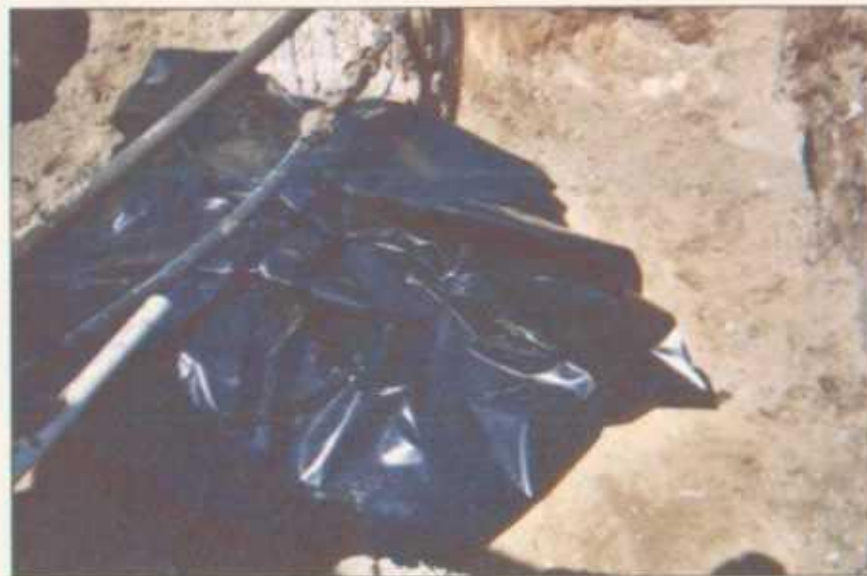
Installing Poly Liner
