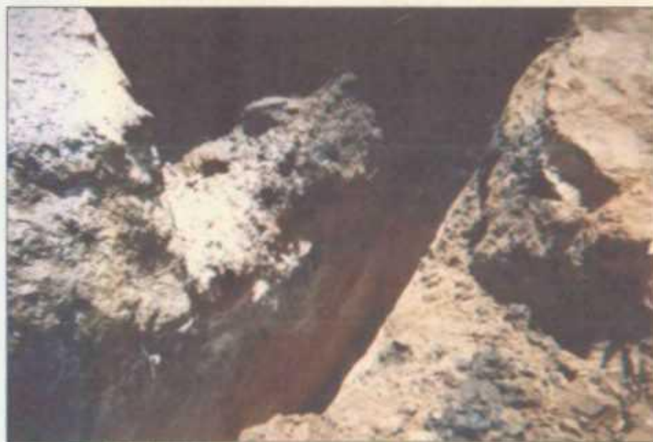
Vertical Excavation trench 7/31/2003
