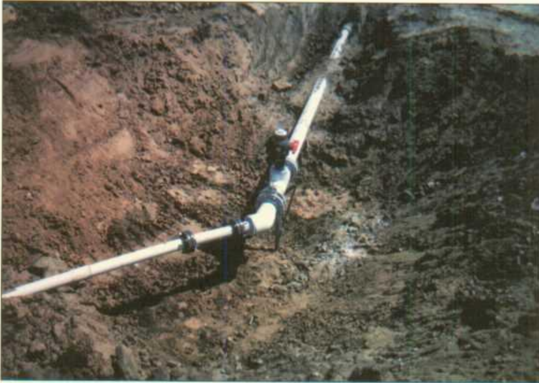
Remediation (with new plumbing)
