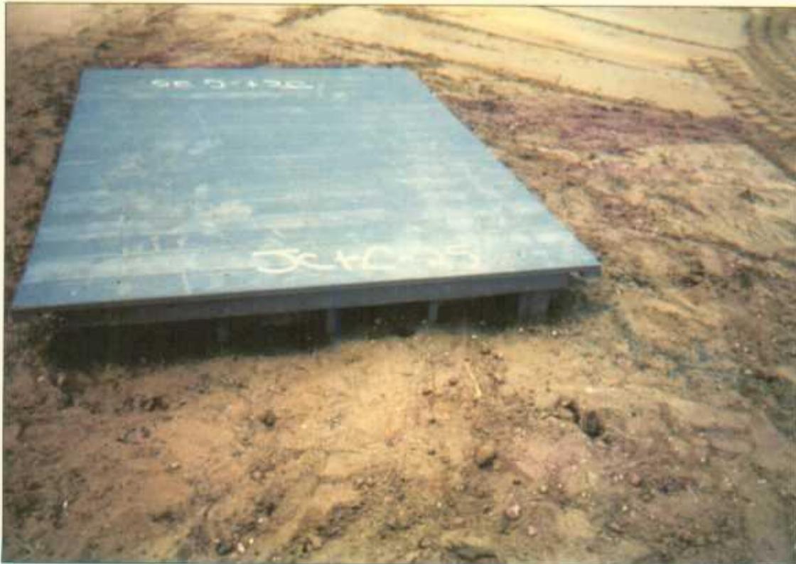
Completed New Junction Box
